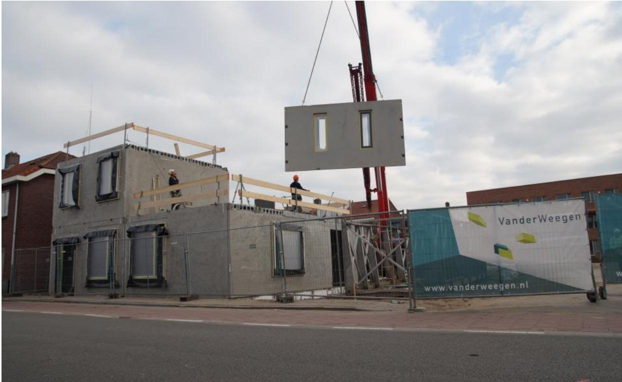
Figure 7.26 A pre-fab concrete building under construction.
