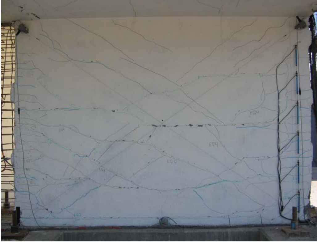
Figure 99 UCSD 7-Story Shake Table Test – Crack pattern after full protocol – Level 1
