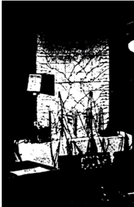
Figure 89 RW2-Crack pattern upon completion of testing (Thomsen and Wallace, 1995)
