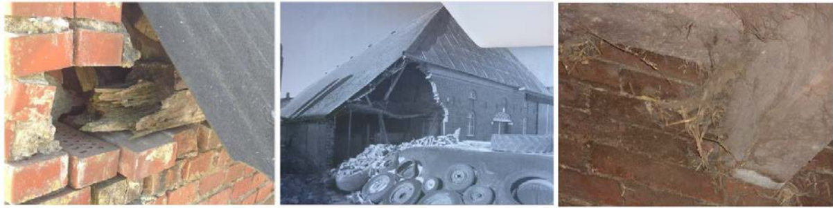
Figure 6.2: Timber URM Old Barn – Damage associated with decay over time
