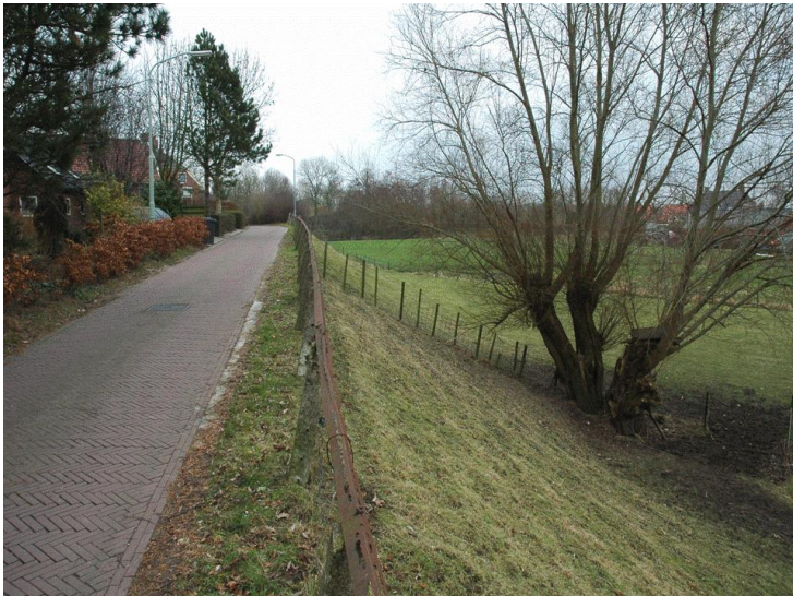
Figure 3.16: fence posts show that soil creep is a current process on the steep terp side of Wirdum after quarrying (photo: J. Meijering, Province of Groningen)
