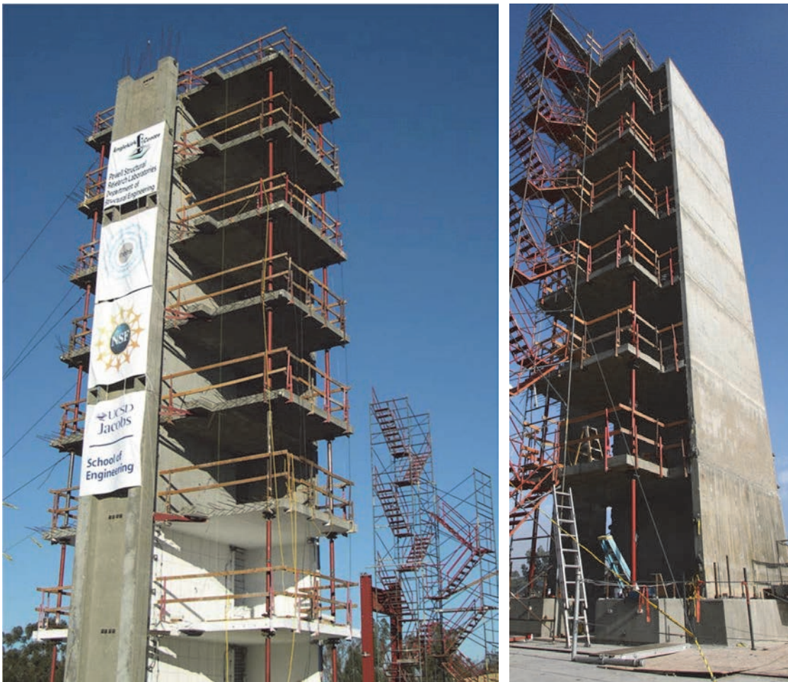
Figure 44: Full-scale seven-storey RC shear wall building tested at the NEES Large High-Performance Outdoor Shake Table at UCSD's Englekirk Structural Engineering Center
