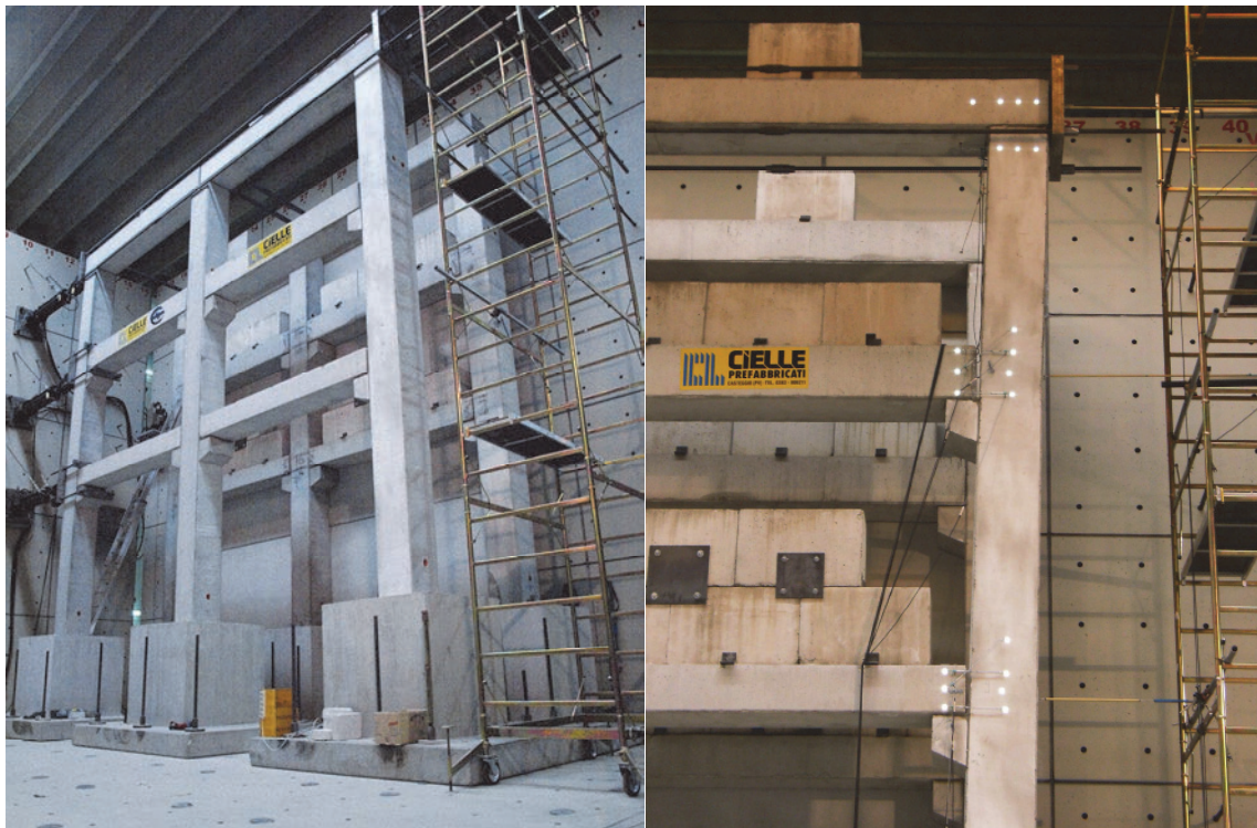
Figure 11: Three-dimensional precast reference building tested at the EUCENTRE of Pavia (Italy)
