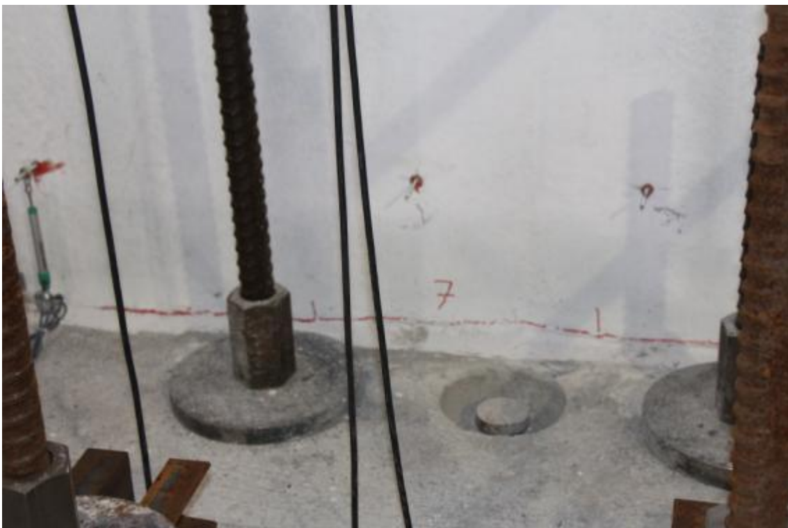
Figure 207. Evolution of crack pattern at the base of the transversal walls – North side of the specimen.
