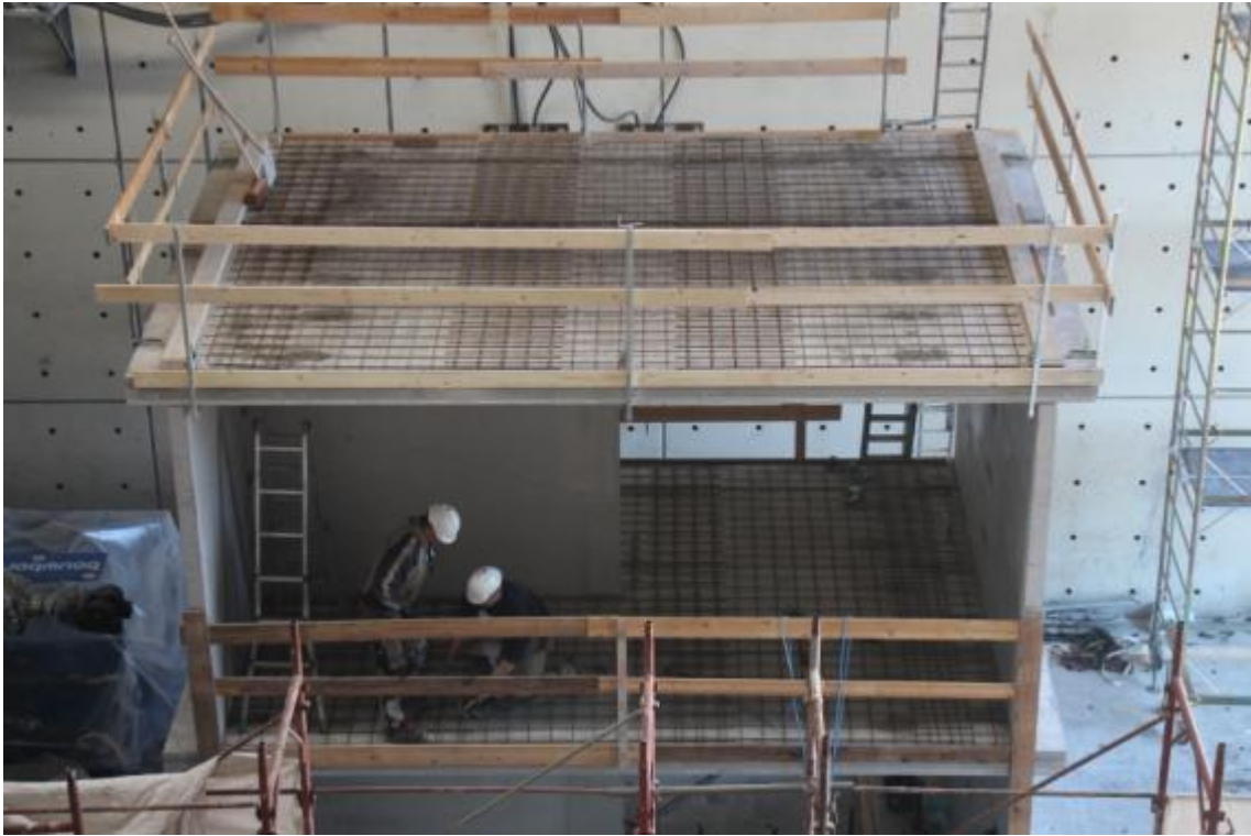
Figure 52. Steel reinforcement of concrete slab topping – first floor.
