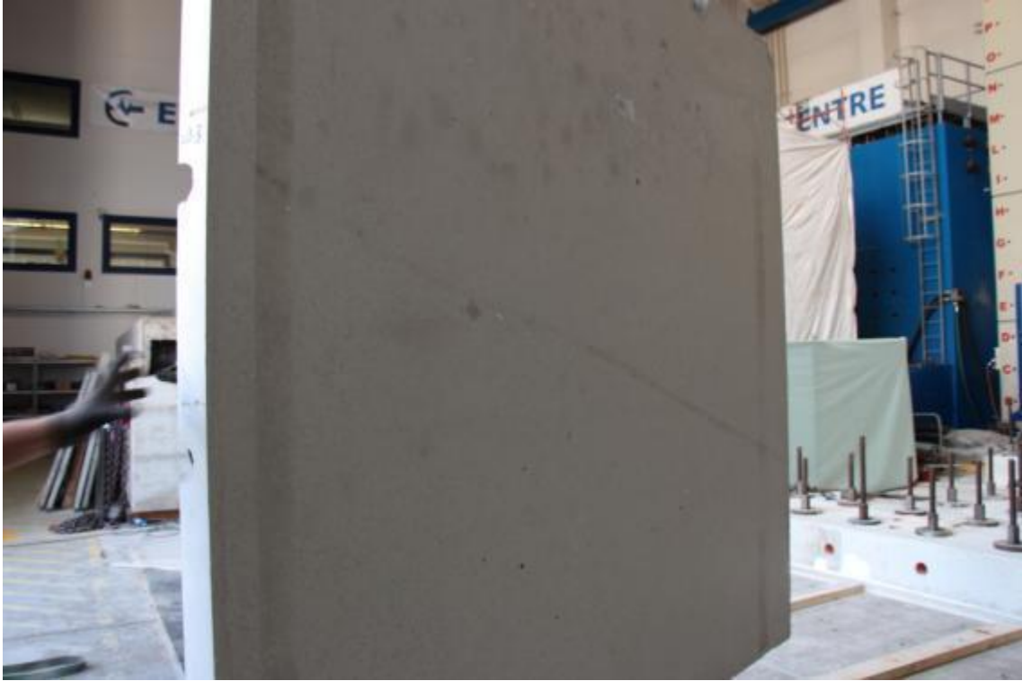
Figure 20. Uplift and transportation of precast wall-elements by means of cranes – detail 3.
