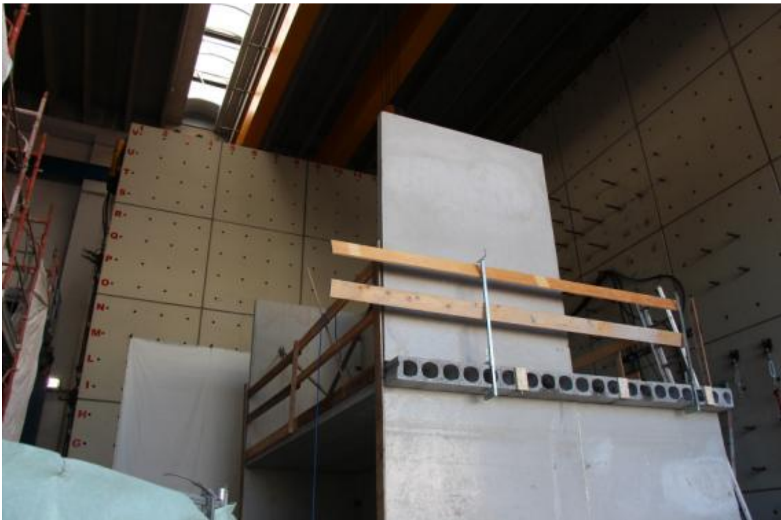
Figure 39. Assemblage of precast wall-elements of the second storey.
