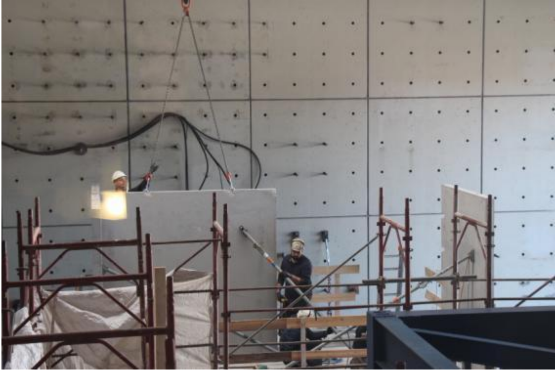
Figure 42. Panel lifting and fixing of the stability wall panel.
