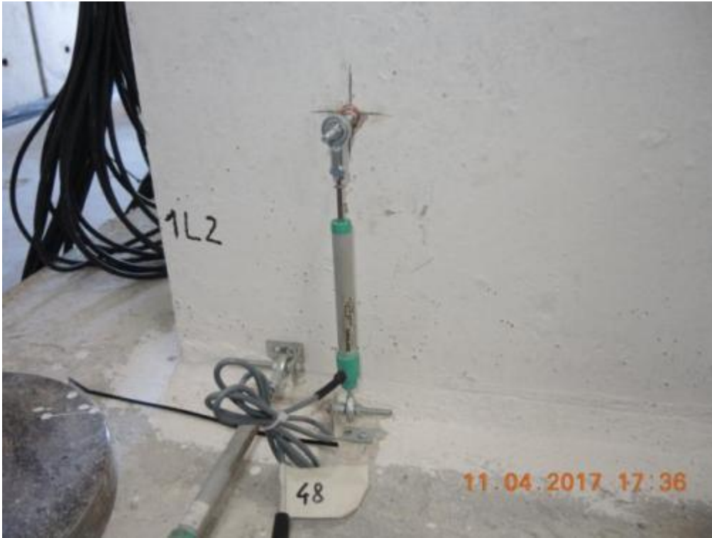
Figure 119. Detail of the instrumentation installed at the base of a lateral wall – Opposite panel.
