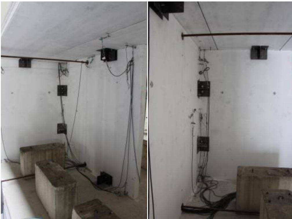
Figure 219. EUC-BUILD4 “retrofitted” specimen – Detail of the second-storey walls, South side.
