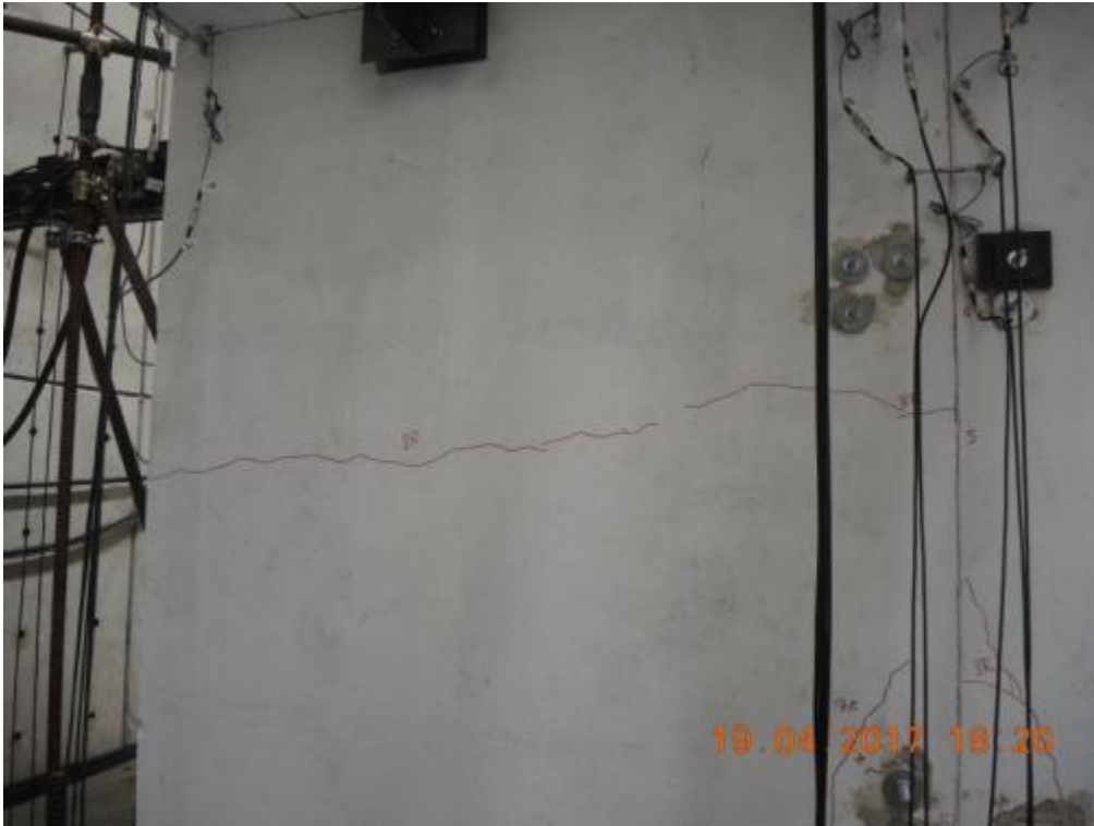
Figure 295. Front view of the full-depth/full-width/mid-height horizontal crack in lateral wall W1L2.
