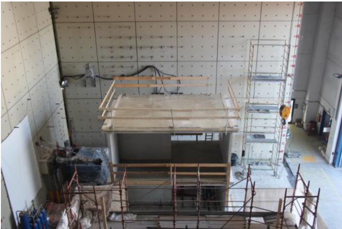
Figure 63. Overall view of EUC-BUILD4 specimen after levelling and finishing – top view.
