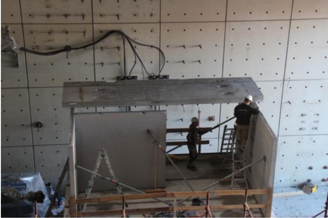
Figure 44. Installation of hollow core slabs of the second storey – top view.
