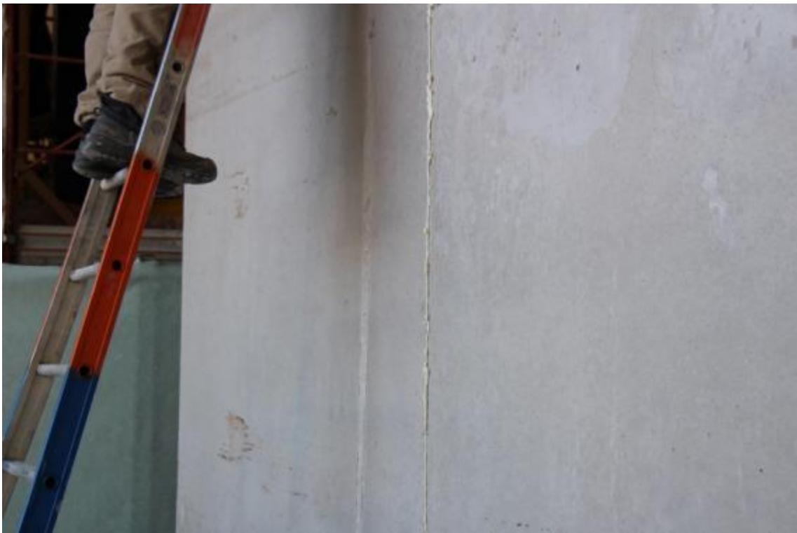
Figure 27. Detail of filling in contiguous precast panels – lateral wall.
