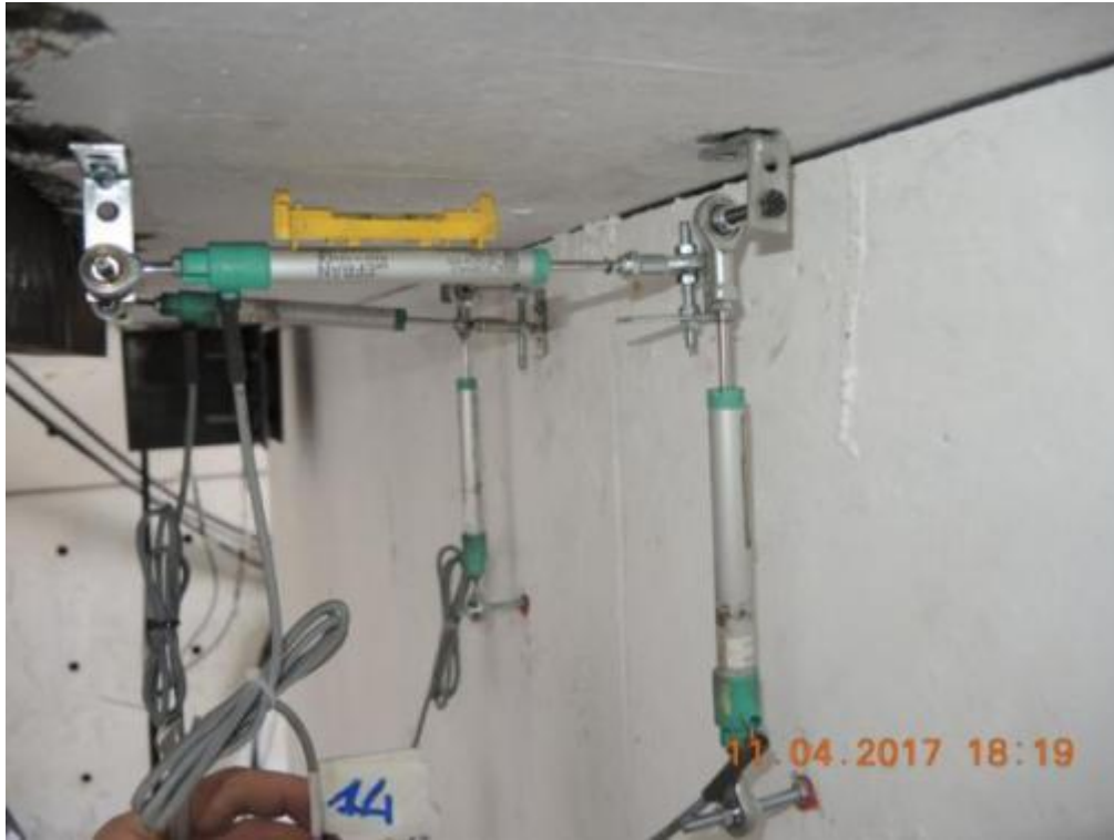
Figure 105. Instrumentation mounted onto the lateral walls – panel-to-panel connection.
