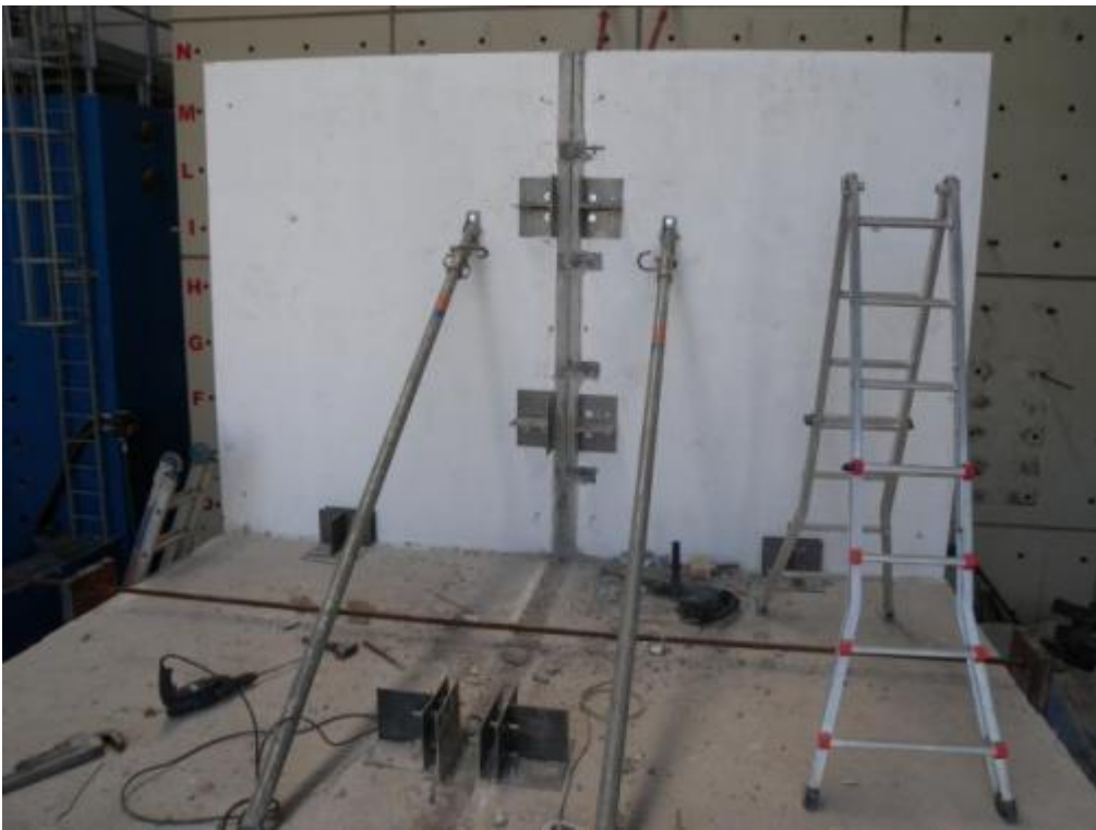
Figure 336. Transversal walls before dismantling – Second storey, South side.
