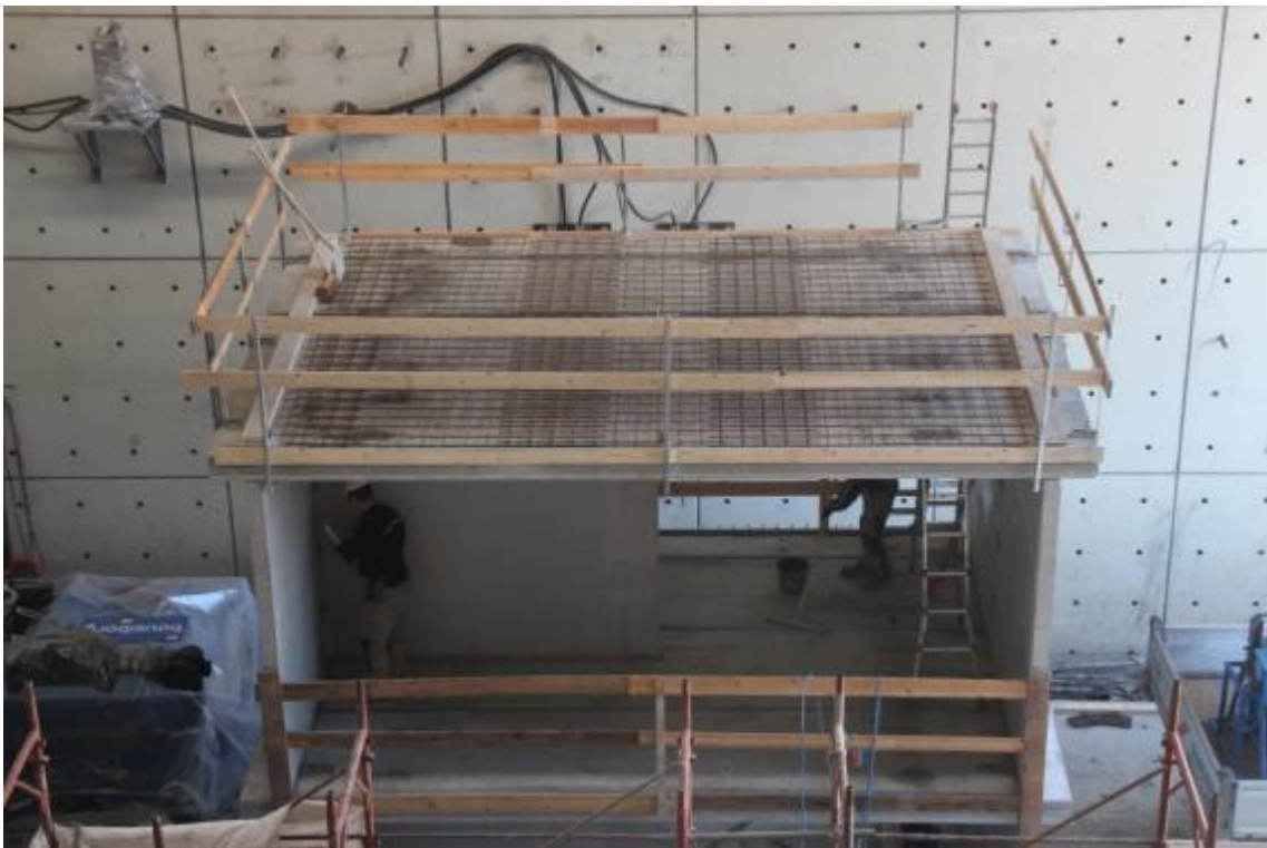
Figure 49. Arrangement of steel reinforcement before casting of concrete topping – second floor.
