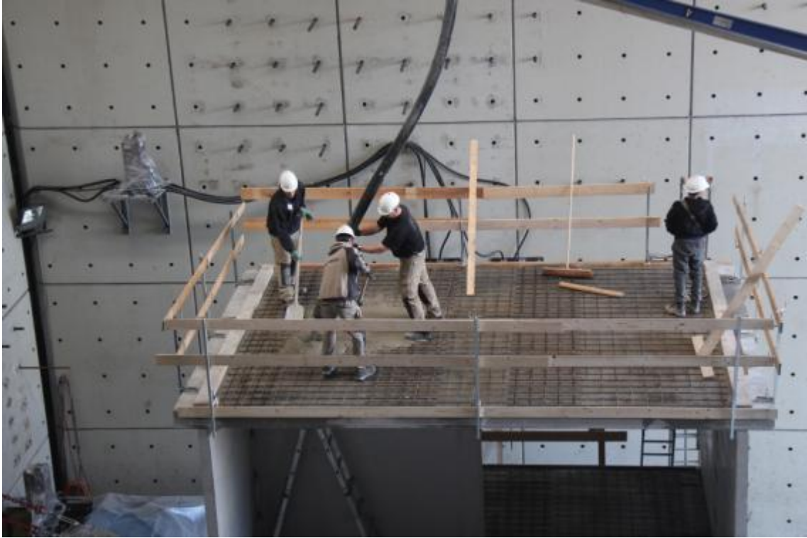
Figure 54. Casting of concrete slab topping – second storey, detail 2.
