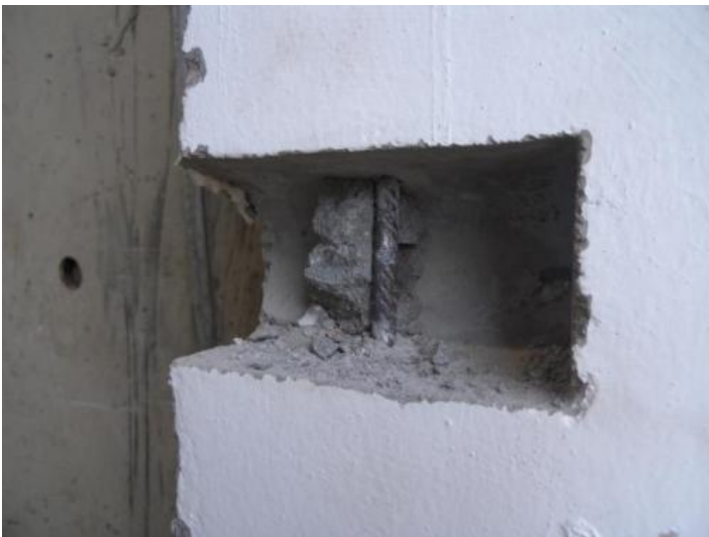
Figure 334. Detail of panel reinforcement in one of the second-storey transversal walls.
