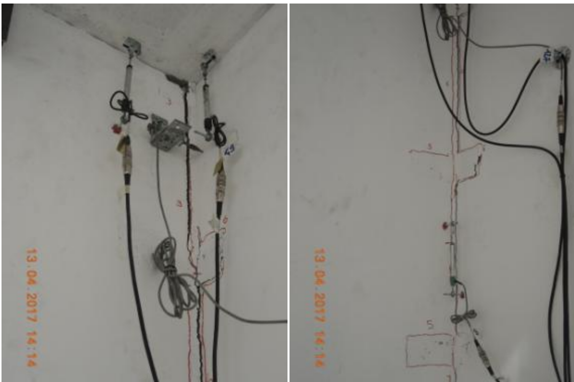
Figure 191. Extensive damage of the top three-way joint – detail of niches and grout, lateral walls.
