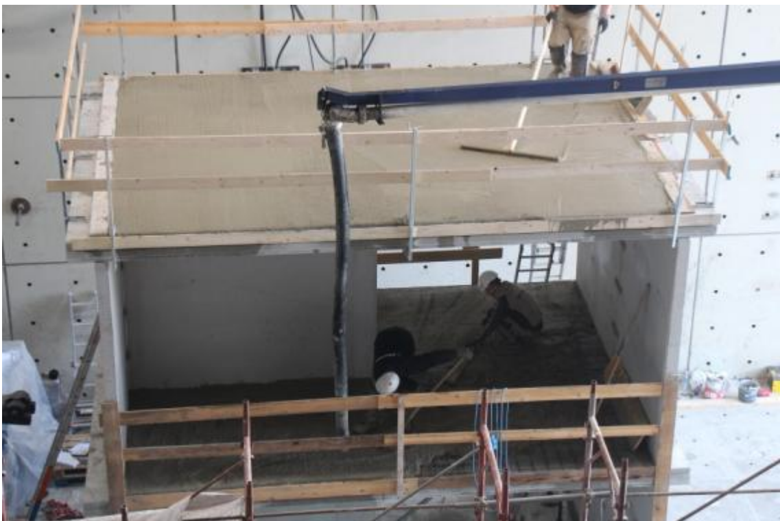
Figure 59. Casting of concrete slab topping – first storey, detail 2.
