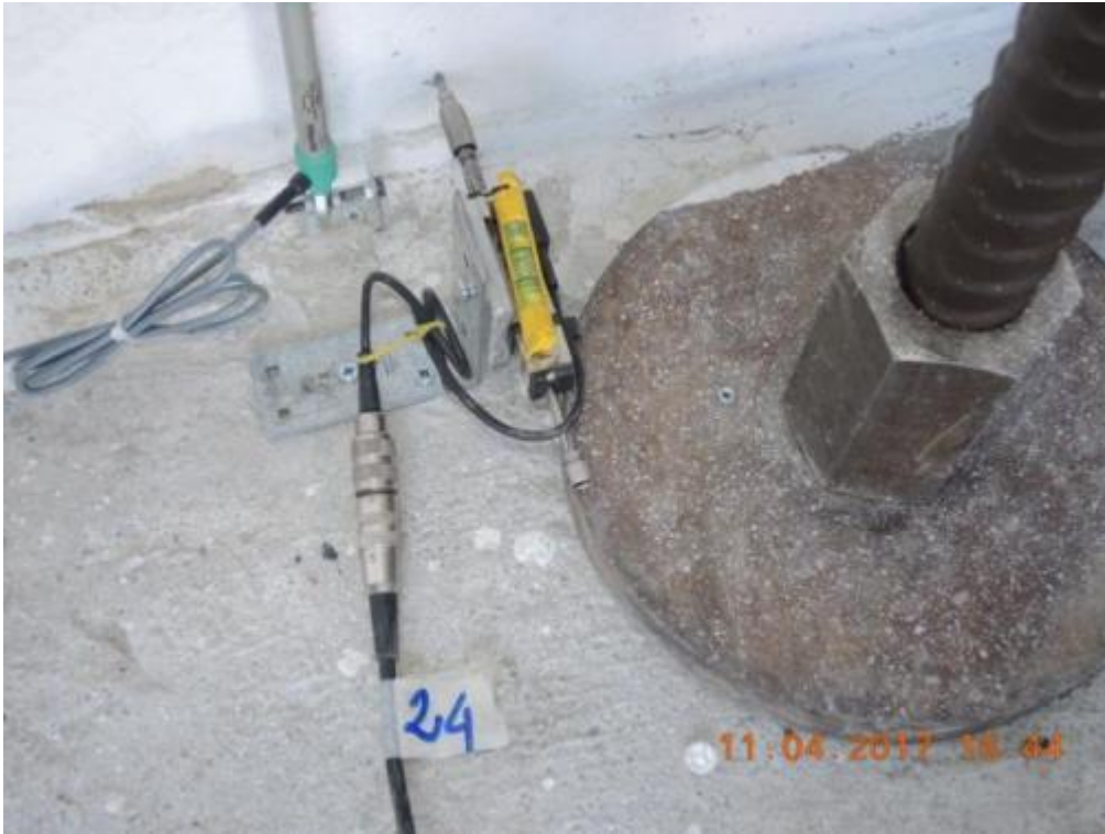
Figure 73. Detail of bars post-tensioned to the concrete foundation.
