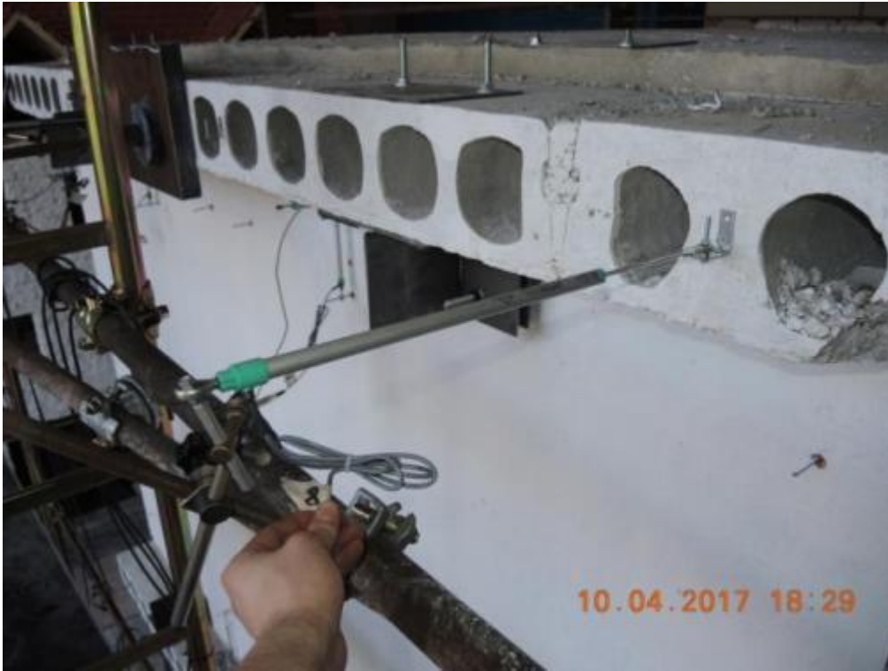
Figure 99. Detail of the instrumentation for global displacement of the second storey – Lateral slab panel.
