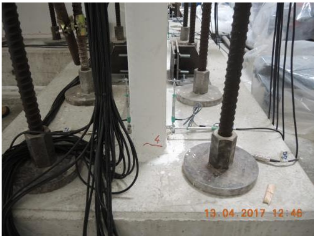
Figure 179. Formation of a new crack at the base of transversal walls – South side of the specimen.
