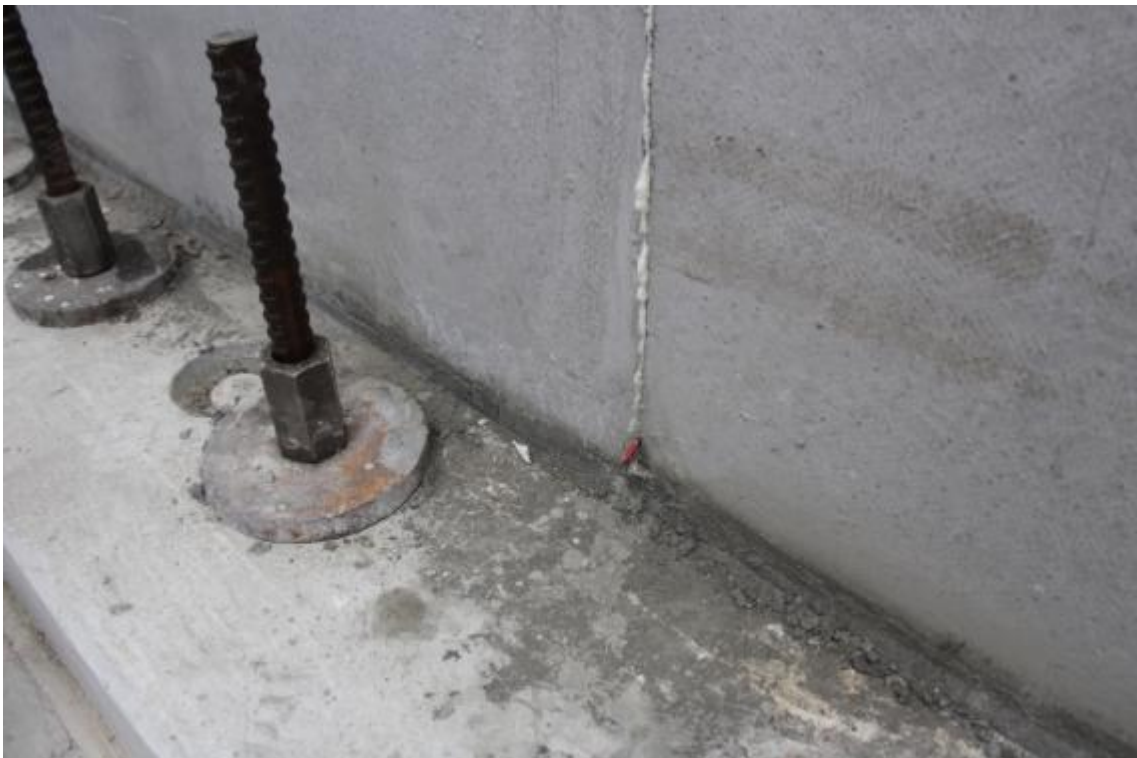
Figure 37. Detail of base mortar joint after dismantling of plywood beams.
