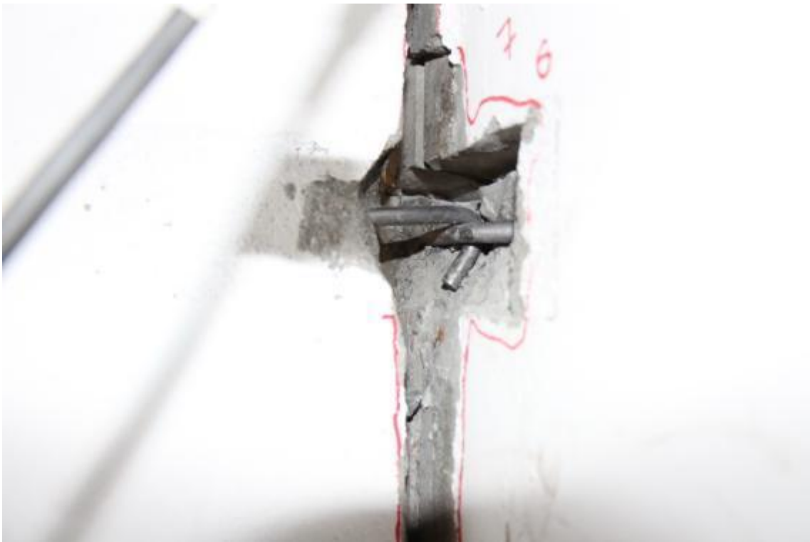
Figure 211. Flexural failure mode of the anchors embedded in the transversal walls – Top three-way joint.
