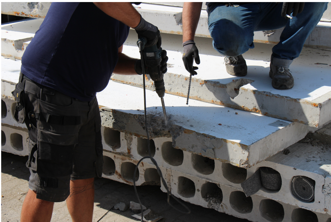
Figure 371. Removal of concrete close to a panel niche.
