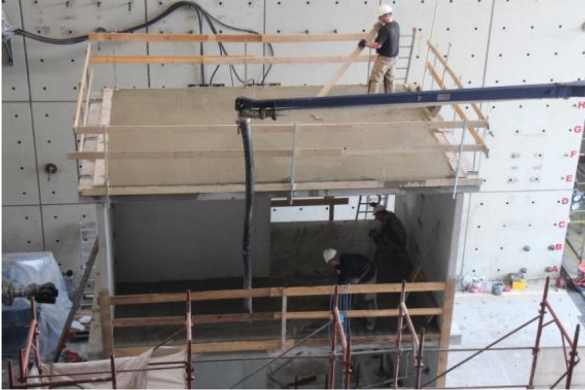
Figure 60. Casting of concrete slab topping – first storey, detail 3.
