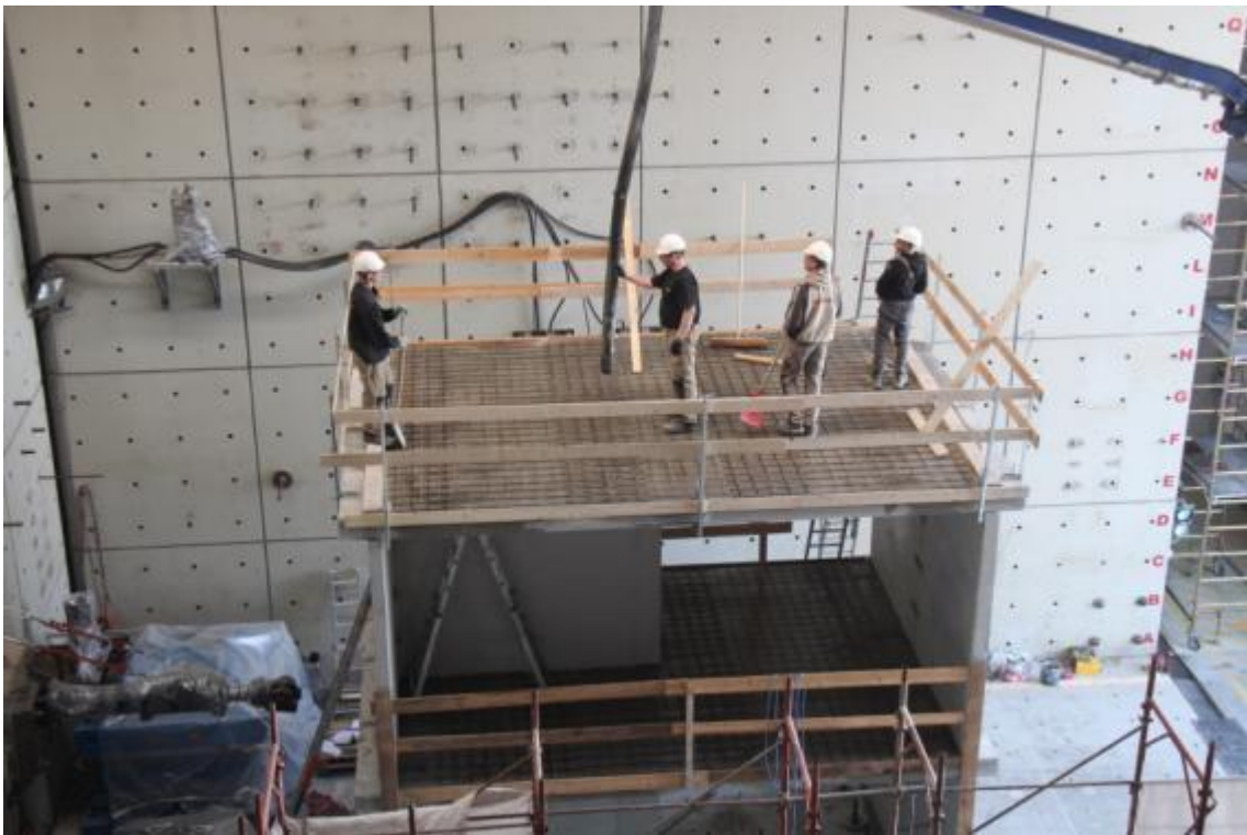
Figure 53. Casting of concrete slab topping – second storey, detail 1.
