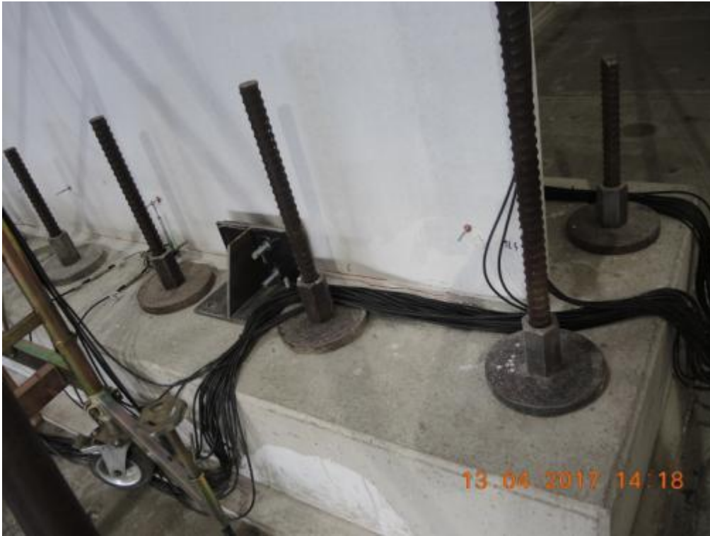
Figure 194. Formation of horizontal cracks at the base of the transversal walls – North side, opposite edge.
