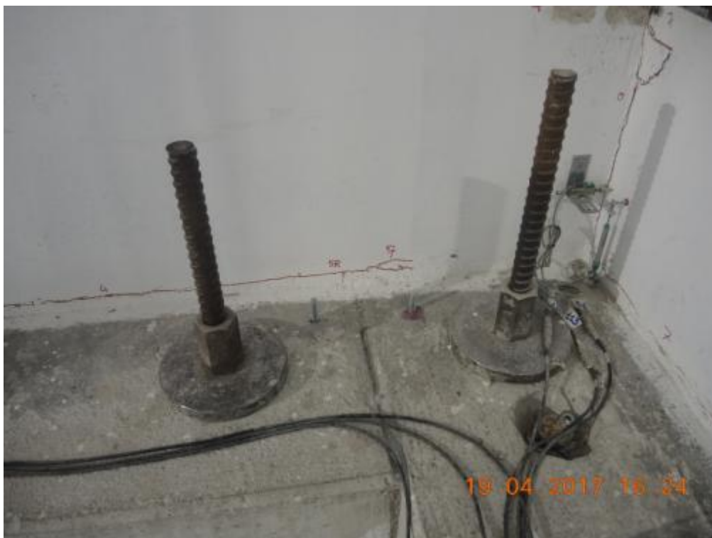
Figure 272. Crack pattern at the base of the ground-floor stability wall – West side.
