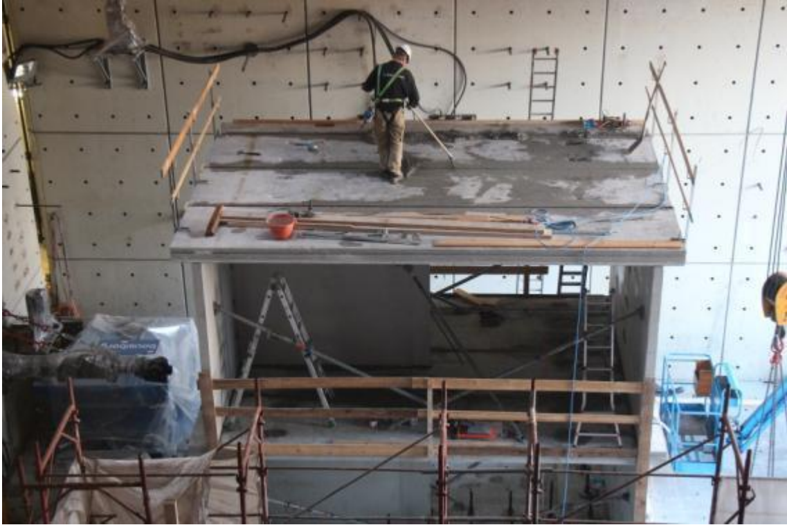
Figure 48. Detail of injection grout and final levelling.
