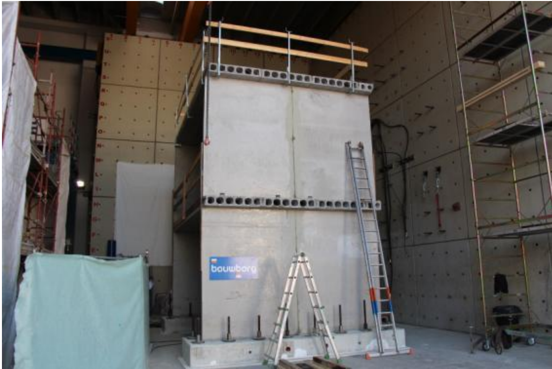
Figure 64. Overall view of EUC-BUILD4 specimen after levelling and finishing – side view.
