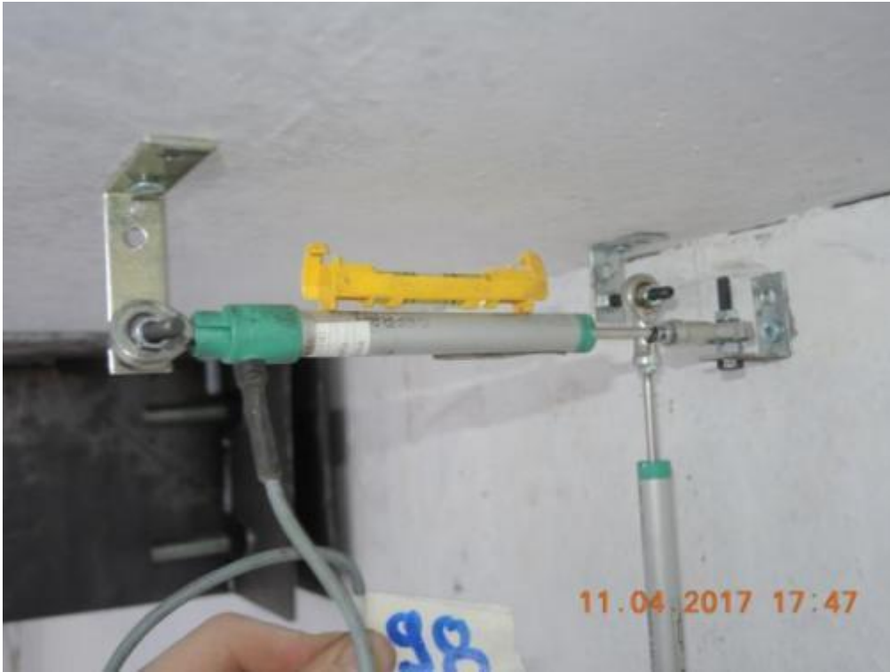
Figure 121. Detail of potentiometers installed at the base of a lateral wall.
