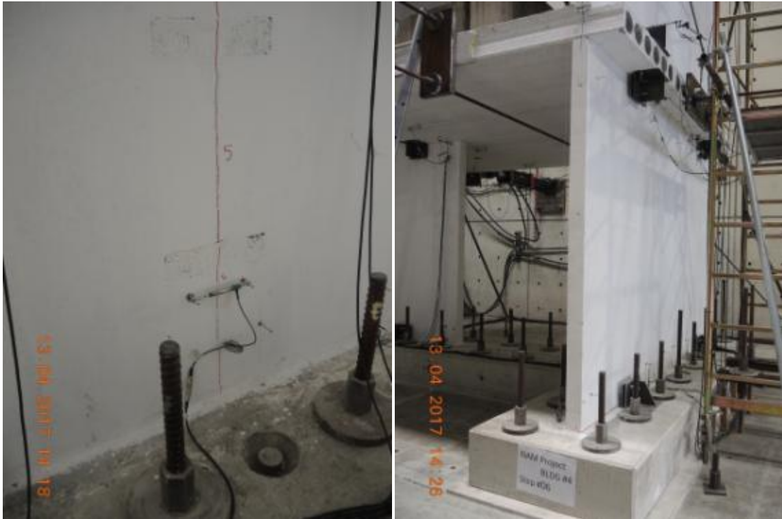
Figure 196. Propagation of vertical crack in the grout of panel-to-panel joint and loss of verticality.
