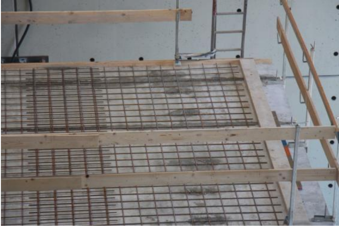
Figure 50. Steel reinforcement of concrete slab topping – second floor.
