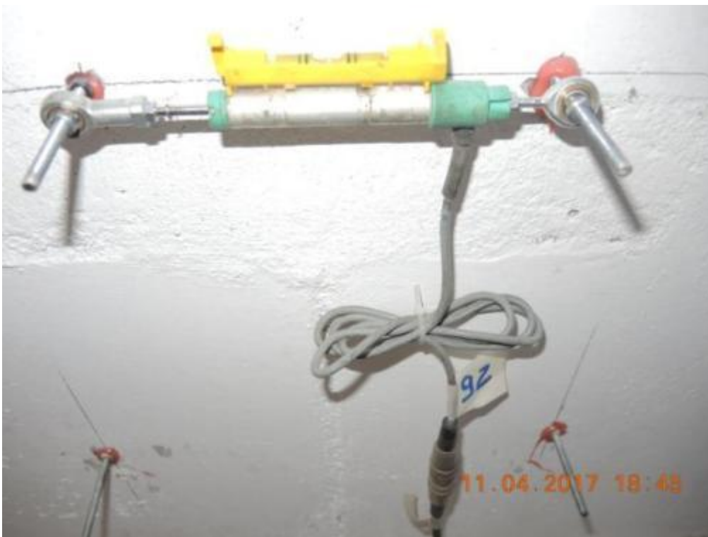
Figure 120. Detail of a potentiometer installed in correspondence to a panel-to-panel connection.
