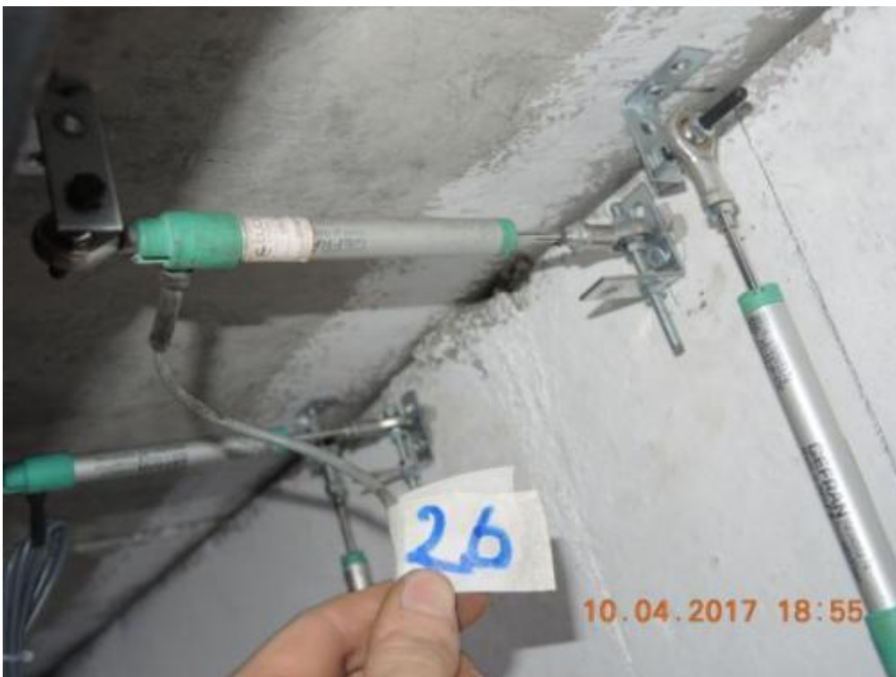
Figure 112. Instrumentation installed on lateral walls – Top of the wall, second storey, central zone.
