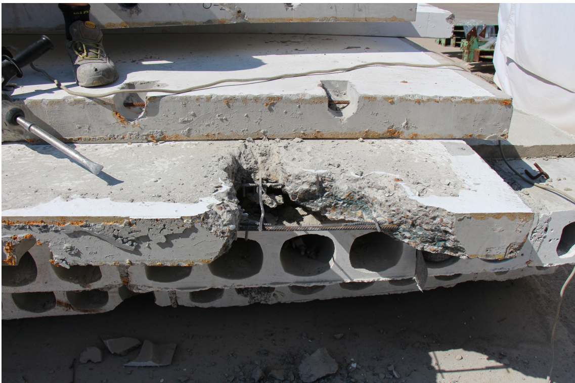
Figure 373. Detail of steel net and adjacent 10 mm diameter bar for the steel connectors.
