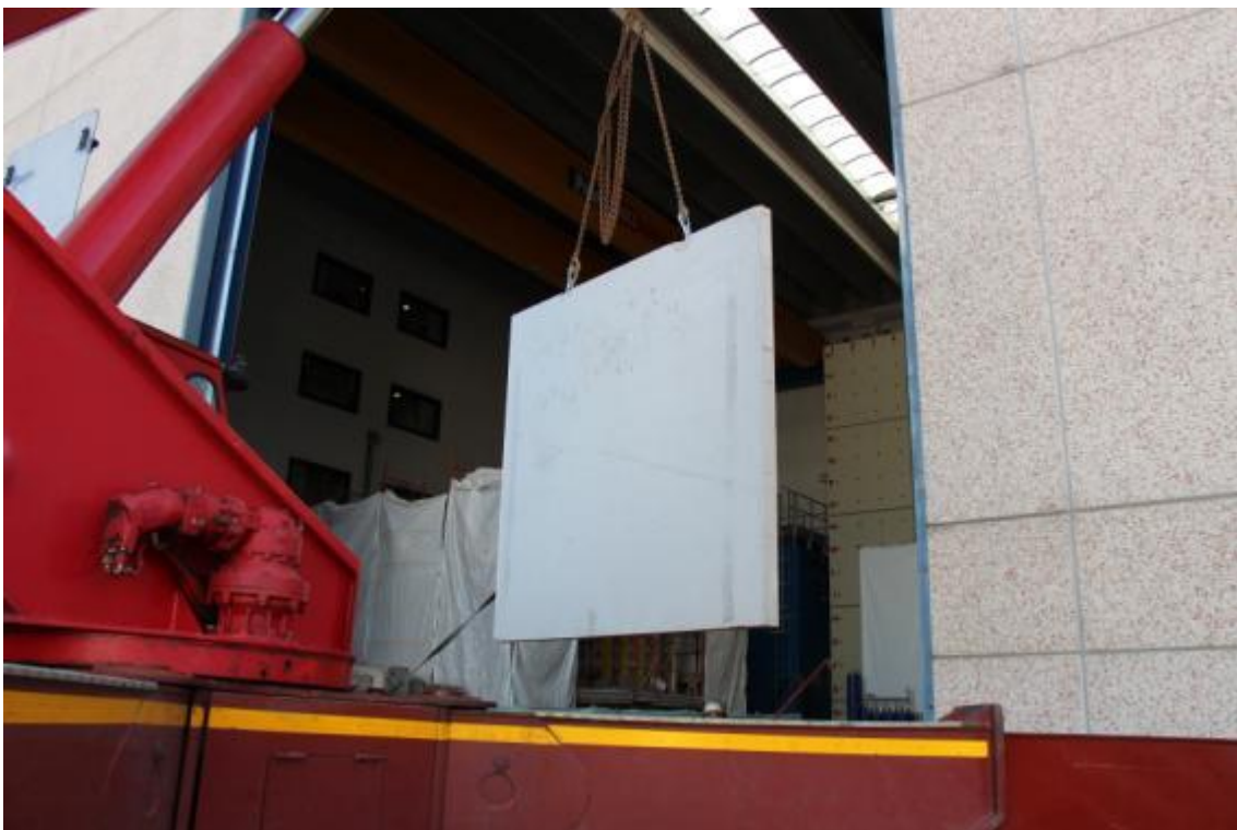
Figure 19. Uplift and transportation of precast wall-elements by means of cranes – detail 2.
