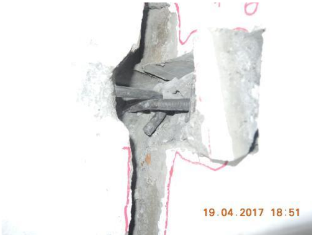
Figure 312. Detail of a three-way joint after removal of crushed grout – West side, North face.
