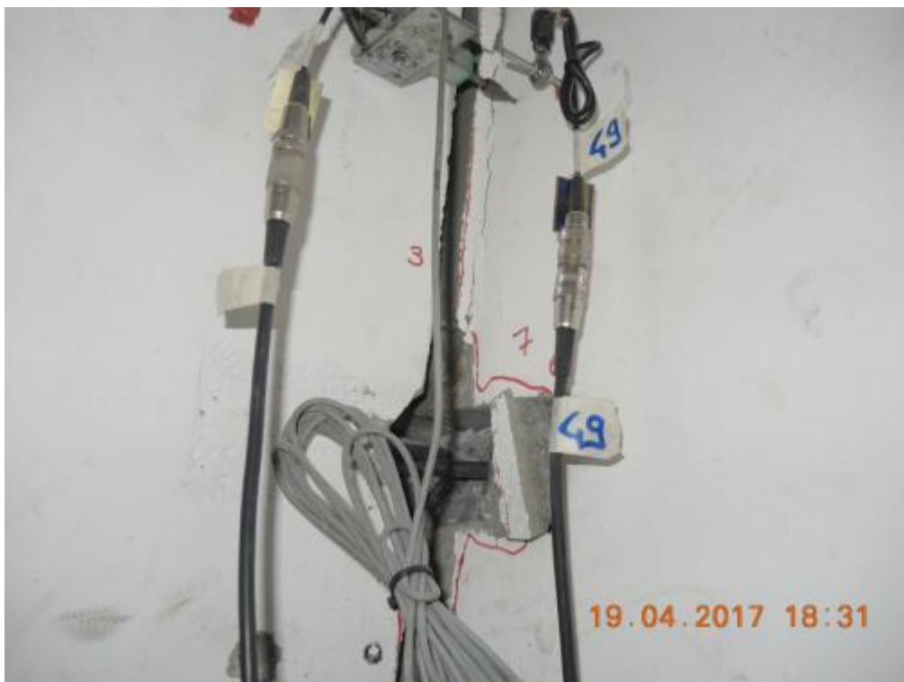
Figure 302. Detail of a three-way connection after test – West side, first storey.
