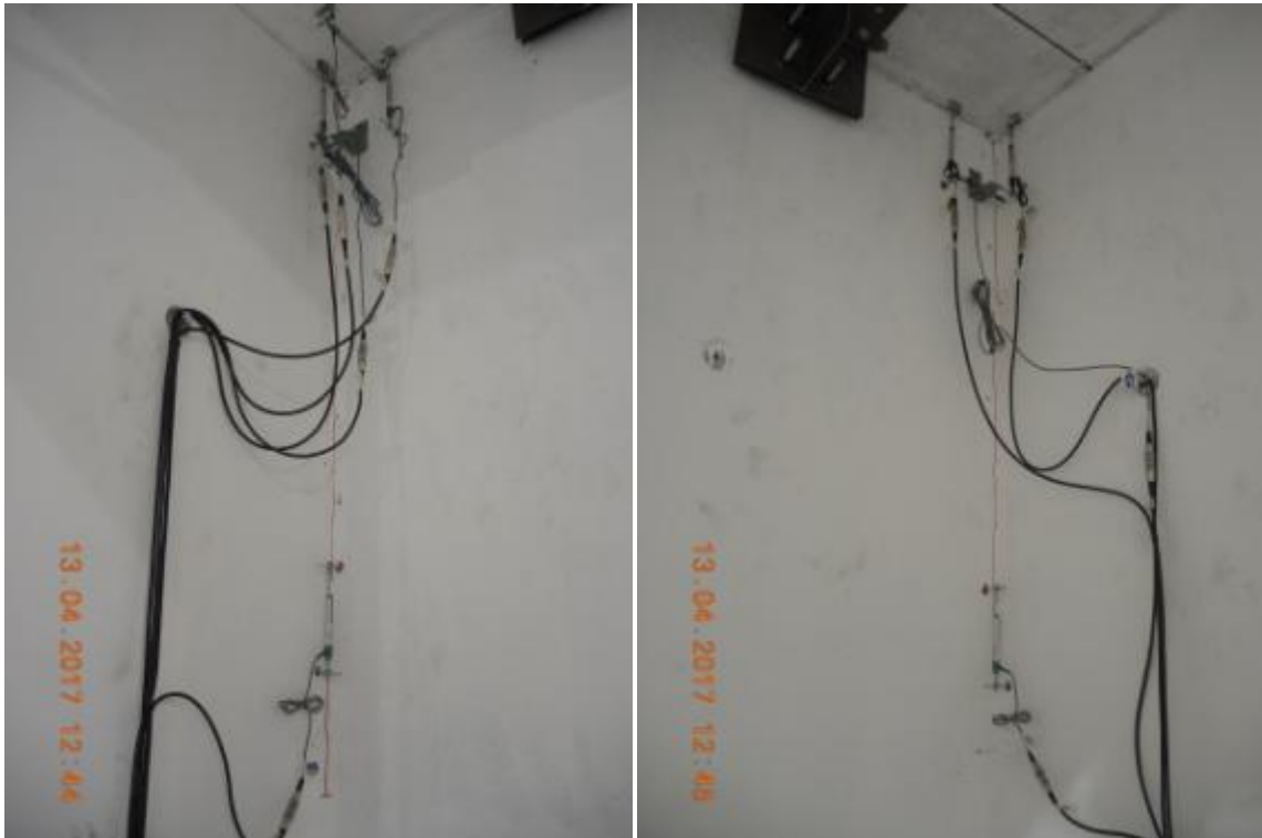
Figure 178. Development of vertical crack in the three-way panel connection (stability-to-lateral walls).
