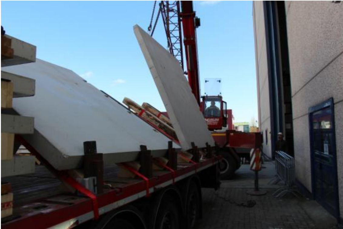
Figure 18. Uplift and transportation of precast wall-elements by means of cranes – detail 1.
