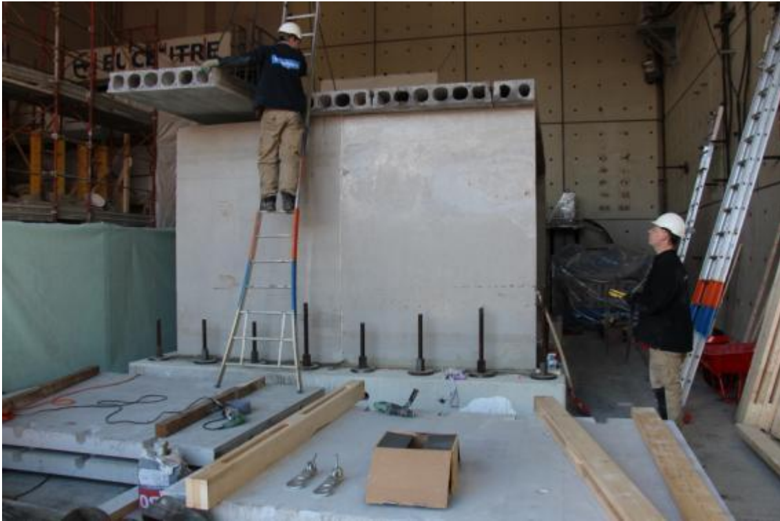
Figure 24. Installation of a precast hollow core slabs of the first floor.
