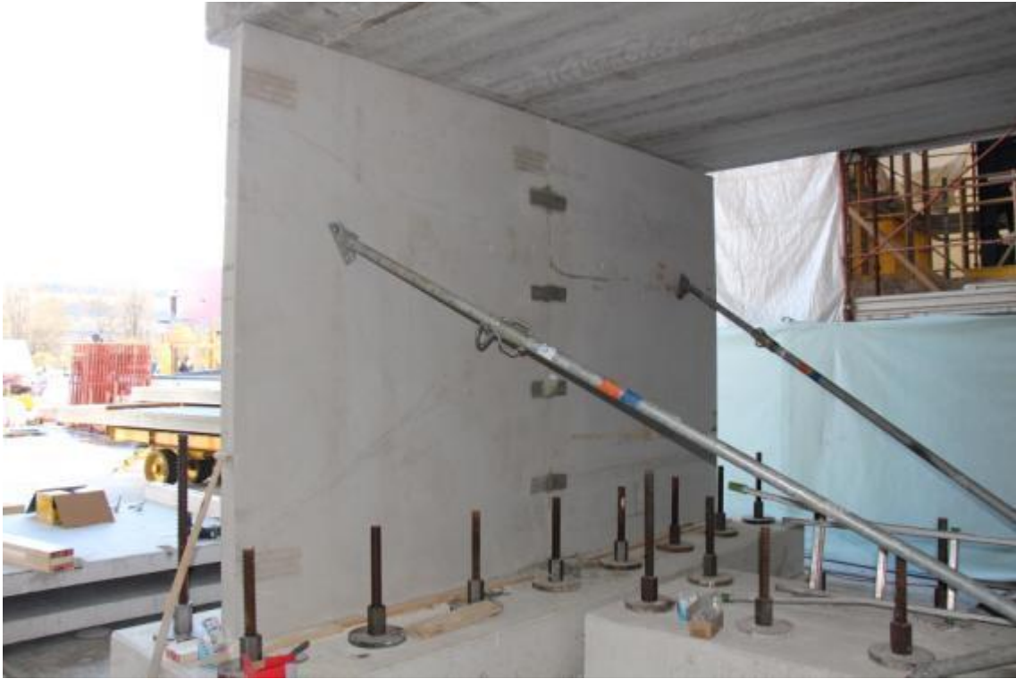
Figure 28. Detail of temporary steel diagonal props for stability purposes – lateral wall.
