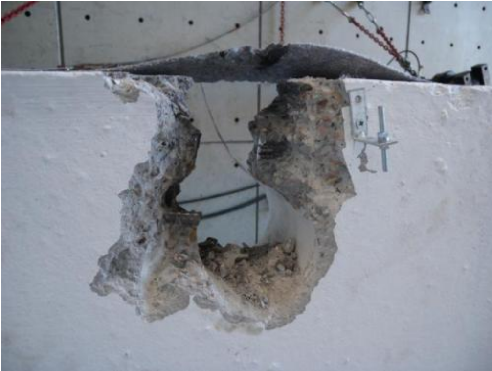
Figure 344. Detail of cut rebars in the ground-floor stability.
