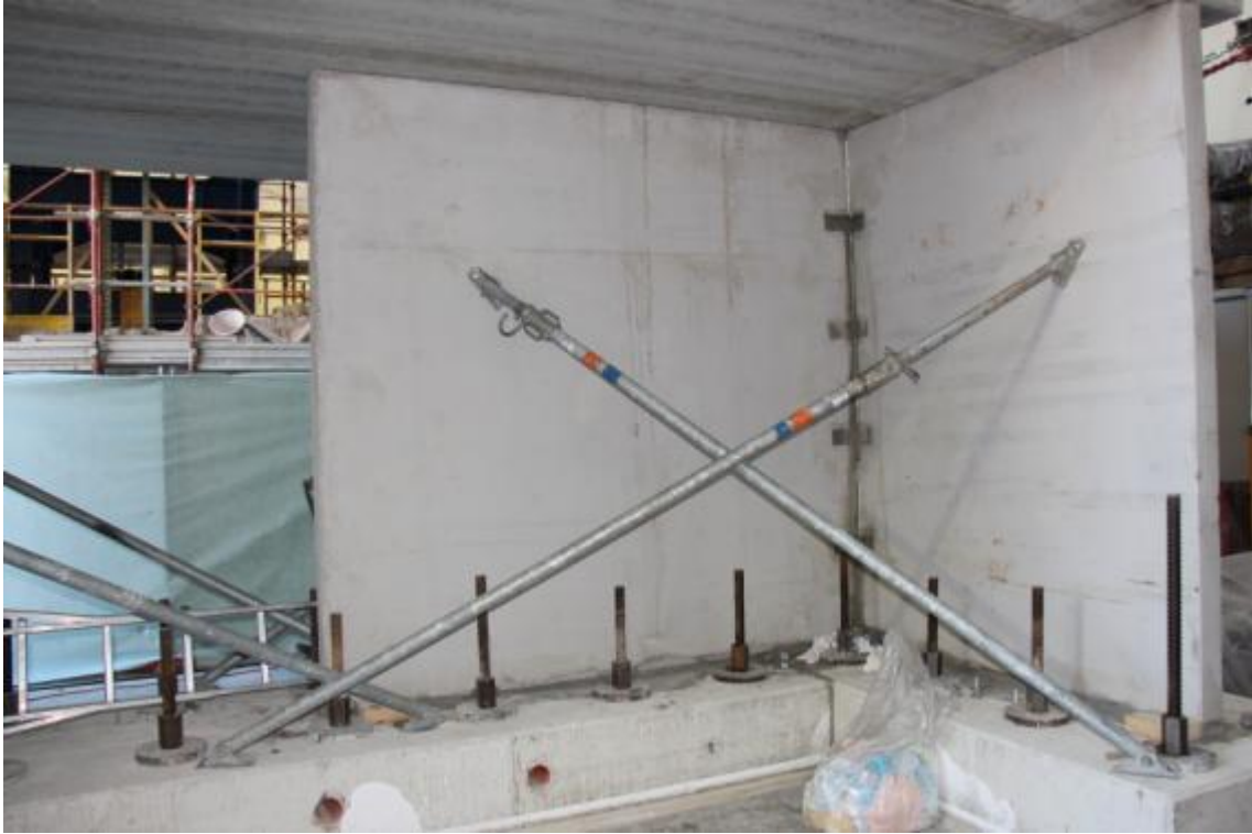
Figure 30. Detail of temporary props – stability and lateral walls.
