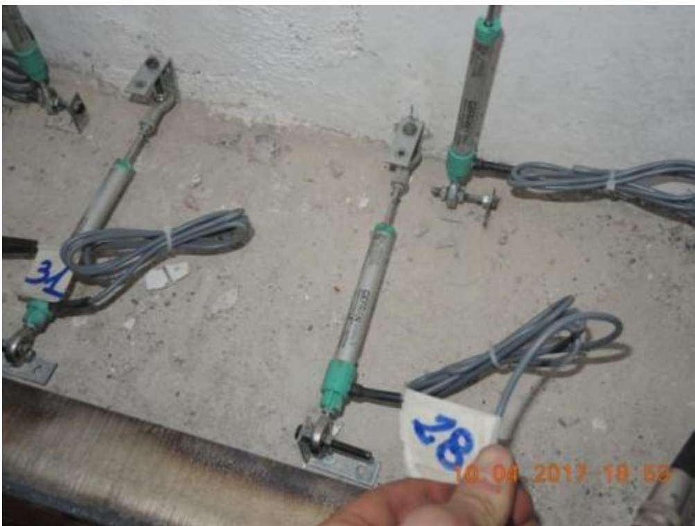
Figure 114. Potentiometers at the base of the lateral walls – Central zone, second storey.
