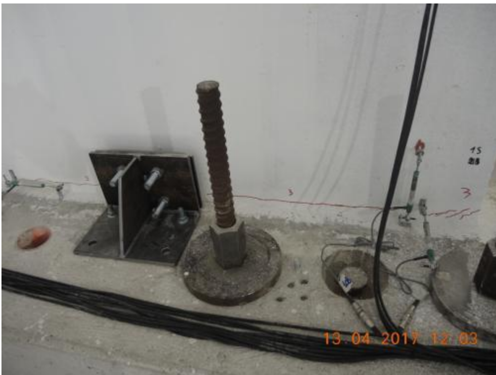
Figure 172. Crack pattern at the base of the first-floor stability wall – Opposite side.
