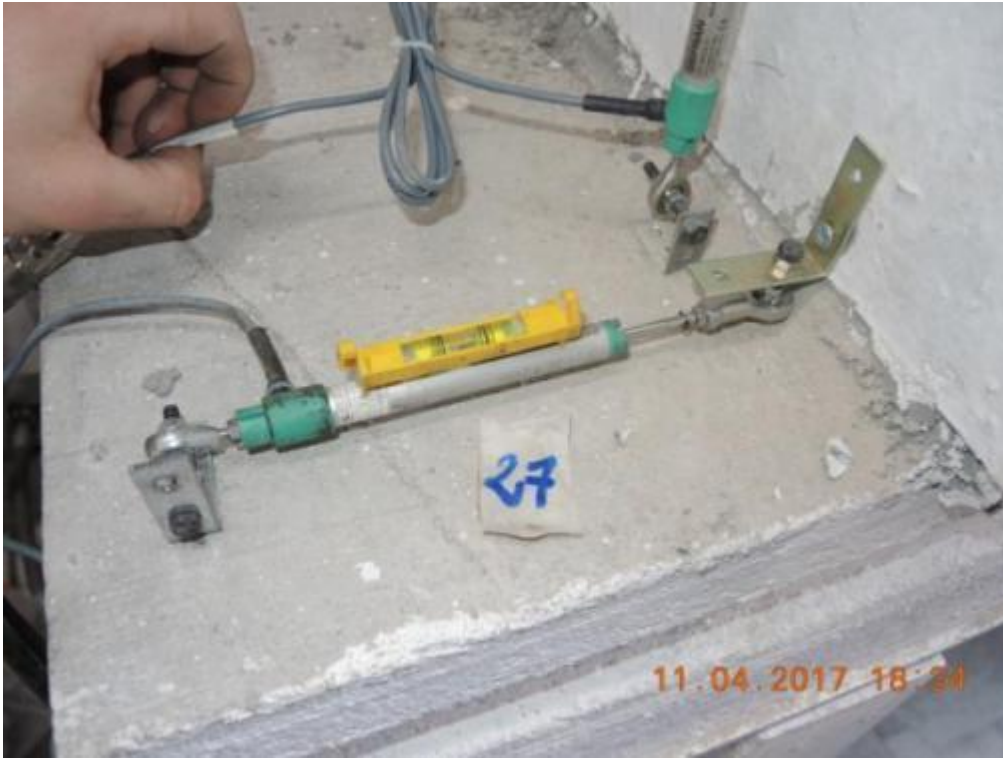
Figure 113. Detail of potentiometers at the base of lateral walls – External edge zone, second storey.
