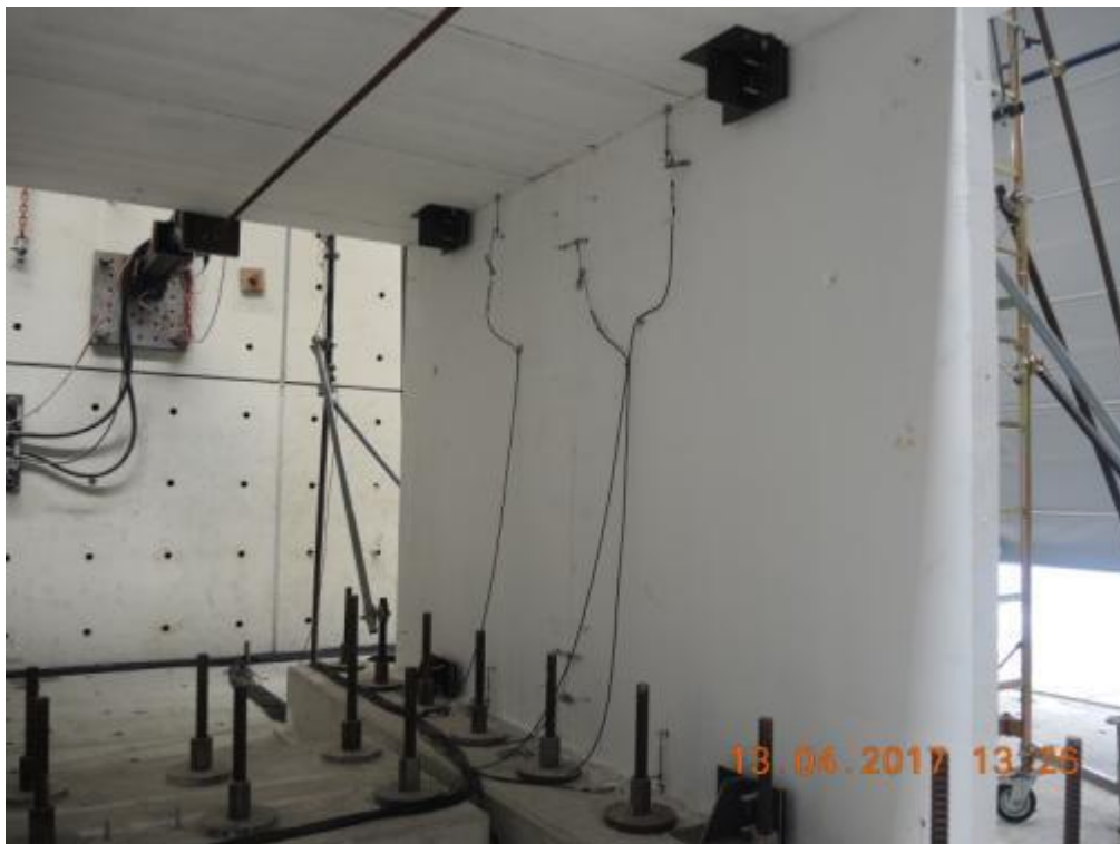
Figure 180. Development of a new crack along the two-way connection between lateral walls – North side.
