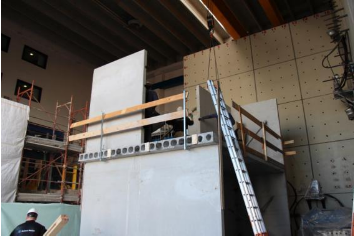
Figure 40. Installation of the stability wall of the second storey.
