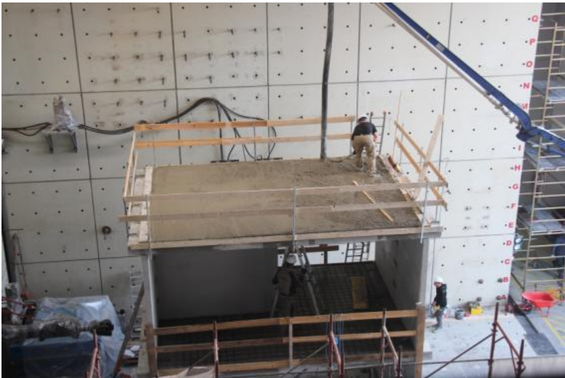
Figure 57. Casting of concrete – detail of levelling and finishing.
