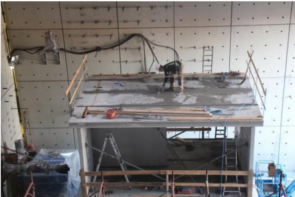
Figure 47. Detail of slab finishing via injection grout between the precast slab-elements.
