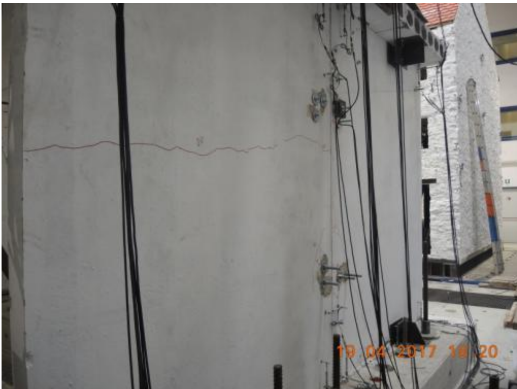
Figure 294. Full-depth/full-width/mid-height horizontal crack in lateral wall W1L2 – West side, South face.
