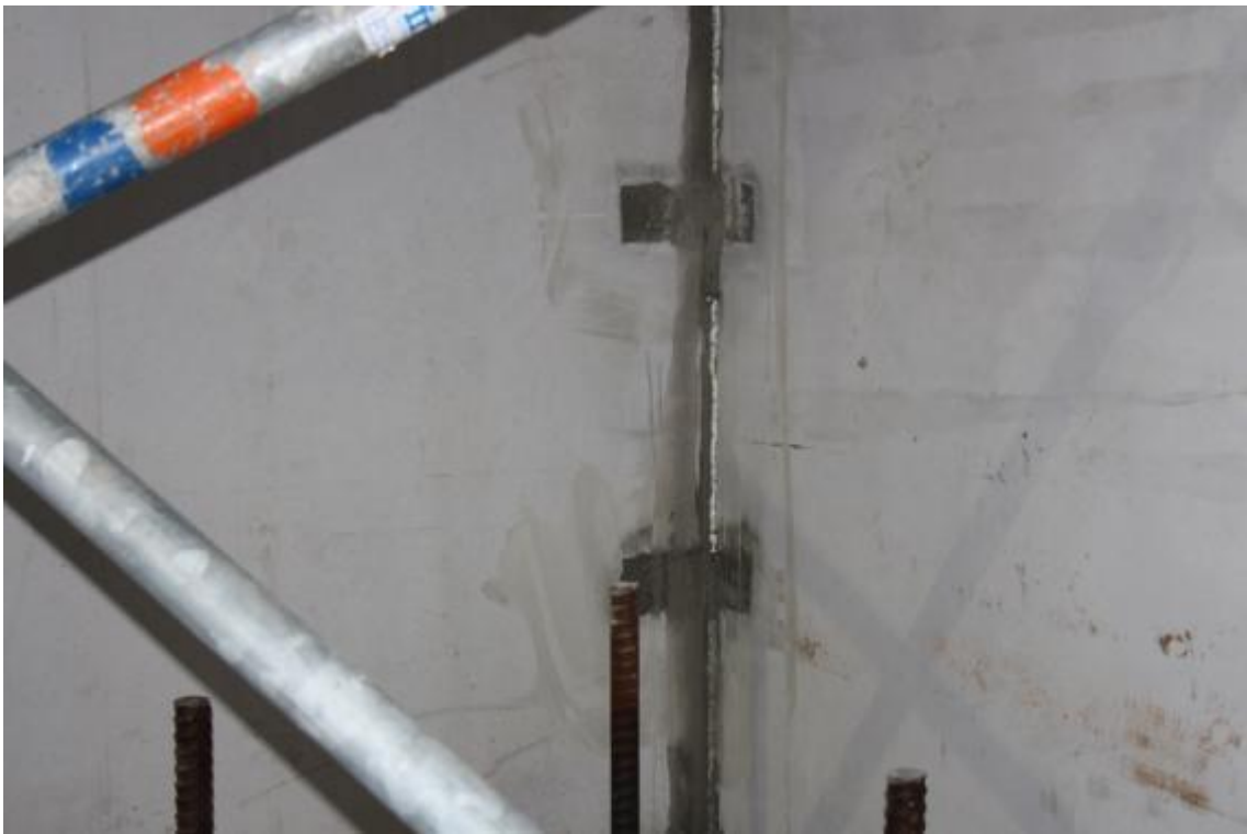
Figure 31. Detail of panel-to-panel three-way connections – stability wall.
