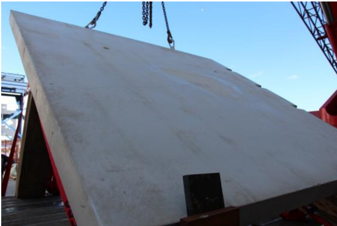
Figure 17. Uplift of precast wall-elements by means of cranes.
