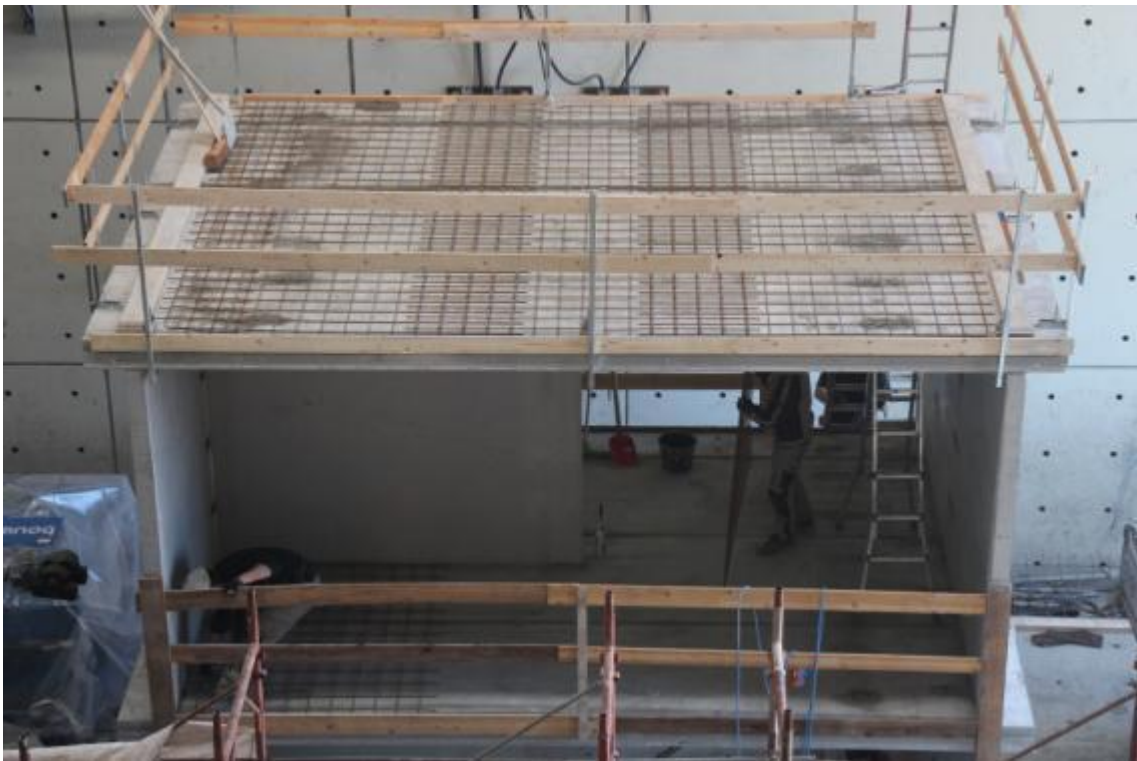
Figure 51. Arrangement of steel reinforcement before casting of concrete topping – second floor.
