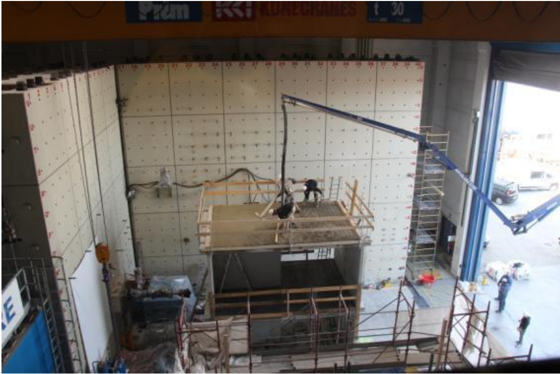
Figure 56. Casting of concrete slab topping – second storey, detail 4.
