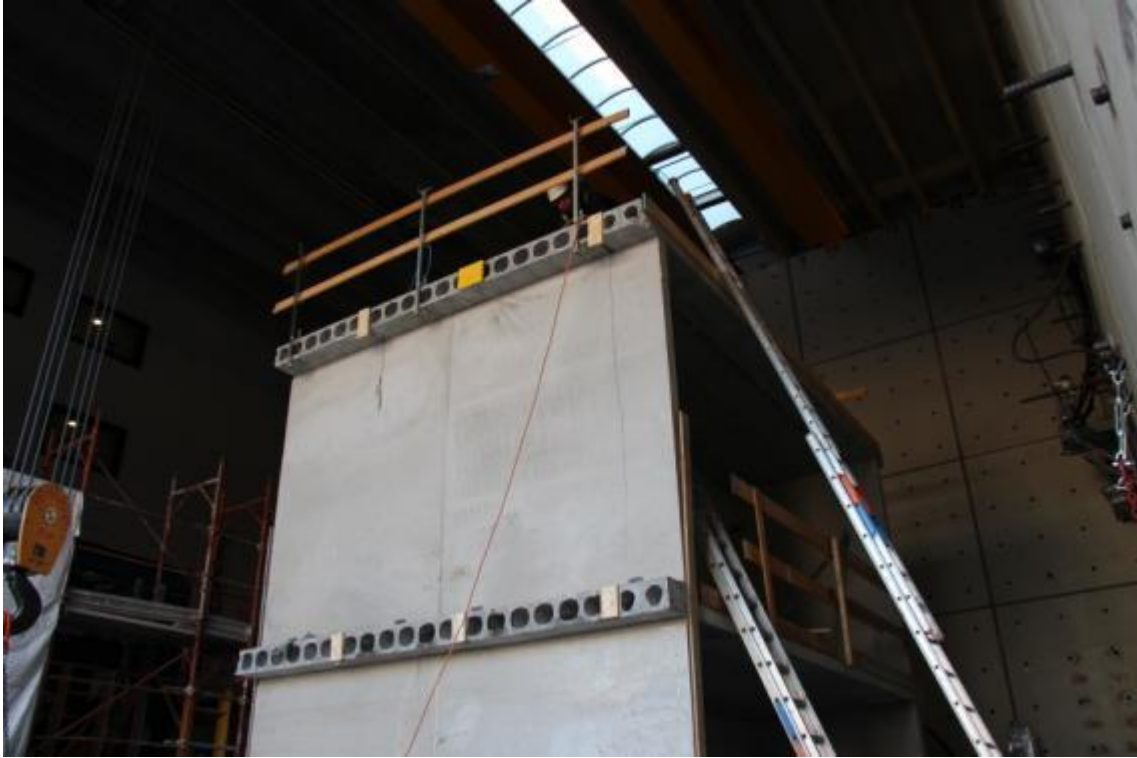
Figure 46. Preparation of the second storey for slab finishing.
