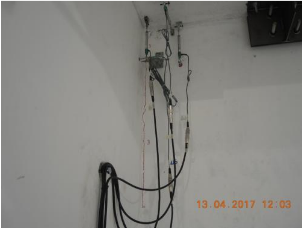
Figure 174. Crack opening in the connection between stability and lateral walls – Opposite side.
