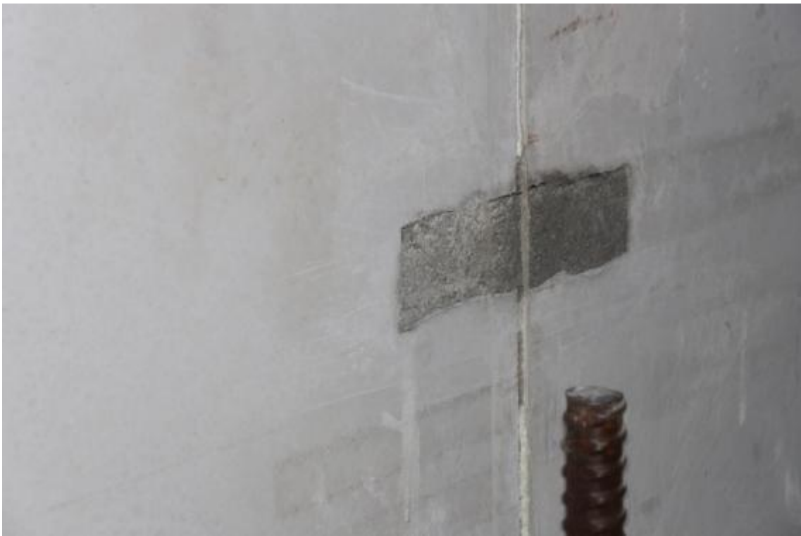
Figure 29. Detail of mortar in a panel-to-panel two-way connection – lateral wall.
