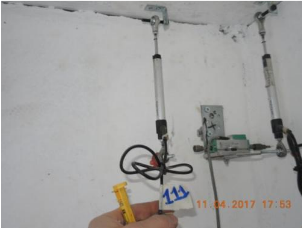
Figure 123. First-storey stability wall – Instrumentation for in-plane rocking at the top of the wall.
