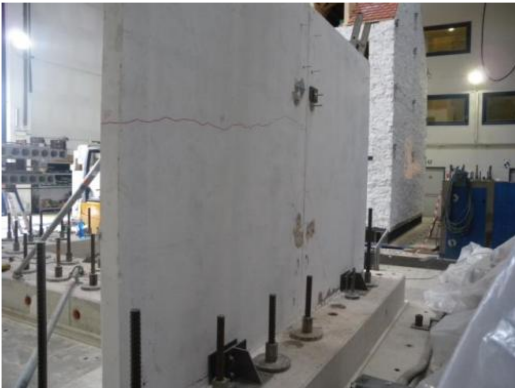
Figure 364. Global view of South-sided transversal walls during their dismantling – First storey.
