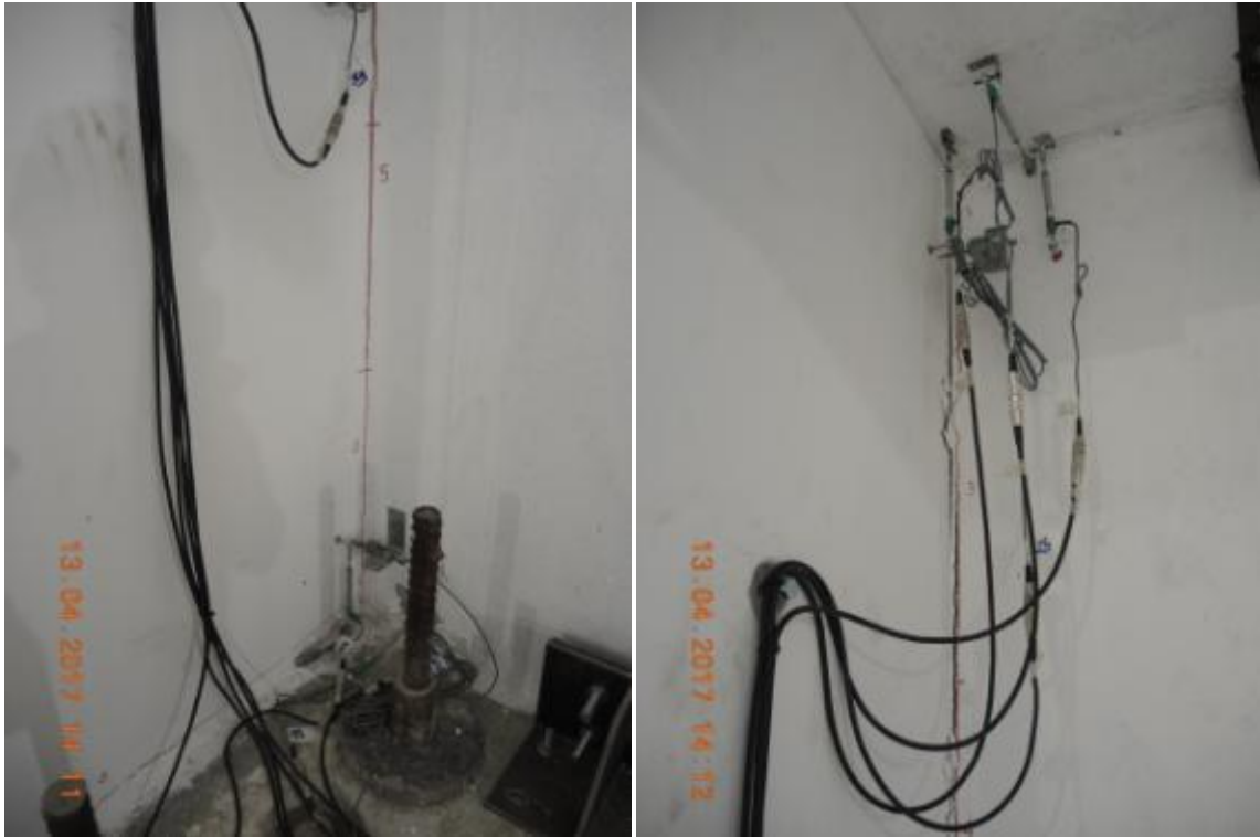
Figure 188. Three-way connection: propagation of vertical crack along the entire height of the stability wall.
