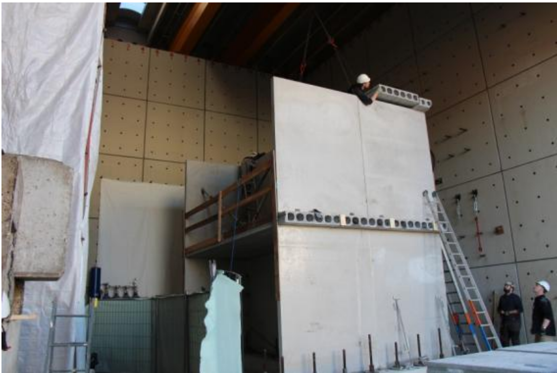
Figure 43. Installation of flooring system at the second floor level – side view.
