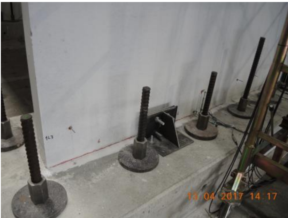
Figure 193. Formation of horizontal cracks at the base of the transversal walls – North side.
