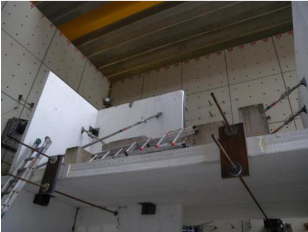
Figure 331. Detail of props for the second-storey stability wall and transversal walls.
