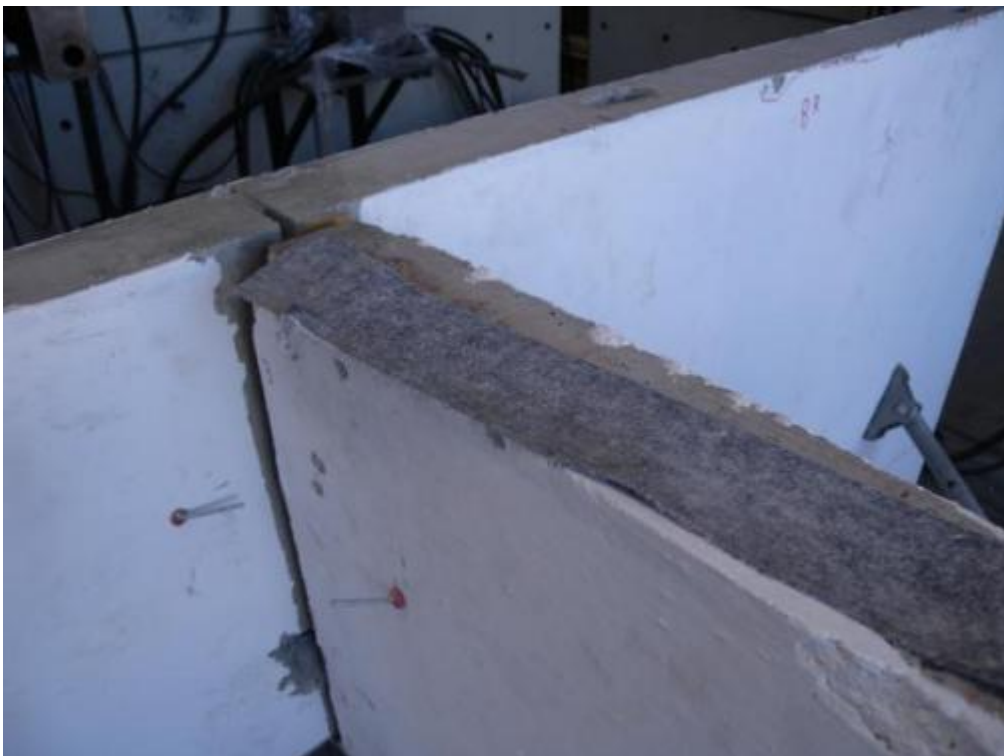
Figure 343. Detail of fabric felt underneath the first-floor slab – Stability wall, South side.
