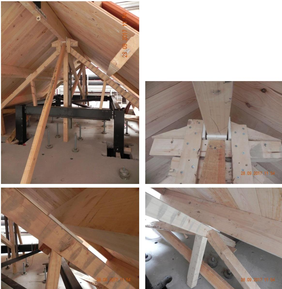
Figure 6.1 Support and guidance system.
