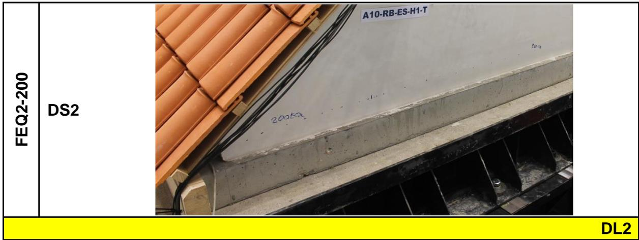
Figure 5.52 Evolution of damage in the gable walls along DL0 to DL2.
