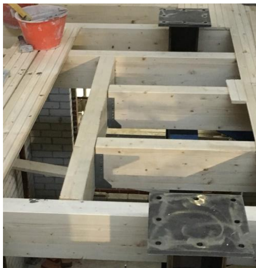
Figure 36 Timber floor framing: timber-to-timber details at staircase hole.
