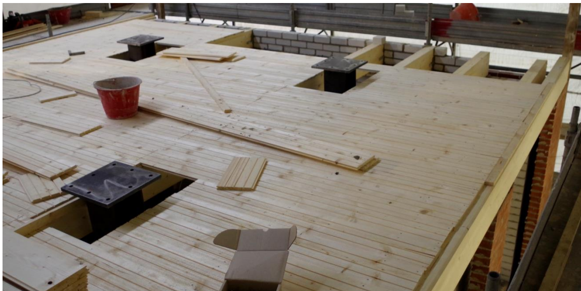
Figure 6 Prototype construction phases: second-floor timber structure.
