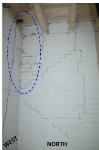
Figure 189 Crack C4 after EQ-NPR 100%: a) overview; b) zoom in.
