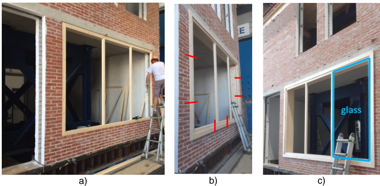
Figure 45 Ground-floor window frame external views: a) during construction, without side cover plates; b) screw locations; c) at the end of construction, with side cover plates and glass.
