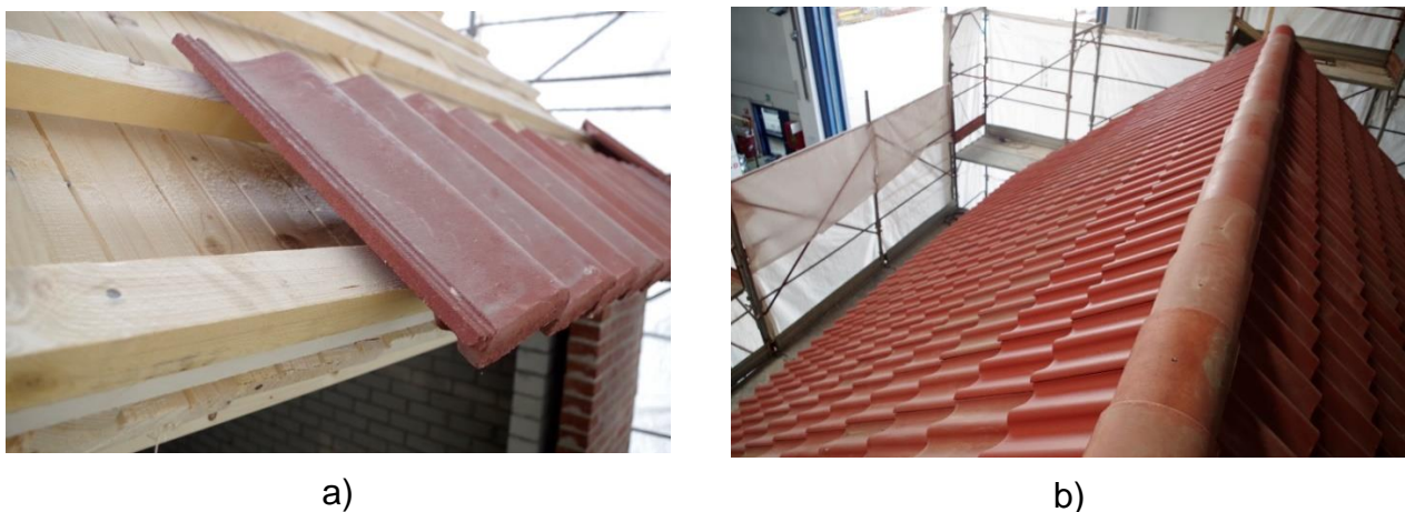
Figure 41 Roof finishes: a) tiles positioning; (b) roof end-construction.
