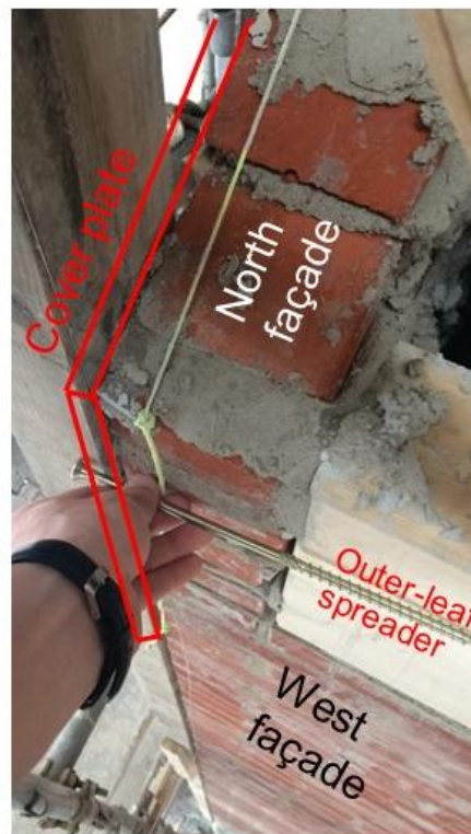
Figure 44 Detail of the cover plate connection to the outer-leaf spreader beam.
