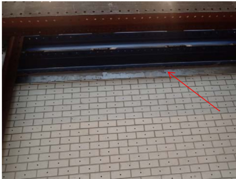
Figure 42: TUD-COMP-4: repair of the horizontal crack during the pre-test phase
