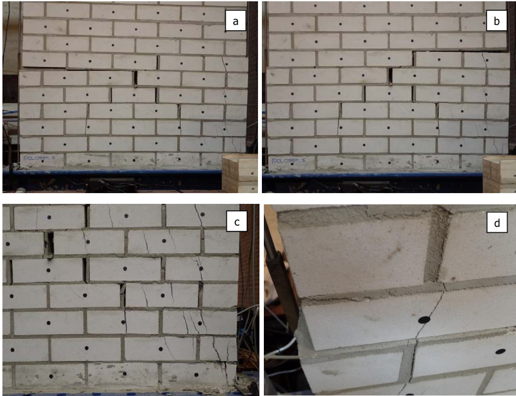
Figure 22: TUD-COMP-2: Crack pattern at failure for positive (a) and negative (b) drifts; details of the toe crushing (c) and sliding (d) at end stage.
