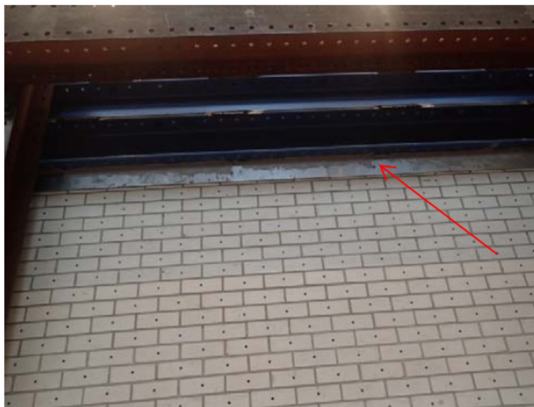
Figure 39: TUD-COMP-4: repair of the horizontal crack during the pre-test phase
