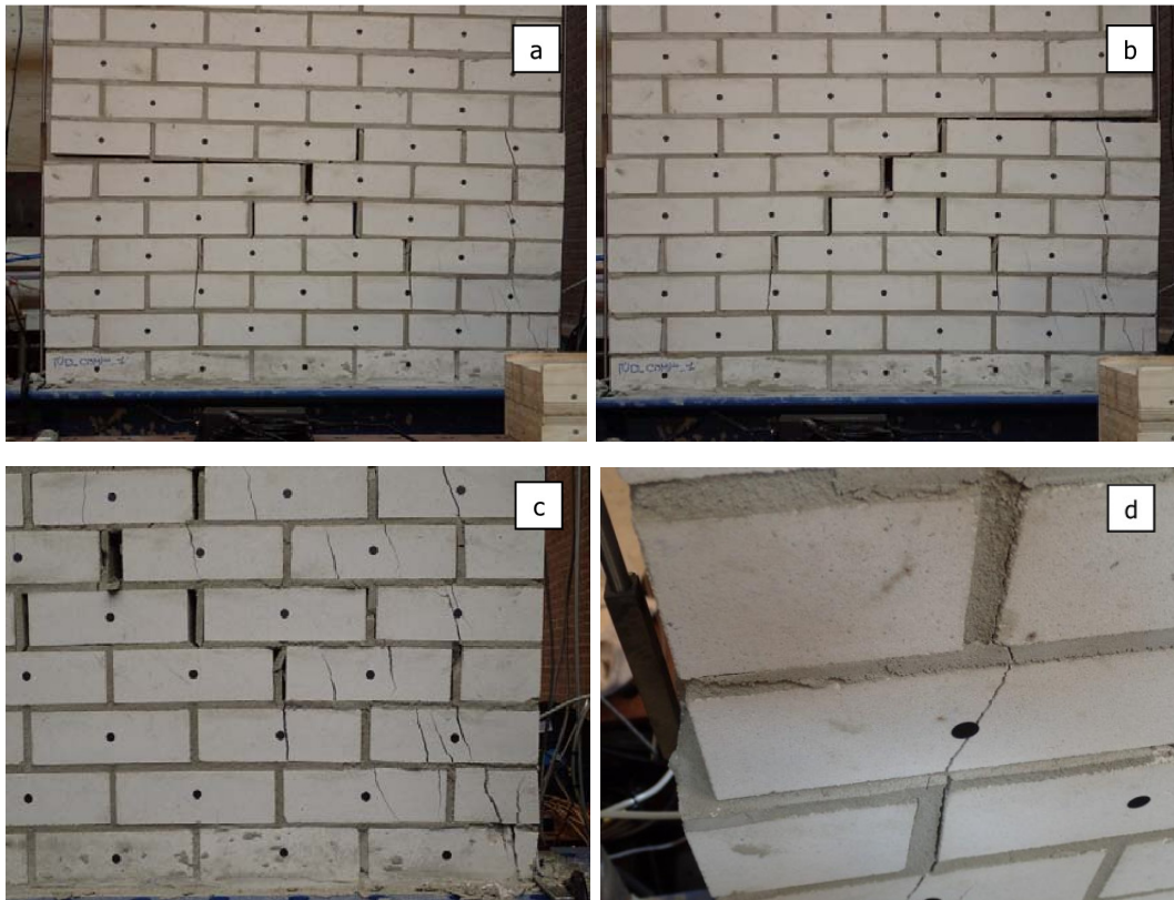
Figure 21: TUD-COMP-2: Crack pattern at failure for positive (a) and negative (b) drifts; details of the toe crushing (c) and sliding (d) at end stage.
