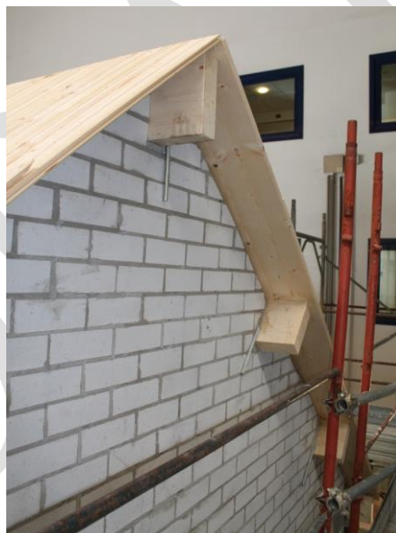
Figure 24. Roof and c.s. gable - South side
