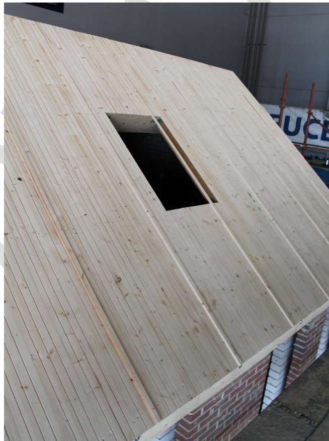
Figure 26. Roof - West side
