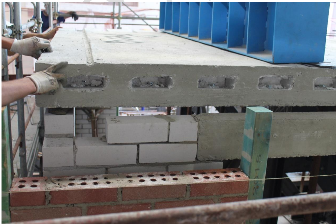
Figure 16. Positioning of the r.c. slab of the first floor - East side
