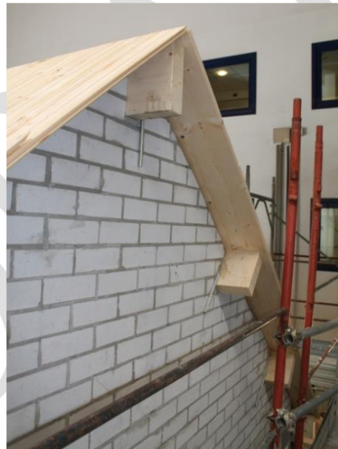
Figure 24. Roof and c.s. gable - South side
