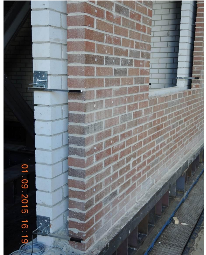
Detail of installation of markers on the CS inner wall.
