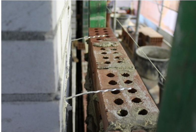
Figure 13. Laying of the ties
