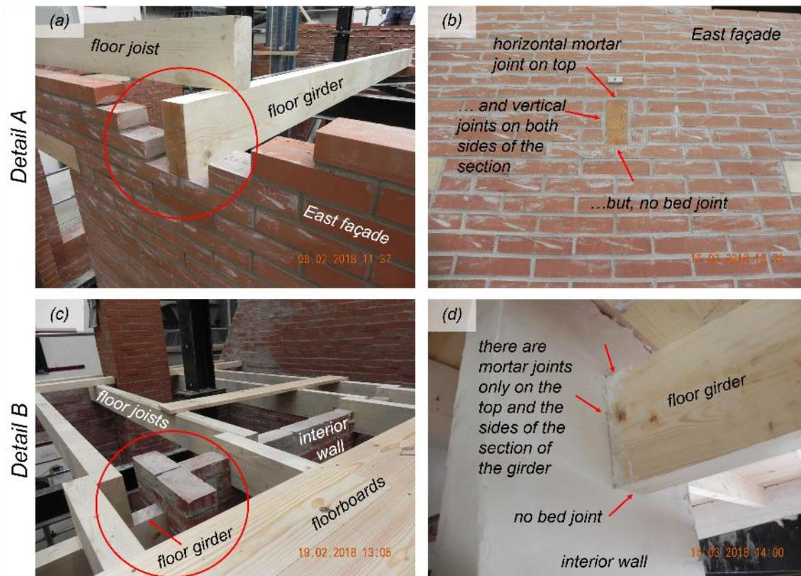
Figure 2.10 Construction details of the floor: (a, b) connection of the floor girder to the East wall; (c, d) support of the floor girder on the interior wall.
