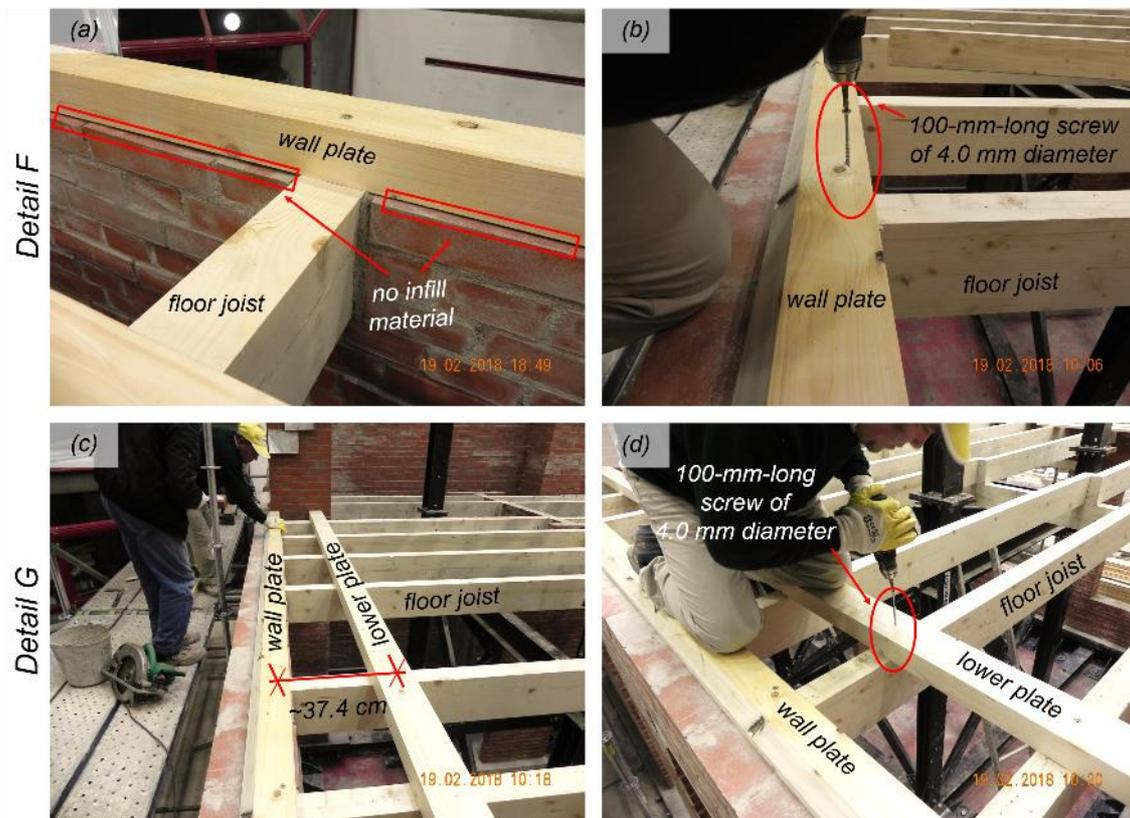
Figure 2.12 Construction details of the floor: (a, b) connection of the wall plates to the floor joists; (c, d) connection of the lower plates to the floor joists.
