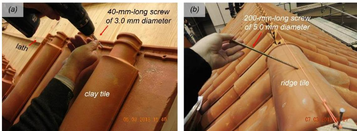
Figure 2.23 Roof finishing with clay tiles: (a) fastening of the tiles on timber laths; (b) attachment of the ridge tiles to the ridge beam.
