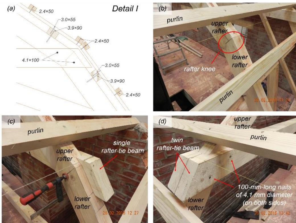
Figure 2.16 Construction details of the rafters' knee: (a) detail drawing of the joint; (b) contact point of the gambrel rafters; (c) realisation of the lap joint; (d) completion of the joint with a double tie-beam.
