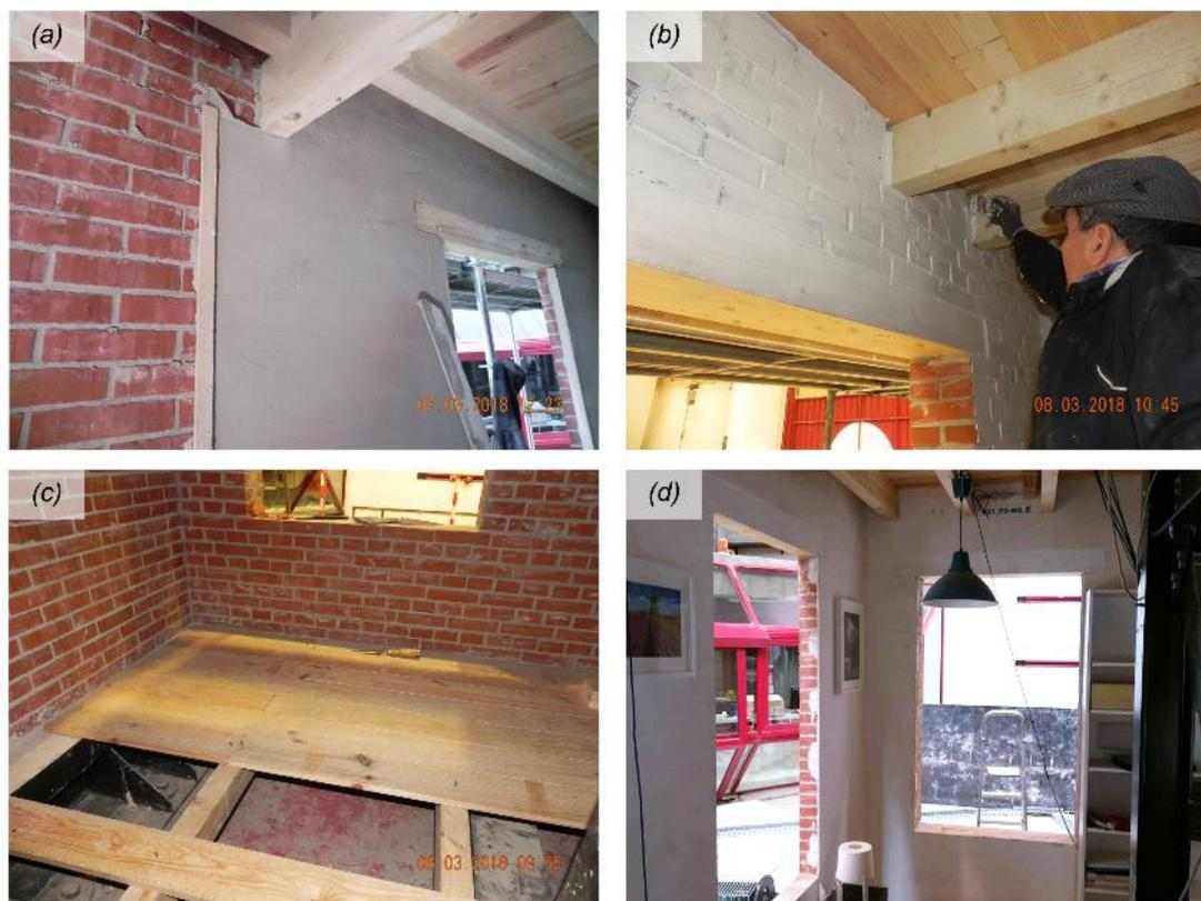
Figure 2.27 Building finishing: (a) rendering of the East wall; (b) painting of the interior side of the walls; (c) timber floor above the foundation; (d) furnishing.
