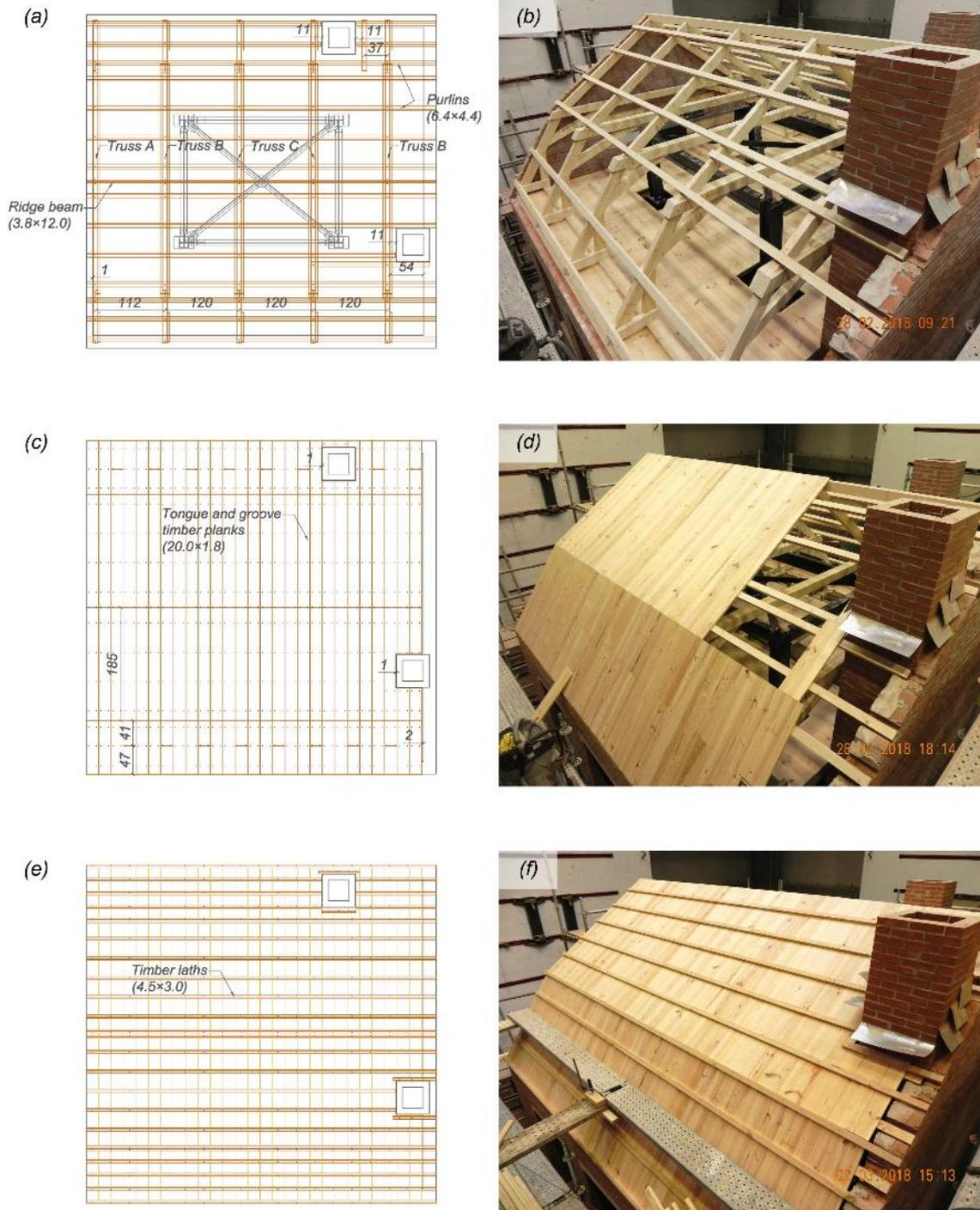
Figure 2.14 Roof framing: (a) roof framing plan; (b) roof trusses spanning between the South and North walls; (c) roof planks layout; (d) roof sheathing during construction; (e, f) strips of laths installed to fasten the tiles. Units of cm.
