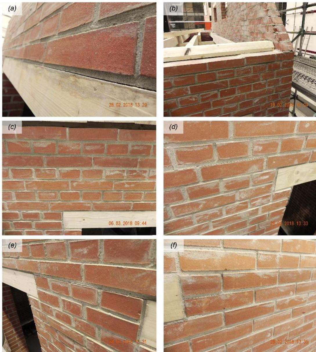
Figure 2.28 Damage detected prior to the testing: (a) cracking at the mortar-timber interface; (b, c) cracking due to floor joists-wall interaction; (d) crack propagation from the corner of an opening; (e) crack propagation between two lintels of the North façade; (f) crack propagation between the lintels of the East gable wall.
