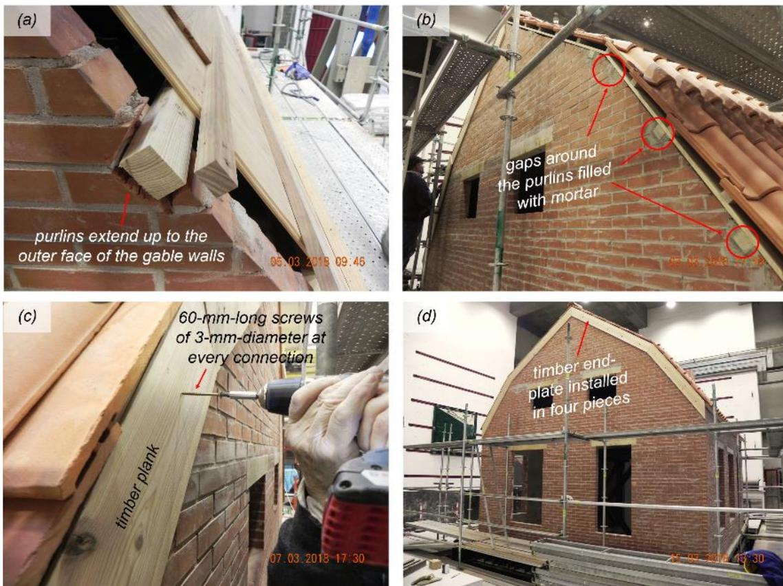
Figure 2.21 Construction details of the roof: (a, b) connections between the purlins and the East gable; (c, d) planks blocking the purlins outside the East gable wall.
