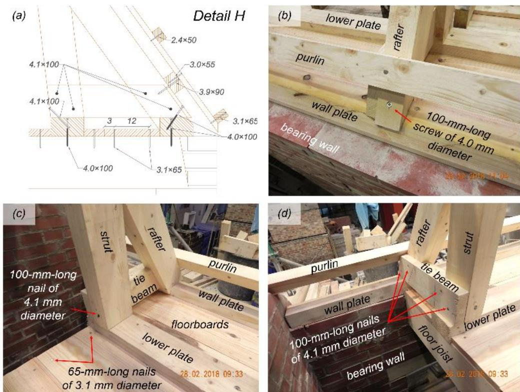
Figure 2.15 Construction details of the roof truss supports: (a) detail drawing of the truss supports; (b) connection of the truss rafter to the wall plate; (c, d) connection details at the lower ends of the truss.
