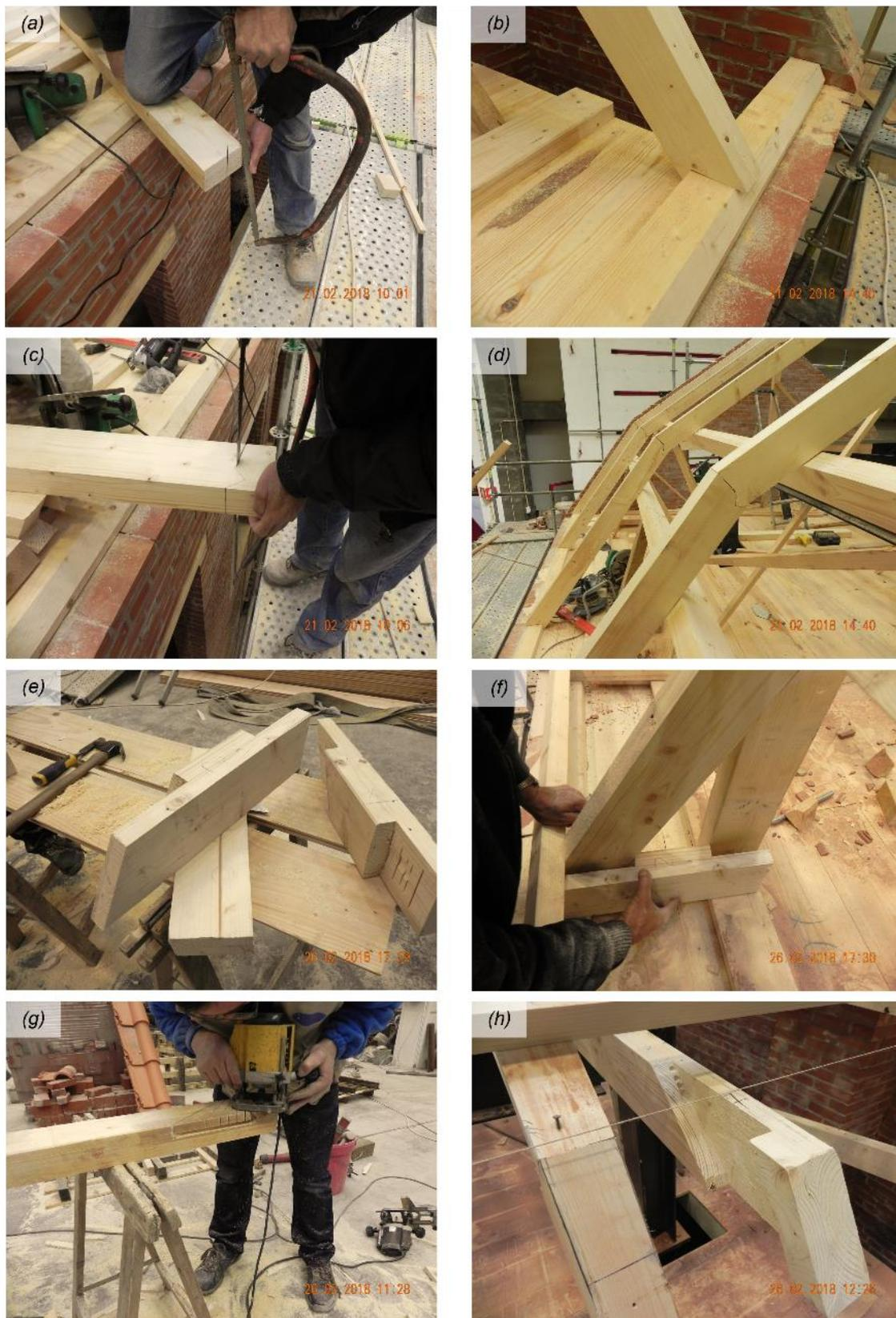
Figure 2.18 Crafting the connections of the timber roof trusses: (a, b) rafters toe; (c, d) rafters knee; (e, f) lower tie beams; (g, h) mortise joint.
