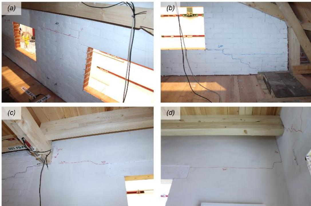
Figure 6.23 Damage on the East façade after test SC2-300%: (a, b) cracks on the gable wall; (c) cracks around the support of the floor girder; (c) horizontal cracking above the level of the windows.
