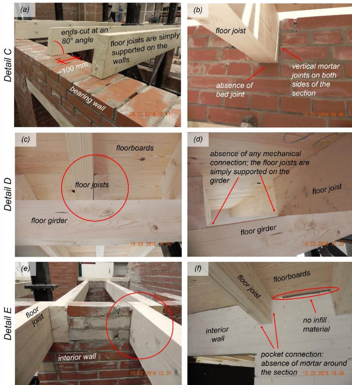
Figure 2.11 Construction details of the floor: (a, b) support of the floor joists on the perimeter walls; (c, d) support of the floor joists on the central girder; (e, f) connection of the floor joists with the interior wall.
