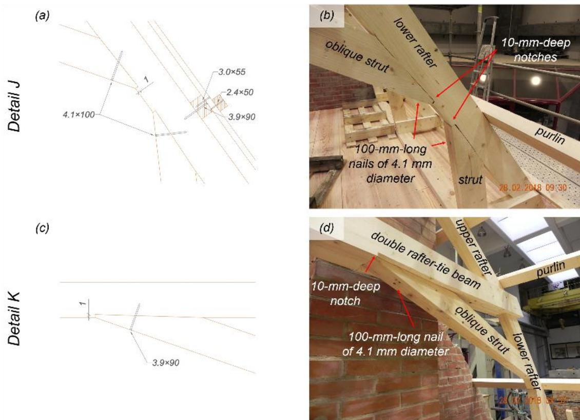
Figure 2.17 Construction details of the roof trusses: (a, b) connection of the struts to the lower gambrel rafter; (c, d) connection of the struts to the double tie-beam.
