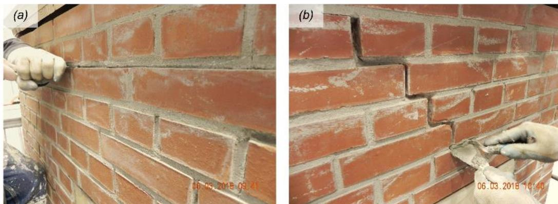
Figure 2.30 Mortar joints repointing: (a) removal of the old mortar joint; (b) filling with new mortar.
