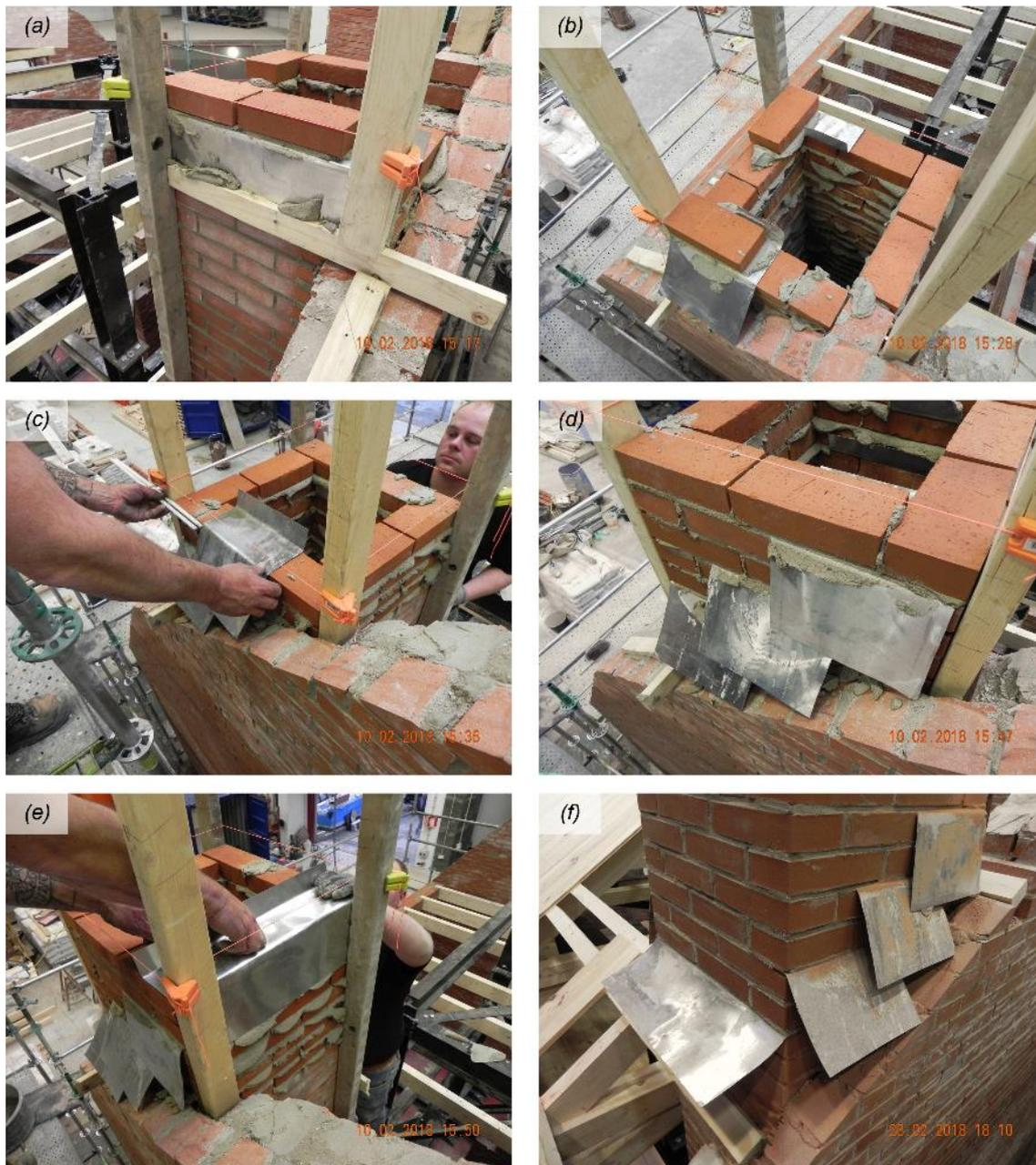
Figure 2.25 Construction details of the West chimney flashing: (a) wide piece of zinc at the chimney apron; (b) bottom layer of step flashing; (c) installing sheets of zinc in mortar joints; (d) step flashing on the chimney side; (e) piece of zinc at the chimney head; (f) finished flashing.
