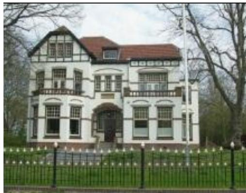
Figure 7.7 Examples of some of the typical unreinforced masonry building typologies found in the Groningen region
