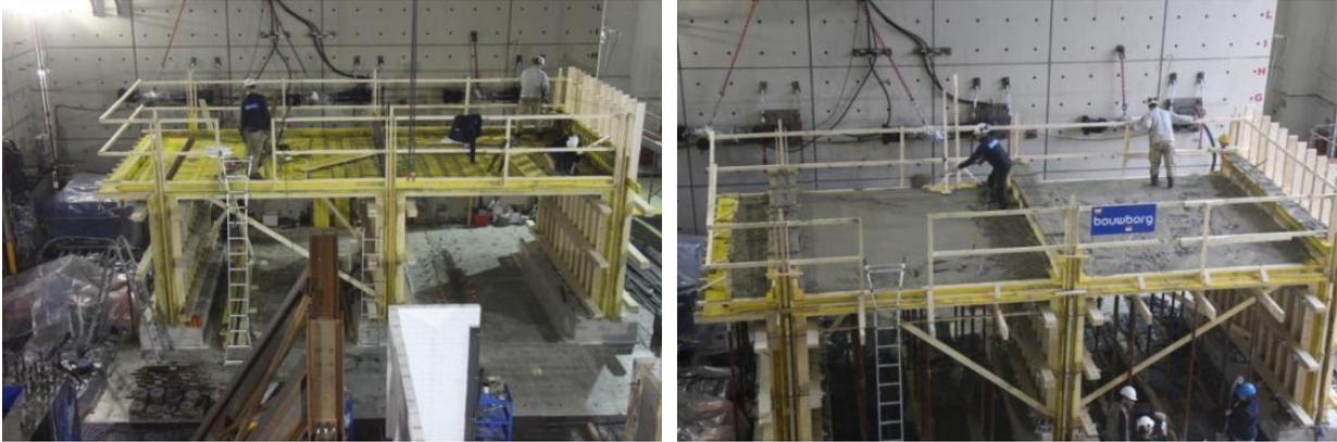
Figure 7.29 The cast-in-place concrete building under construction in the laboratory (Ref. 15). The specimen was built in the laboratory by the Groningen construction company Bouwborg.
