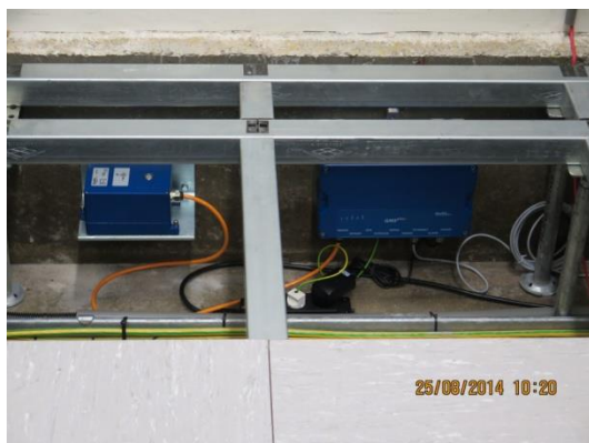
Figure 5.1 Installation of a building sensor at the basement of a building.
