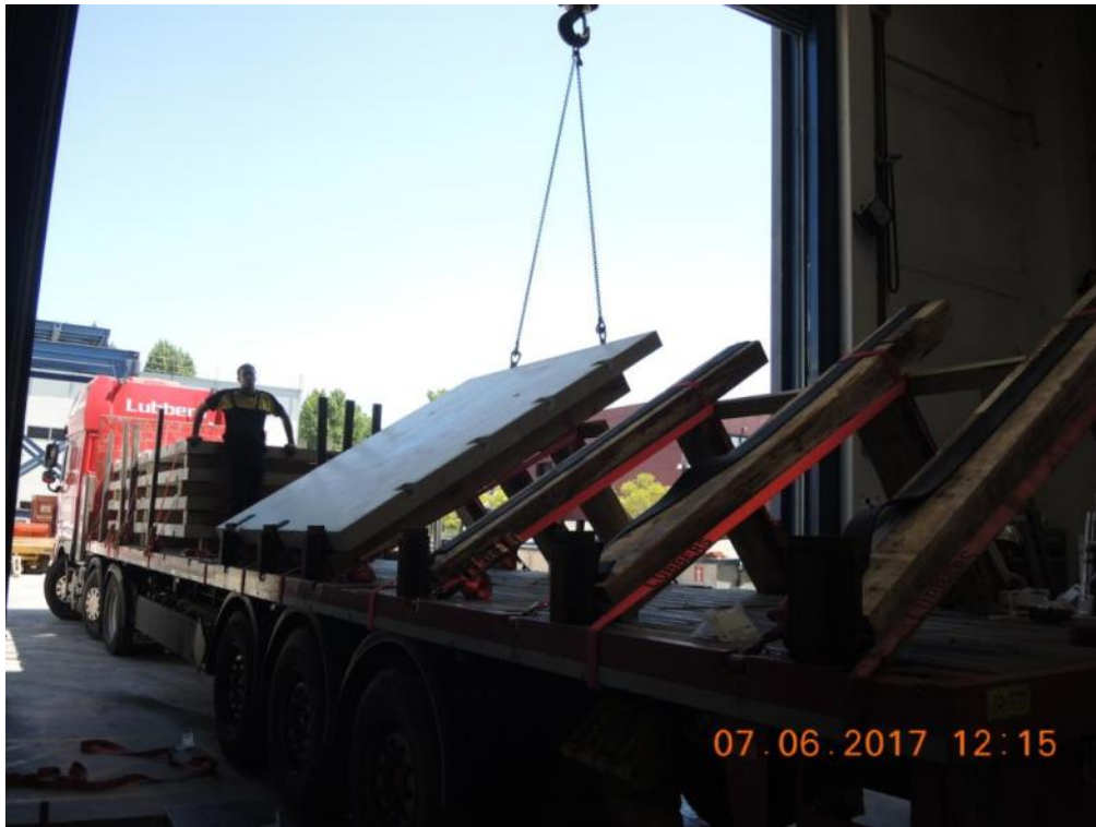
Figure 102. Detail of the static scheme adopted to store stability wall panels on truck for transportation.
