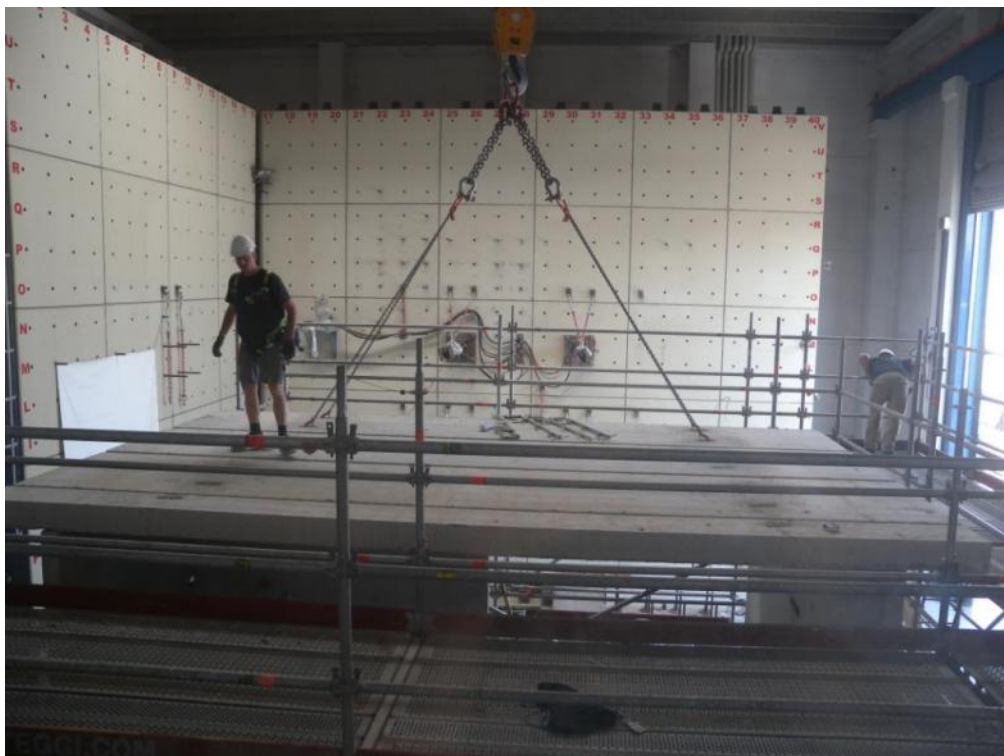
Figure 141. Crane-induced uplift and installation of precast slab panels – Second-storey floor.
