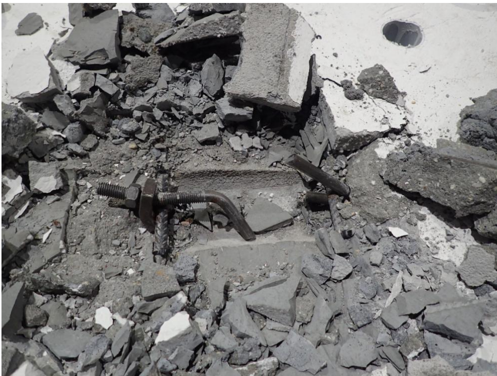
Figure 76. Failure mechanism of the steel connector at the end of the test (after cutting and removal of grout).
