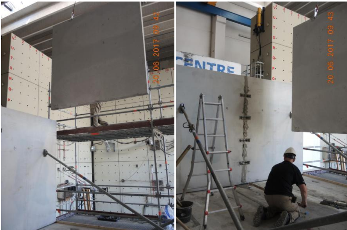
Figure 137. Uplift and transportation of the second-storey stability wall.
