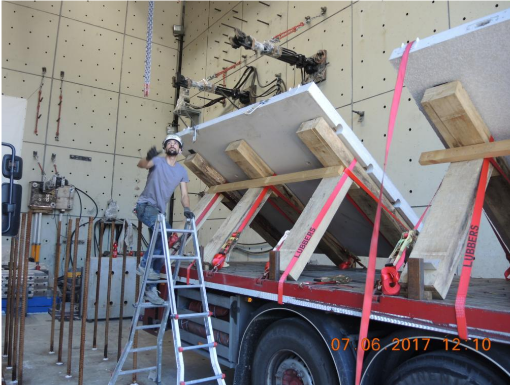
Figure 100. Uplift of a precast wall-element by means of cranes and lifting hooks.
