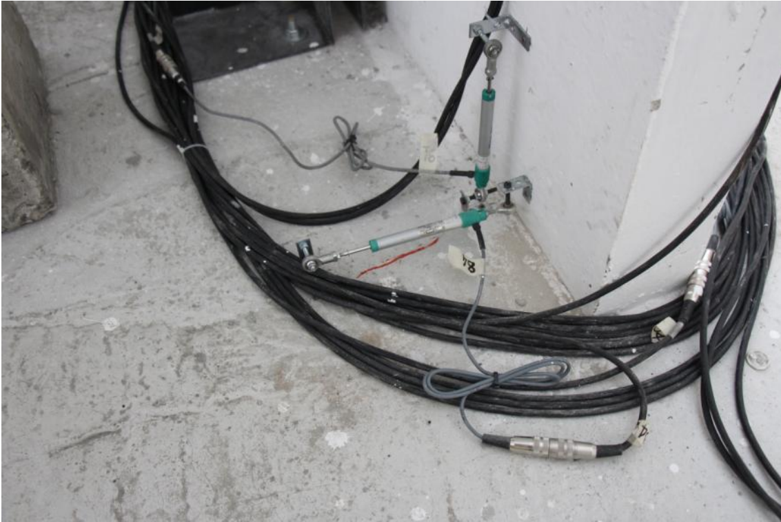
Figure 262. Minor cracks in the concrete topping close to the North edge of the second-storey stability wall.
