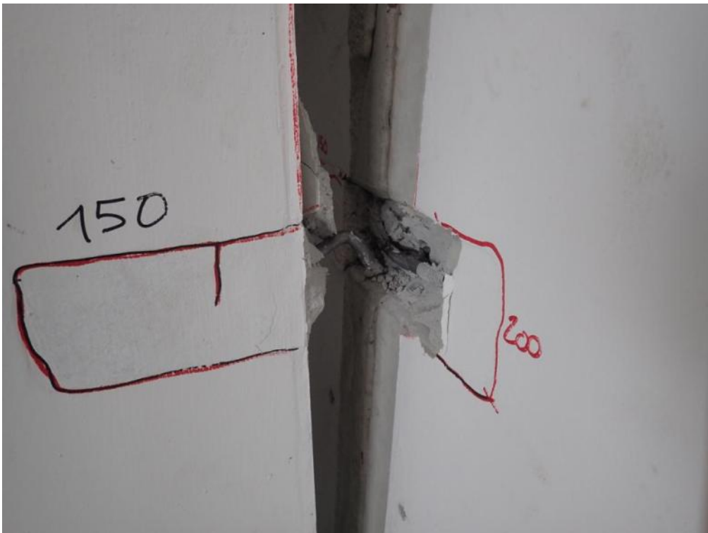
Figure 546. Permanently-bent steel hooks in lateral and stability walls – Third panel joint from the base.
