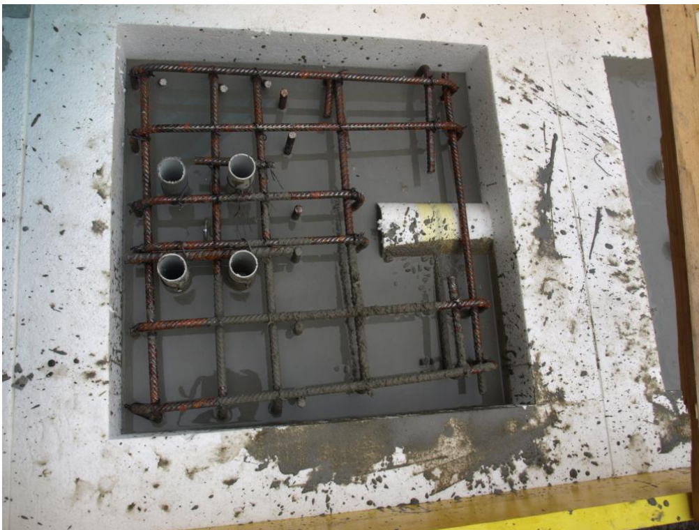
Figure 60. Casting of concrete – Vertical panel (featuring characteristics of the stability walls).
