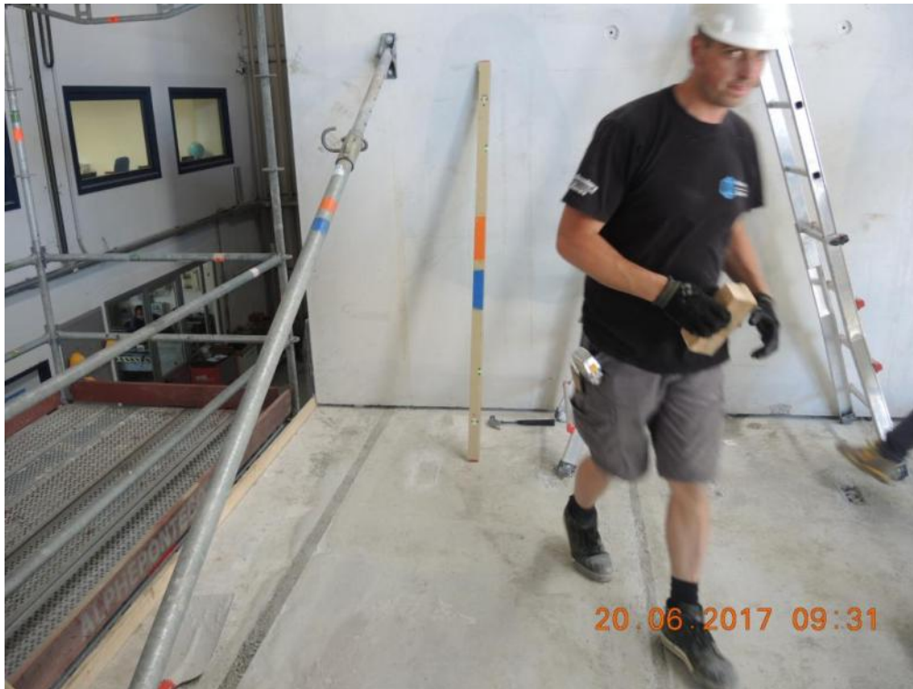
Figure 132. Temporary props for the second-storey walls – Anchorage to precast wall panels.
