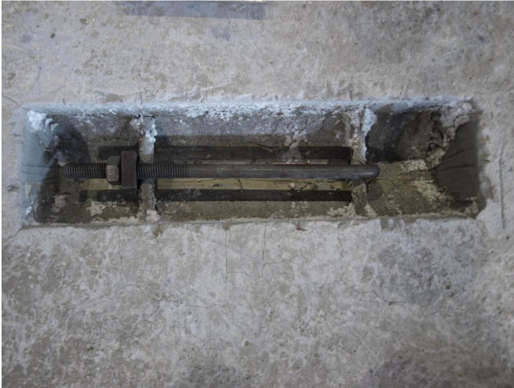
Figure 67. Lodgement of the steel connector in one horizontal panel.
