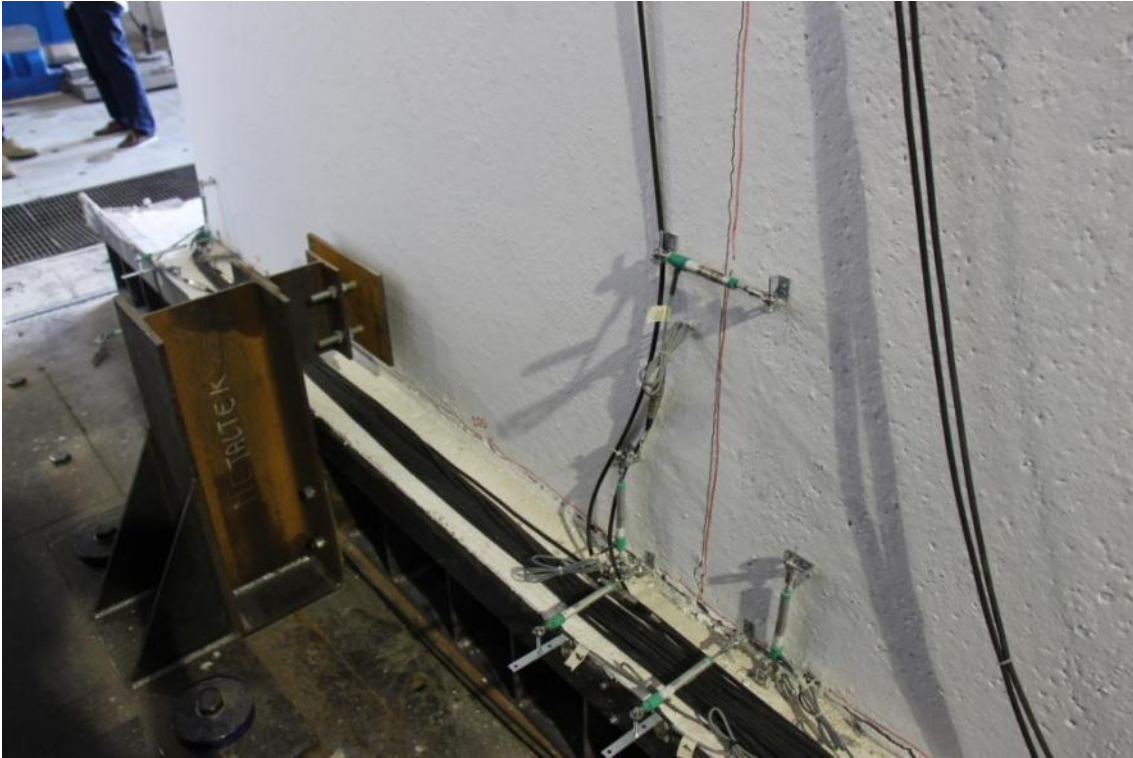
Figure 300. Damage pattern at the base of the South-sided ground-floor lateral walls.
