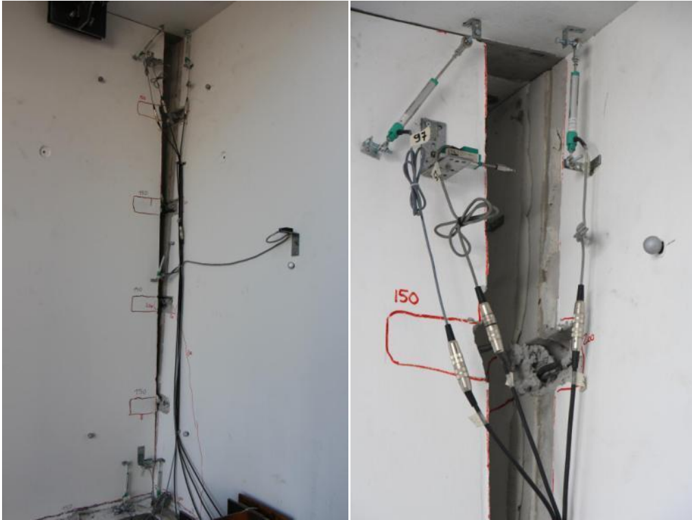
Figure 324. Failure mechanism of three-way panel connections – Detail of permanently-bent steel connectors.
