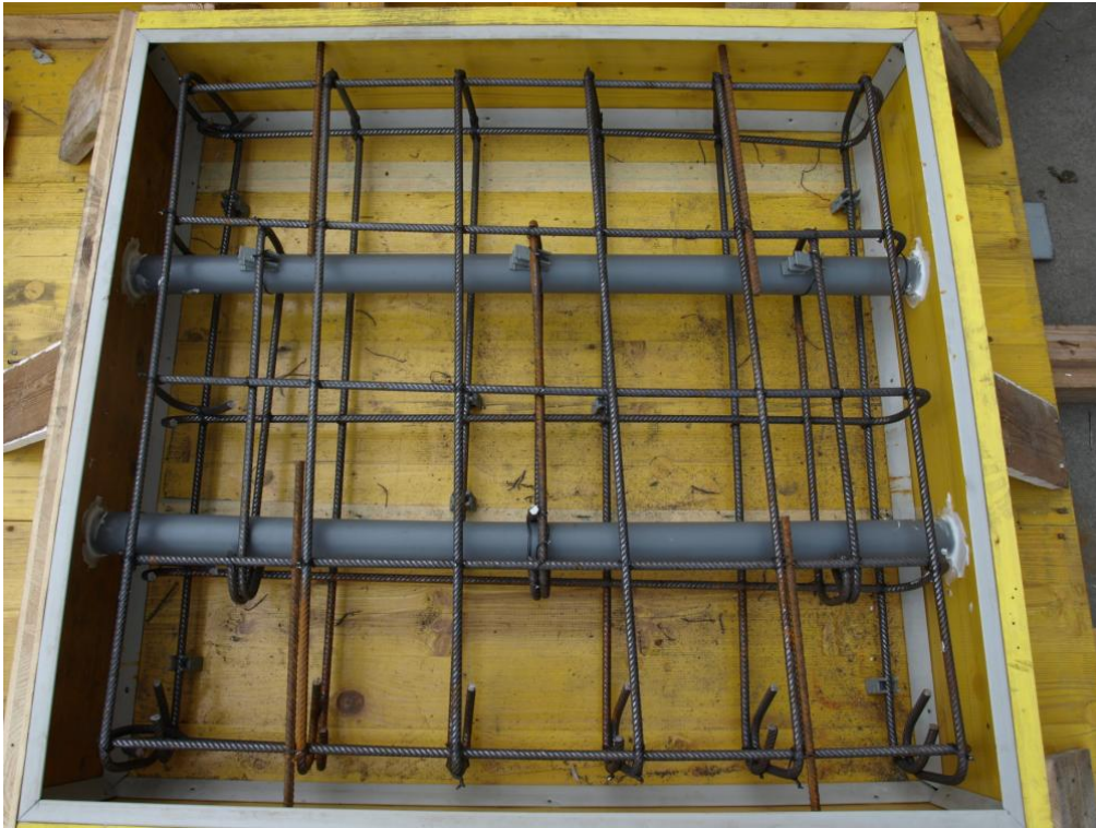
Figure 27. Top view of longitudinal and transversal reinforcing rebars.
