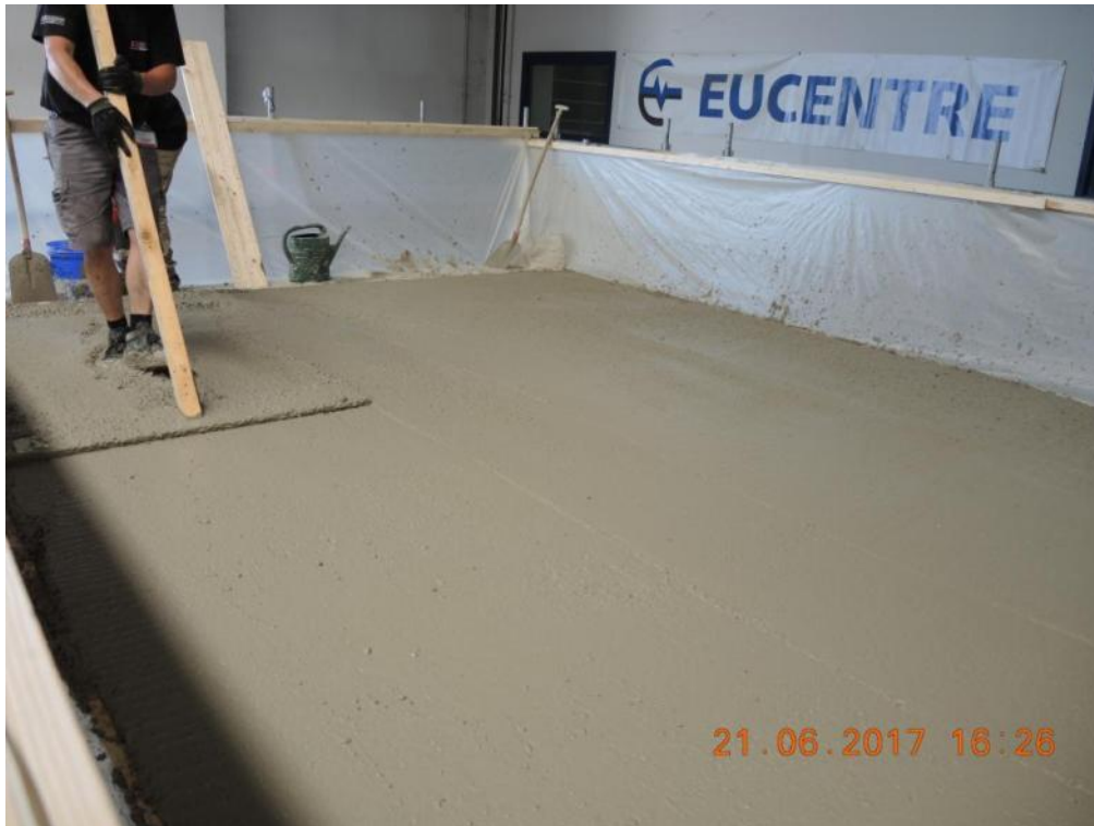
Figure 150. Casting of concrete slab topping – Second storey, levelling and finishing.
