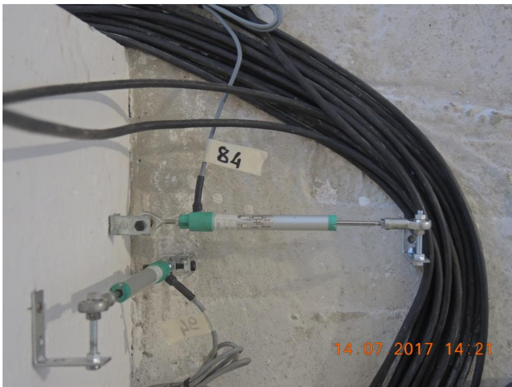
Figure 222. Instrumentation at the base of the second-storey stability wall.
