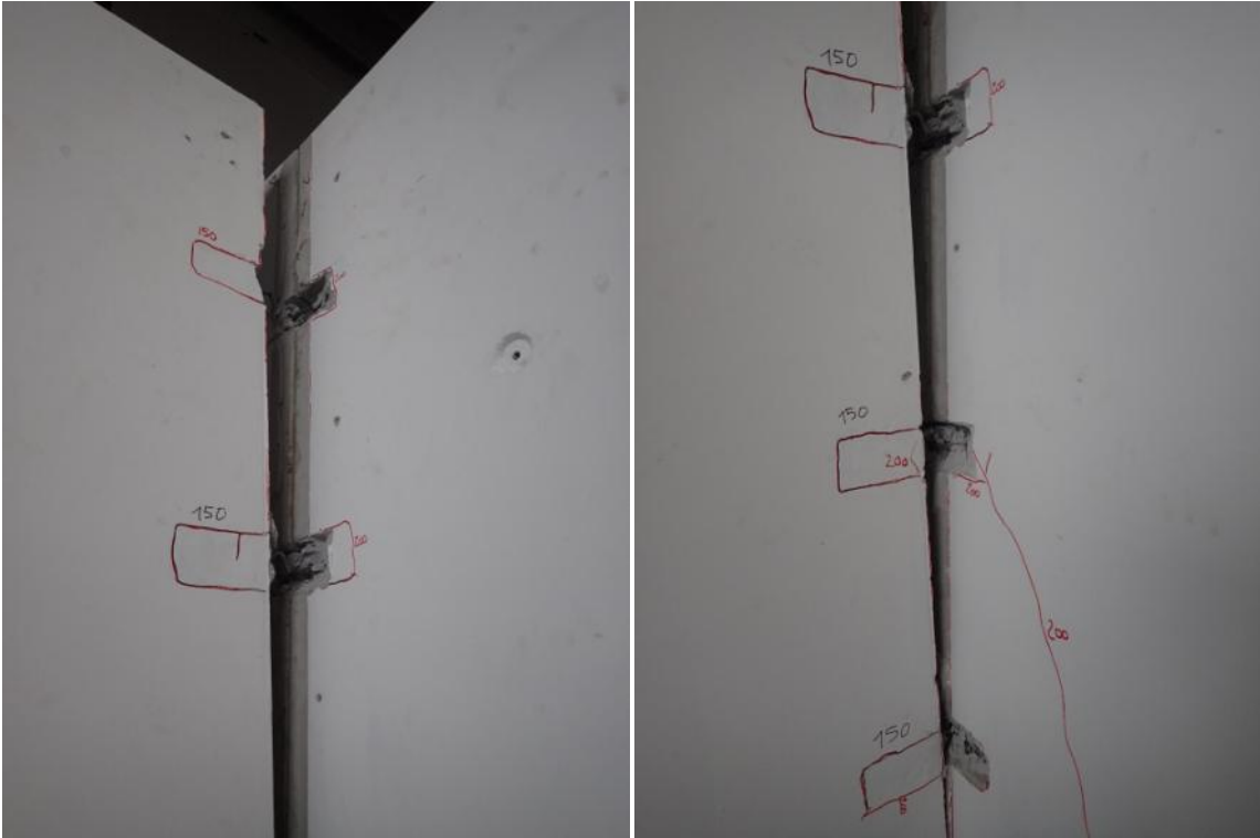
Figure 543. Permanently-bent steel connectors embedded in the stability wall – West-side view.
