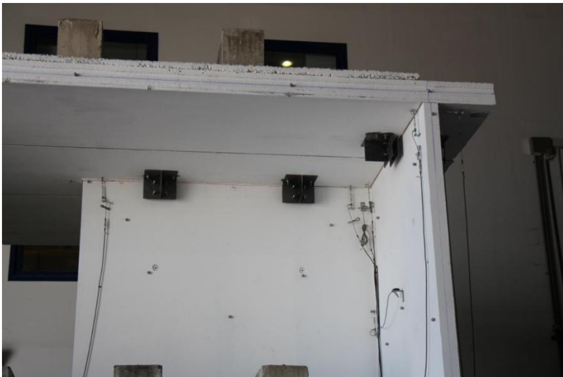
Figure 319. Accumulation of permanent displacements at the second storey of the test specimen.
