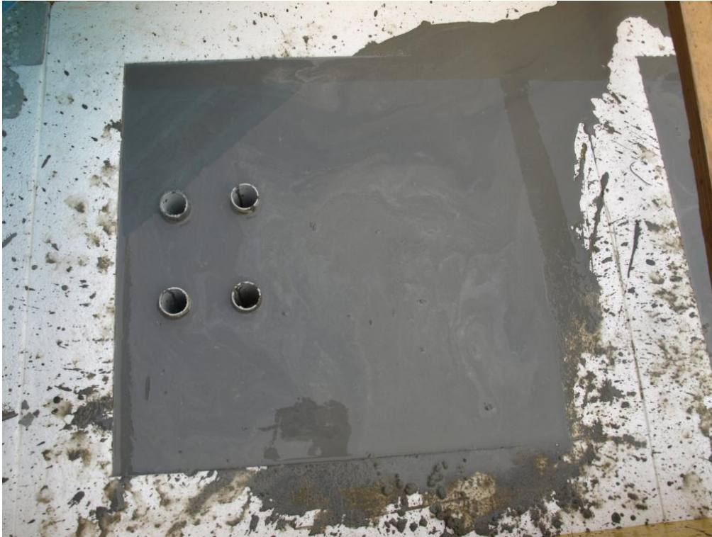
Figure 61. Detail of one vertical panel after casting of concrete.
