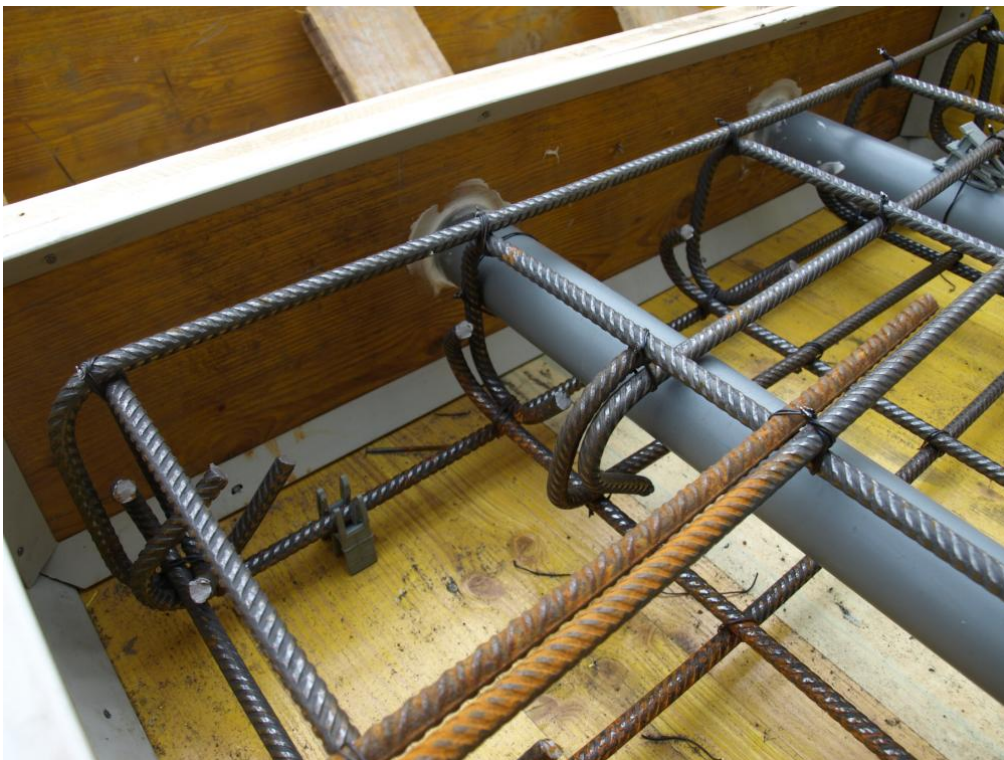
Figure 28. Enlarged view of longitudinal and transversal reinforcing rebars.
