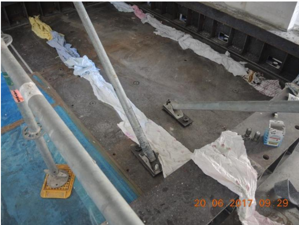
Figure 119. Key details – Installation of temporary diagonal steel members on the shake-table of the laboratory.
