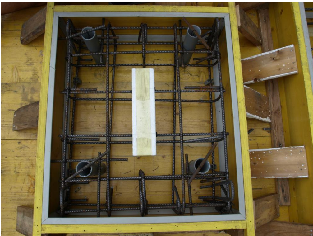
Figure 54. Arrangement of reinforcing rebars in one of the wall stripes.
