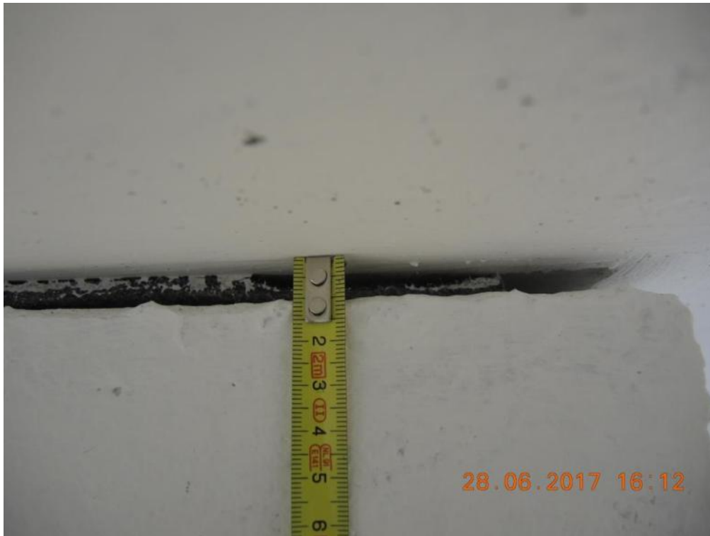
Figure 155. Gap between the stability wall and slab panel of EUC-BUILD5 specimen – Opposite wall face.
