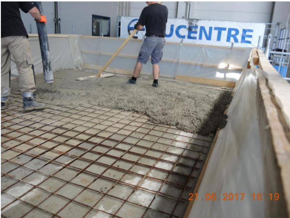
Figure 149. Casting of concrete slab topping – Second storey, levelling.
