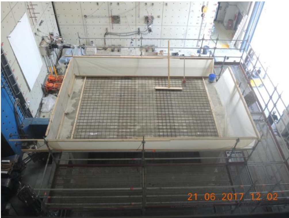
Figure 145. Arrangement of steel mesh before casting of concrete topping – Second floor.
