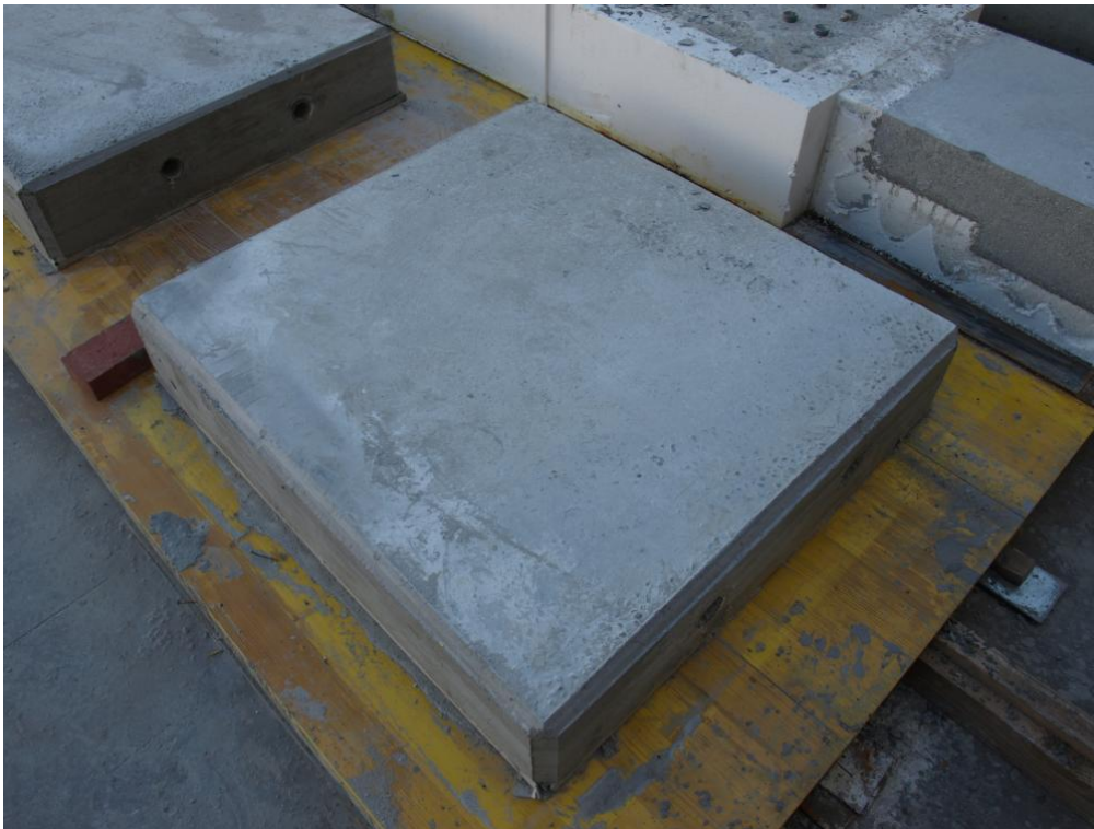
Figure 33. Detail of a concrete block after removal of the formwork.
