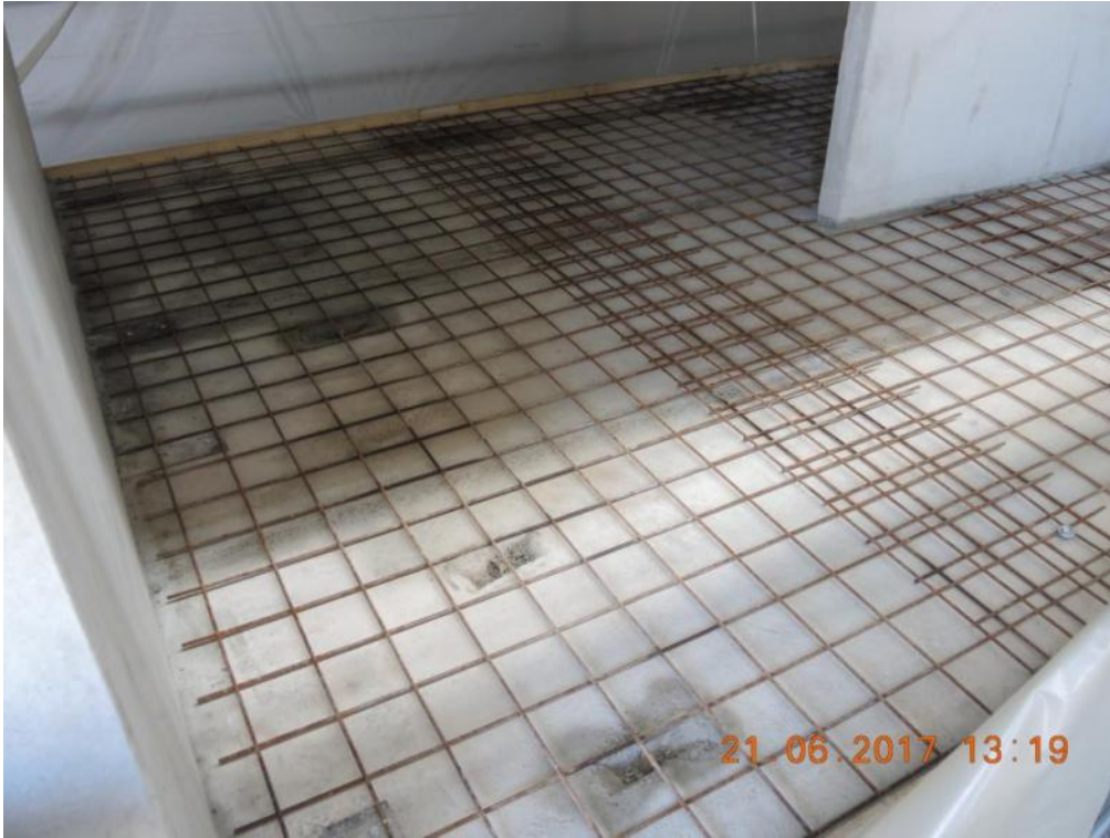
Figure 146. Arrangement of steel mesh before casting of concrete topping – First floor.
