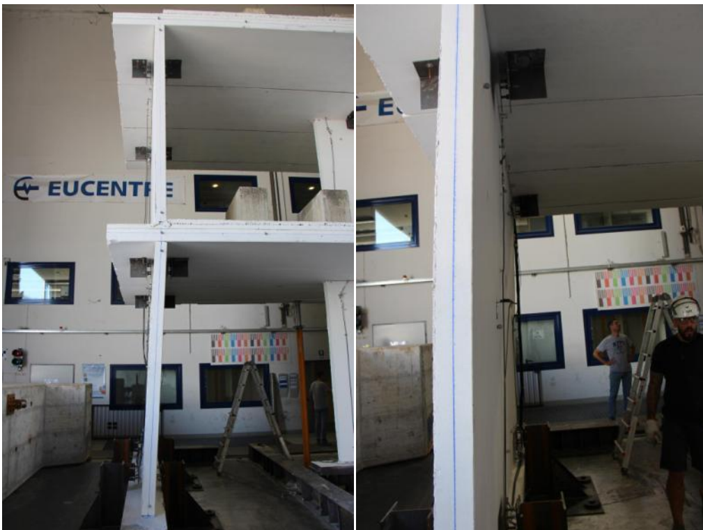
Figure 327. Overall and detailed views of the North-sided transversal walls at the end of testing.
