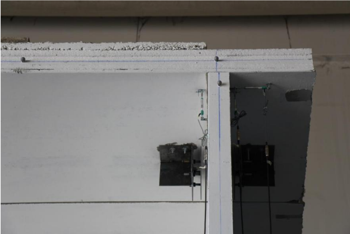
Figure 336. Sliding of second-storey slab on the precast wall – South side of the specimen.
