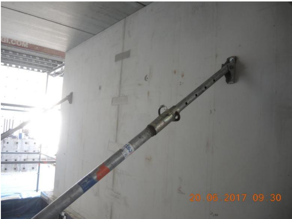
Figure 129. Detail of the installed temporary props – Anchorage to precast wall panels.
