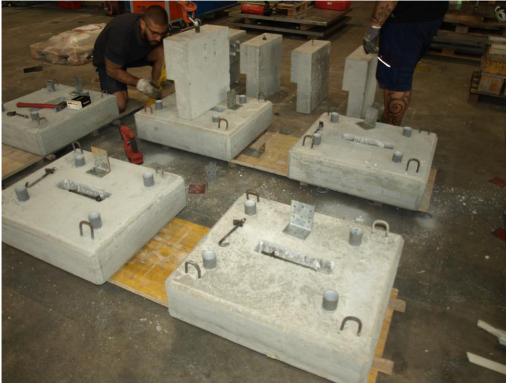
Figure 65. Assembling of the specimens – Uplift of vertical panel.
