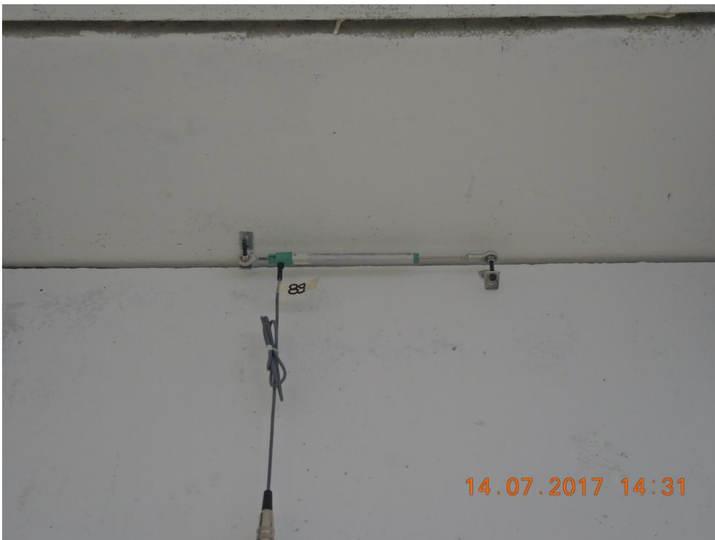
Figure 224. Potentiometer installed between precast wall and slab panels.
