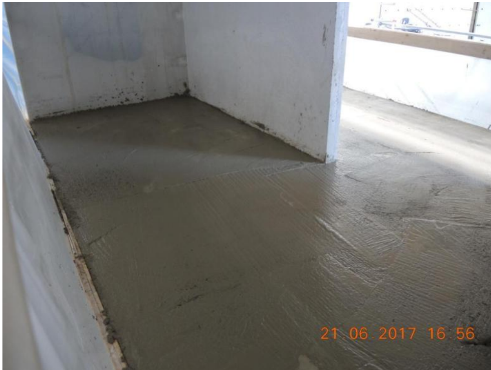
Figure 152. Casting of concrete slab topping – First storey after levelling and finishing.
