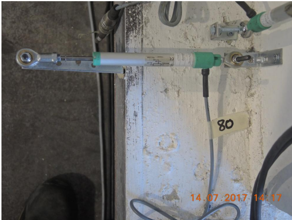
Figure 221. Instrumentation at the base of a first-storey transversal wall.
