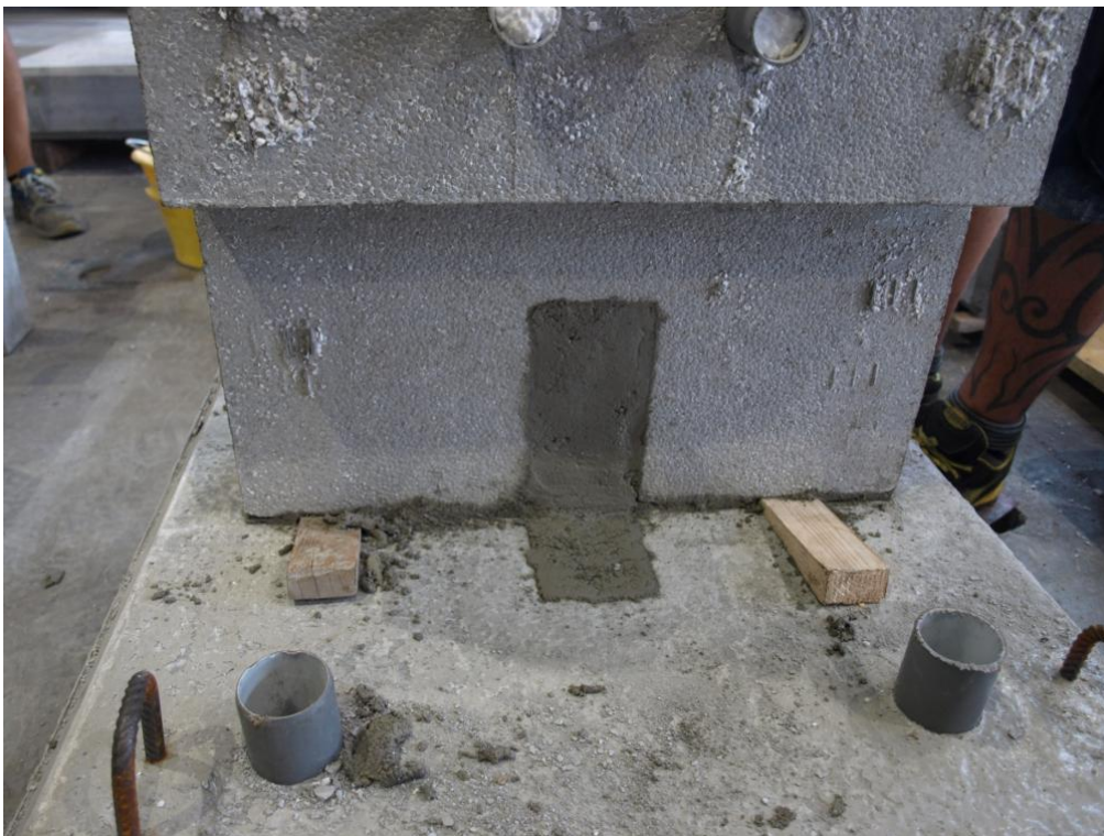
Figure 68. Detail of wood spacers and mortar grout in the connector socket.
