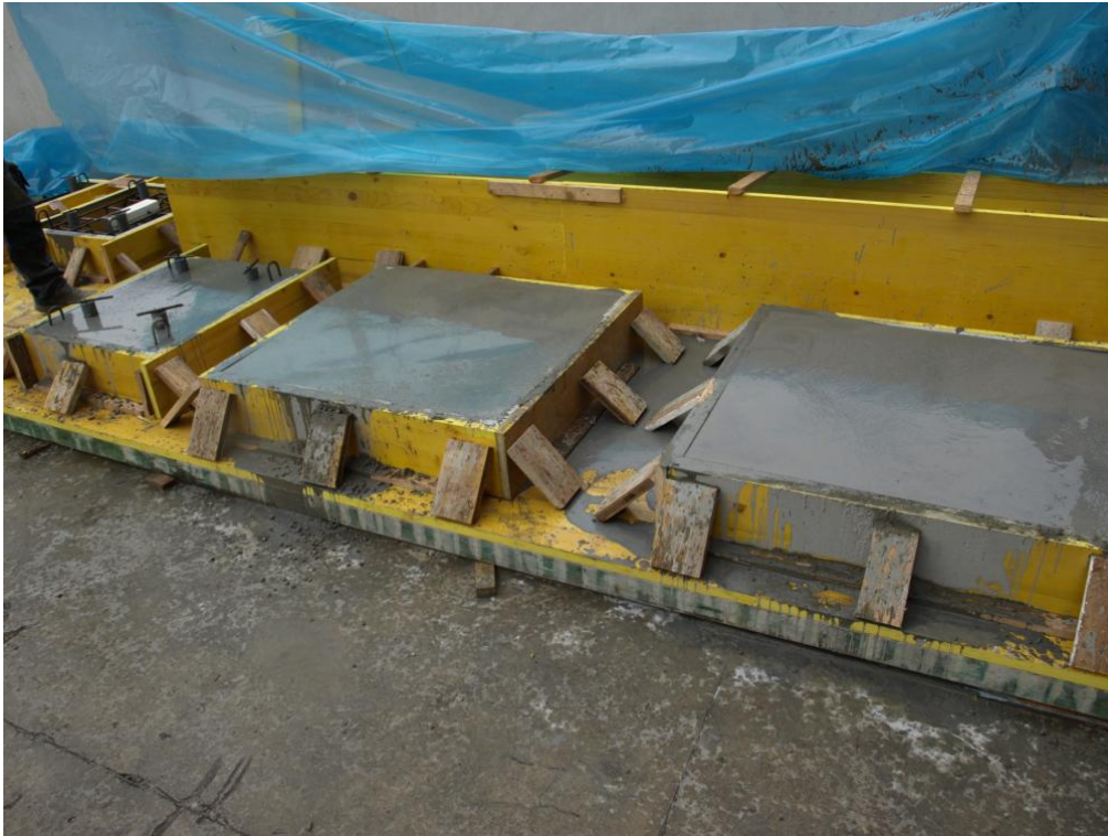
Figure 31. Detail of concrete blocks after casting.
