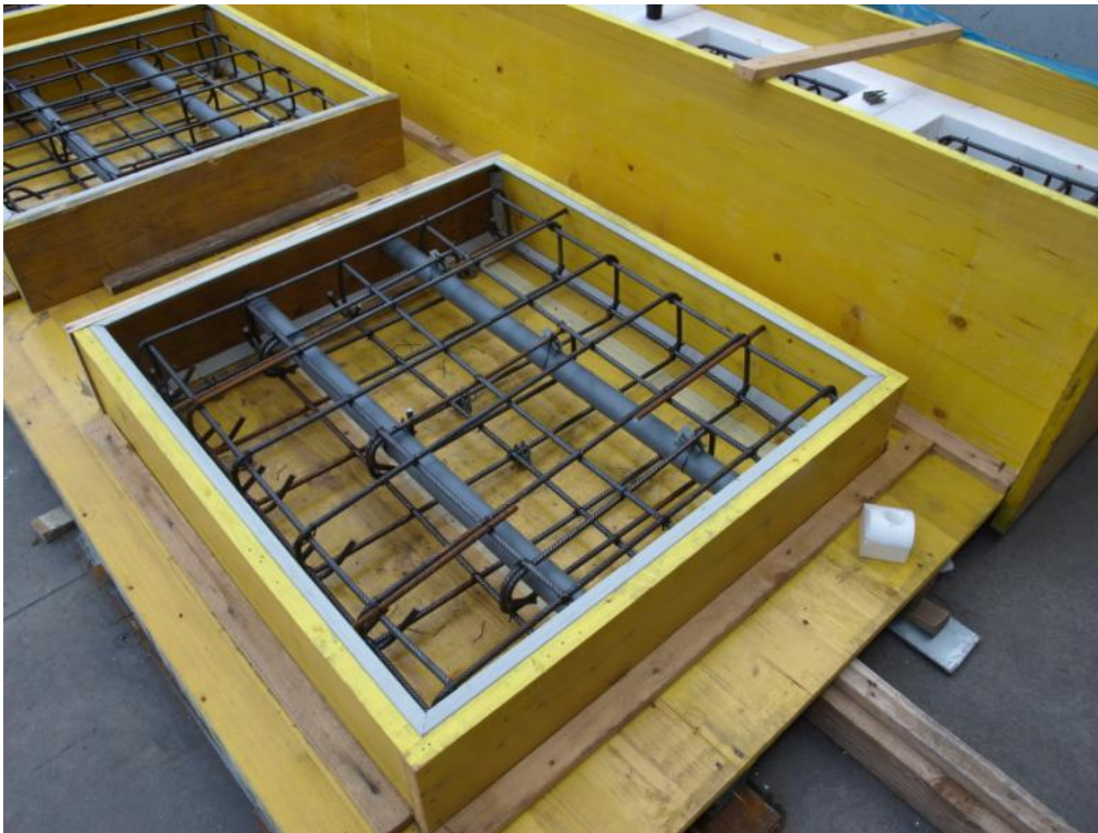
Figure 25. Details of the formworks and reinforcement arrangement.
