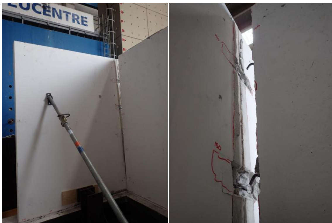
Figure 541. Diagonal props for lateral stability and detail of the damage state of steel connectors.
