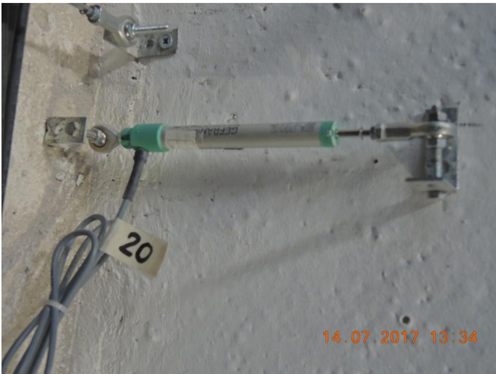
Figure 216. Potentiometers at the base of the lateral walls – Centre.
