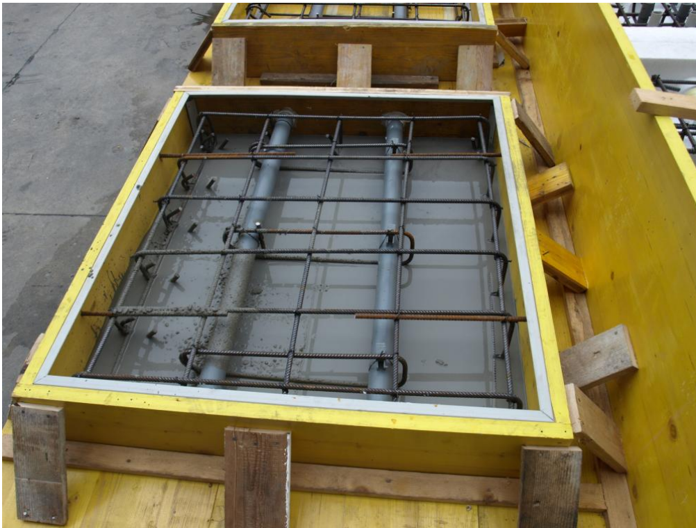
Figure 29. Casting of concrete blocks – Detail 1.
