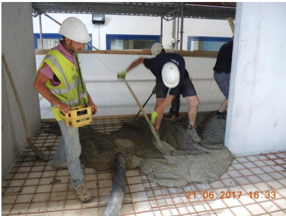
Figure 151. Casting of concrete slab topping – First storey, levelling.
