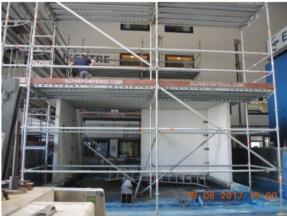
Figure 127. Overall view of the erected first-storey of EUC-BUILD5 specimen.
