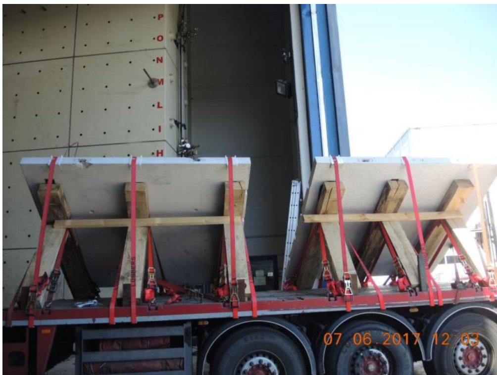
Figure 99. Delivery of precast wall panels.
