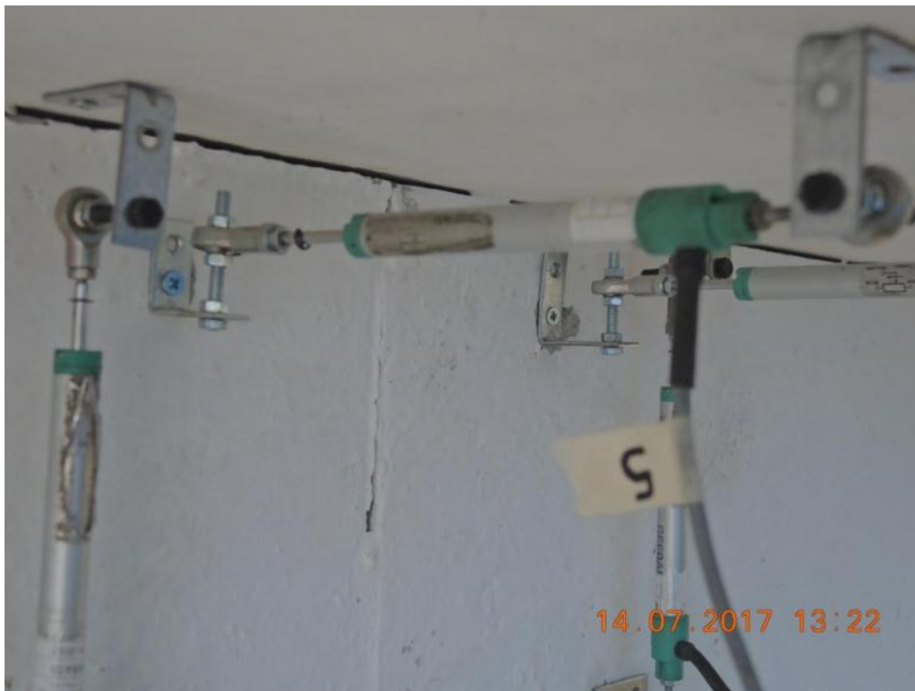
Figure 206. Potentiometer at the top of the South-West-sided lateral wall – South wall face, East corner.
