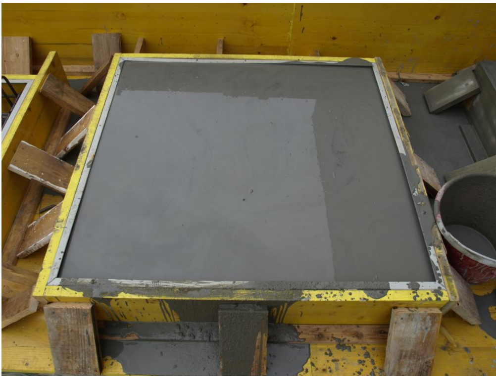
Figure 30. Casting of concrete blocks – Detail 2.
