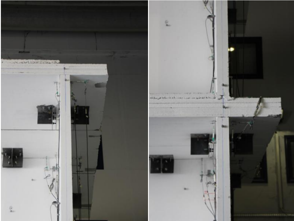
Figure 308. Sliding and accumulation of displacement residuals – Second-storey floor slab, South side.
