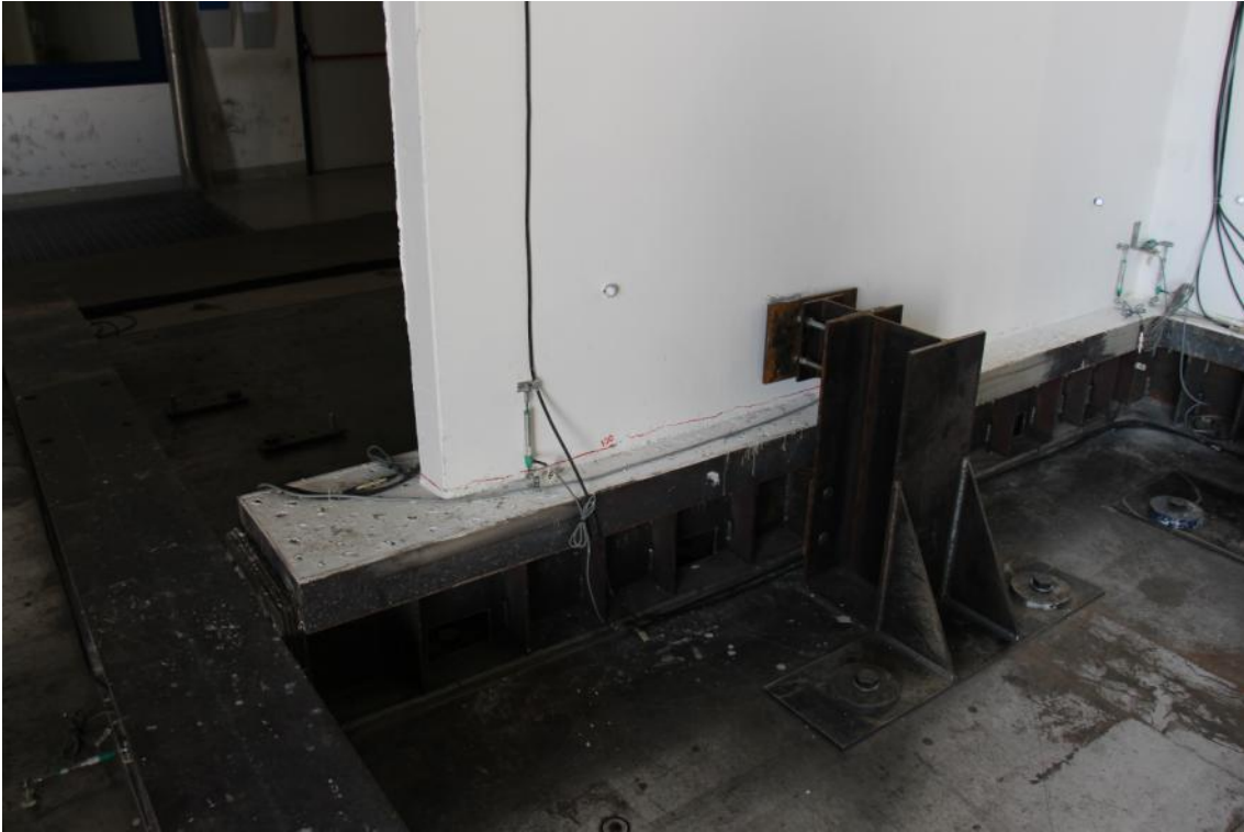
Figure 256. Development of cracks at the base of the ground-floor stability wall.
