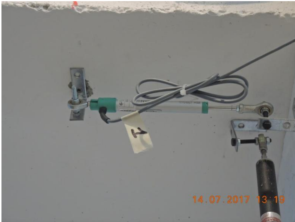
Figure 203. Potentiometer at the top of the South-East-sided lateral wall – South wall face, East corner.
