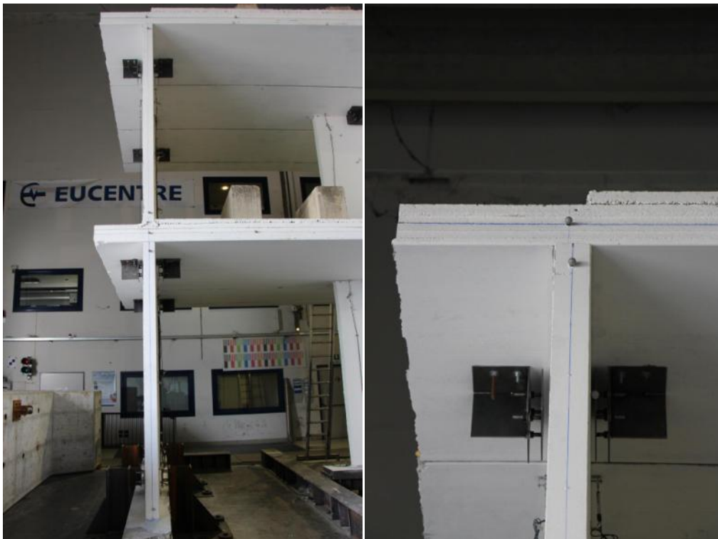
Figure 307. Sliding and accumulation of displacement residuals – Second-storey floor slab, North side.
