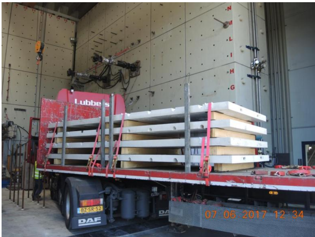
Figure 103. Detail of the static scheme adopted to store lateral wall panels on truck for transportation.
