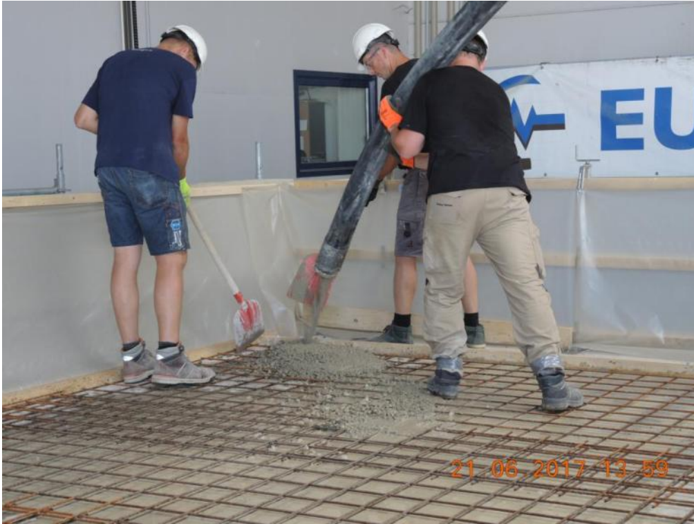
Figure 148. Casting of concrete slab topping – Second storey.
