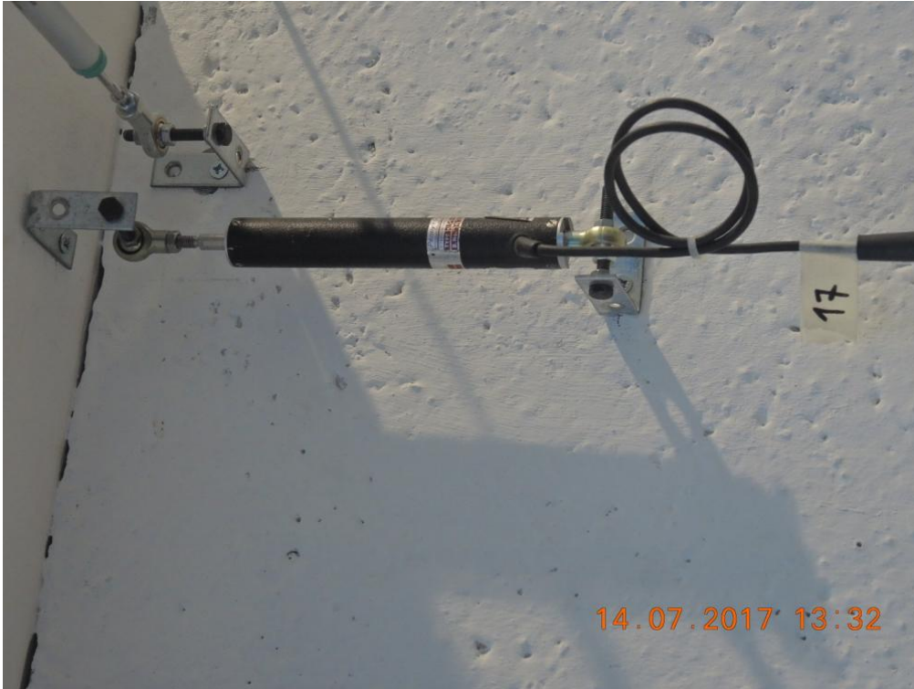
Figure 213. Potentiometers installed onto the top of the lateral walls – First storey.
