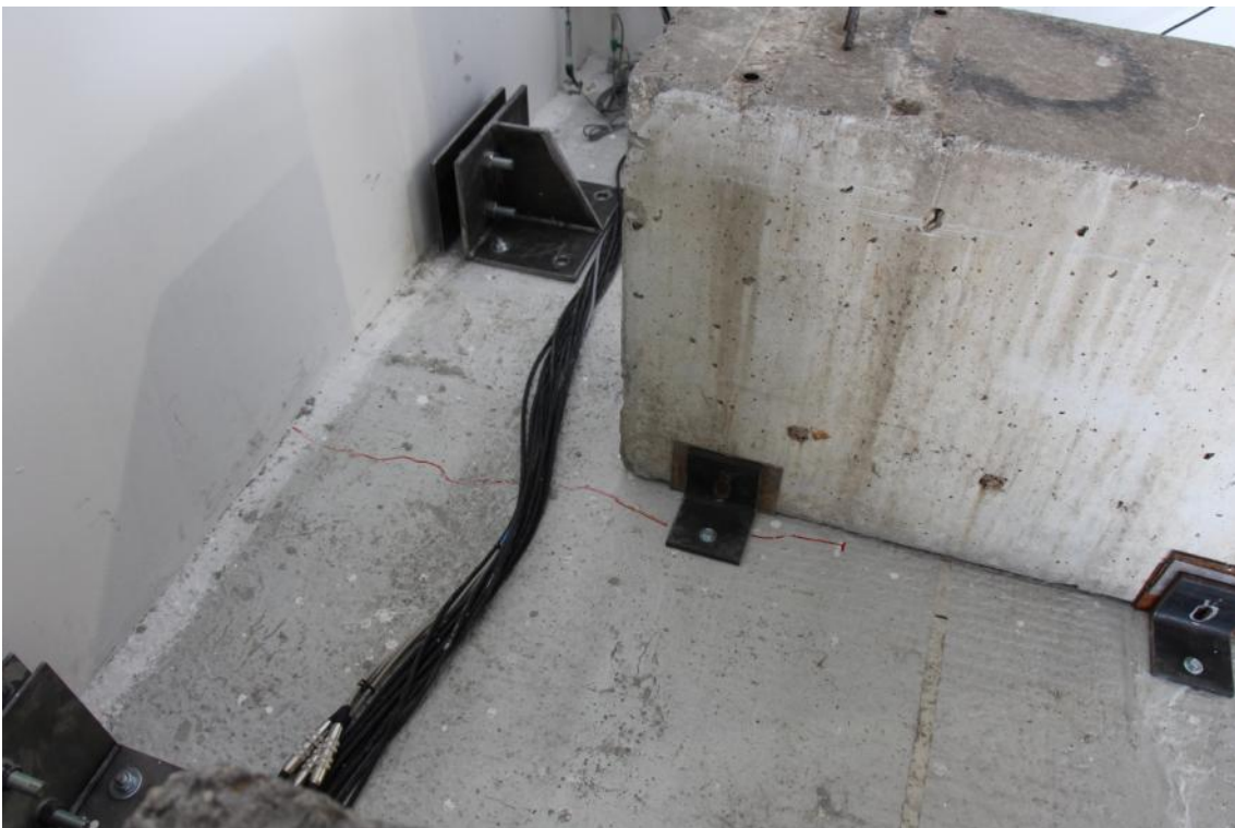
Figure 263. Crack running from the centre of the second-storey stability wall – West wall face.
