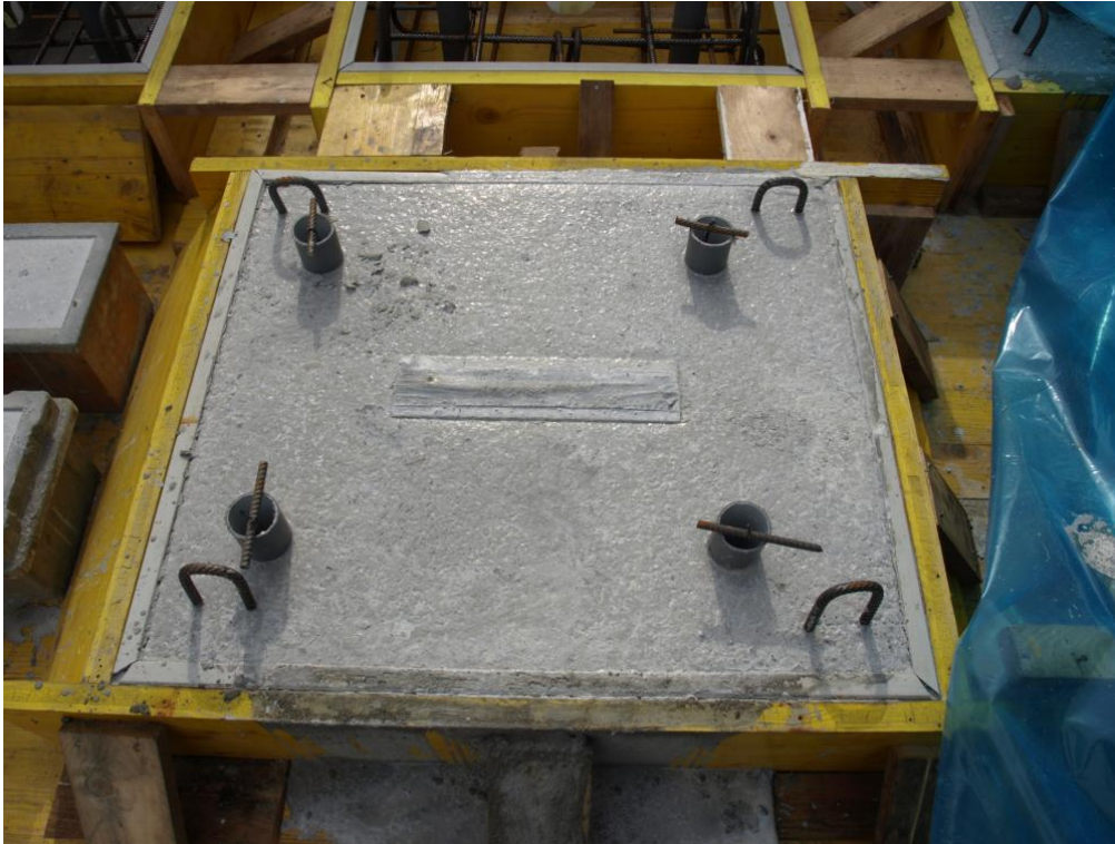
Figure 59. Detail of one horizontal panel after casting of concrete.
