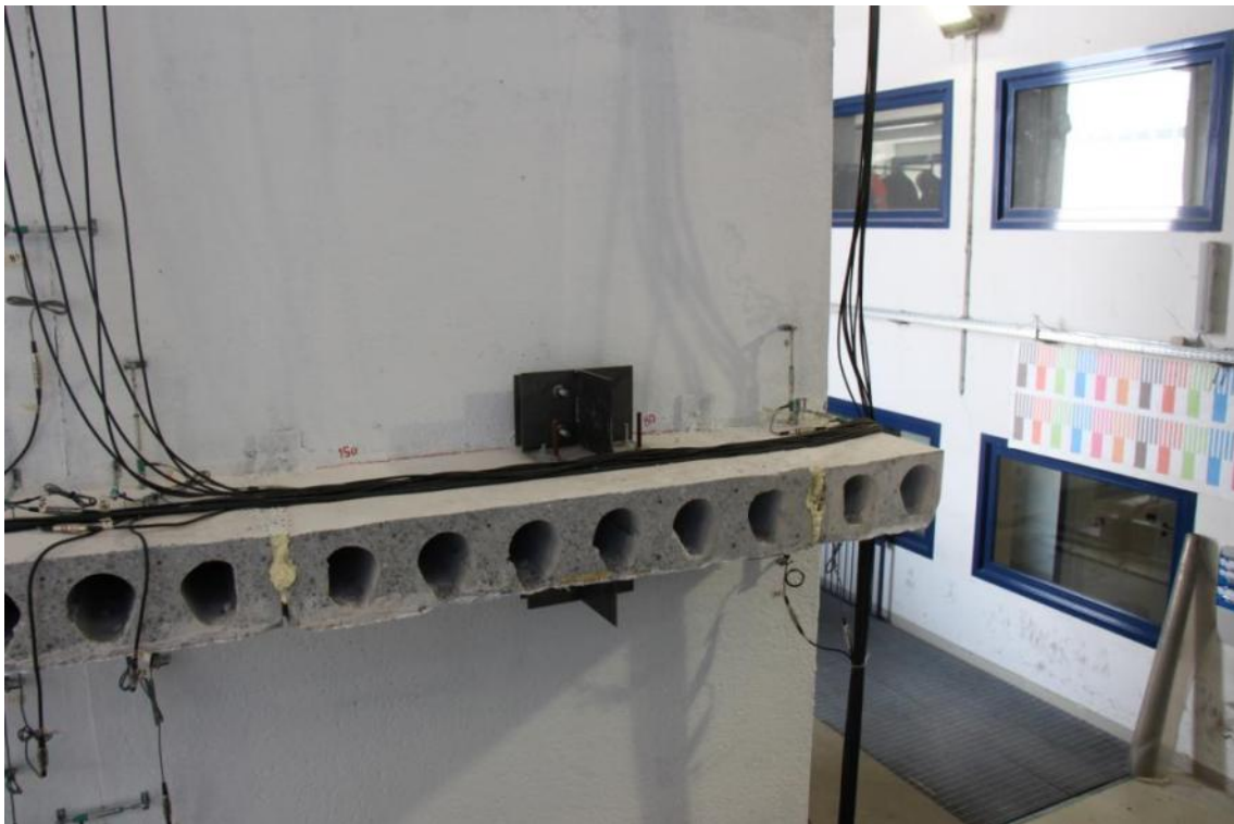
Figure 285. Development of horizontal flexural cracks at the base of panel 2L1 – Second-storey lateral wall.
