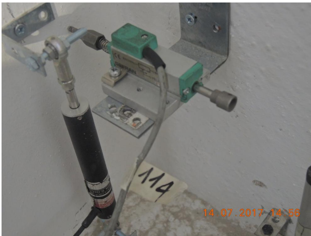
Figure 226. Instrumentation installed on a stability wall – Out-of-plane displacement monitoring.
