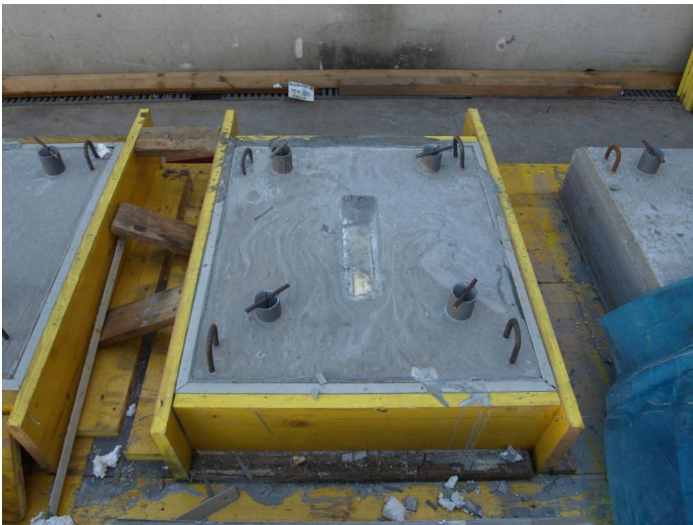
Figure 62. Detail of one horizontal panel before removal of the formworks.
