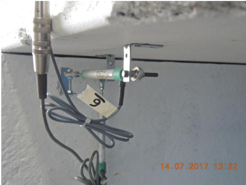
Figure 207. Potentiometer at the top of the South-West-sided lateral wall – South wall face, West corner.
