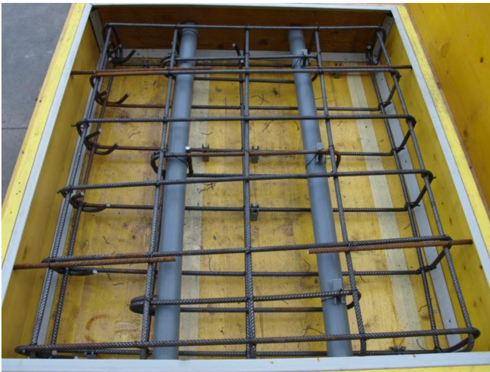
Figure 26. Arrangement of steel rebars and plastic tubes.
