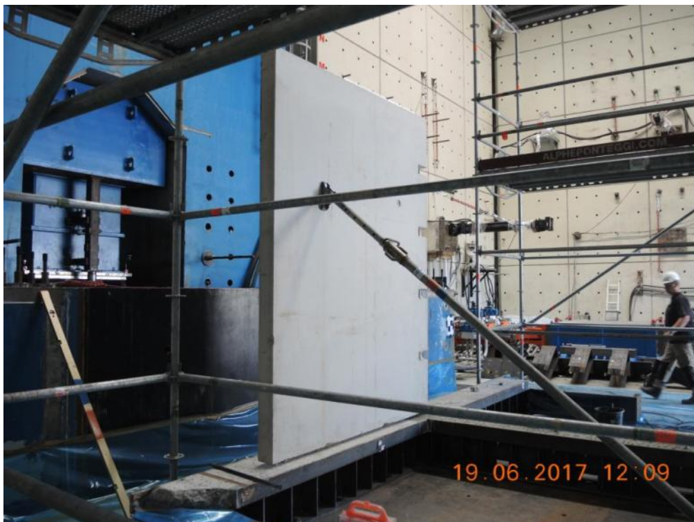
Figure 121. Erection of the first-storey South-East-sided lateral wall on the steel foundation.
