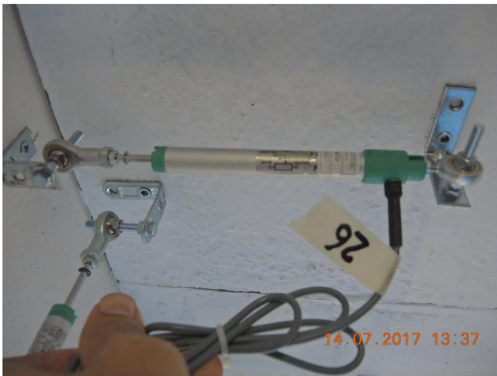
Figure 218. Detail of a potentiometer installed at the top of lateral walls – Opposite side.
