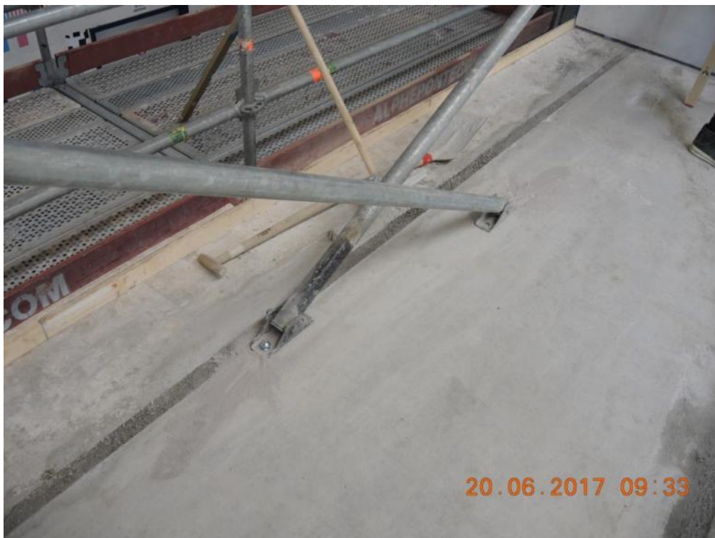
Figure 133. Temporary props for the second-storey walls – Anchorage to precast slab panels.
