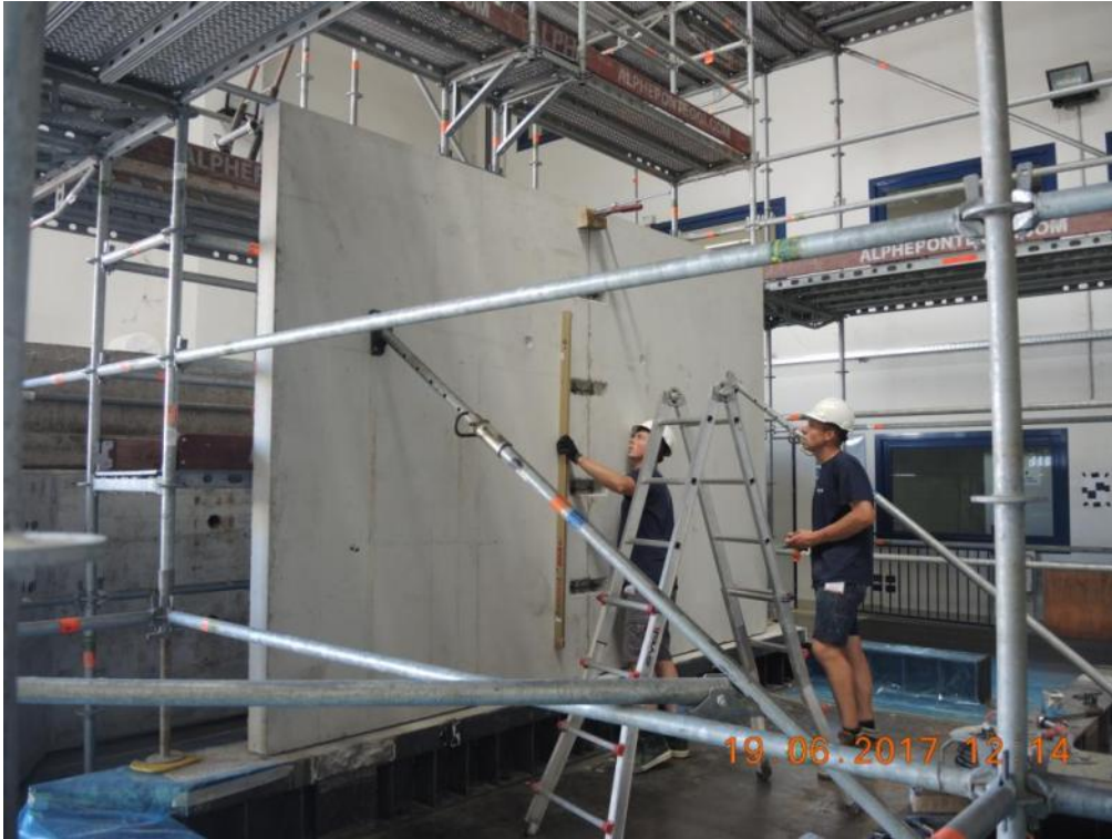
Figure 122. Erection of the first-storey North-sided lateral walls on the steel foundation.
