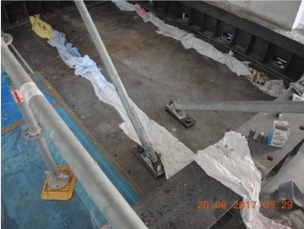
Figure 128. Detail of the installed temporary props – Anchorage to shake-table.
