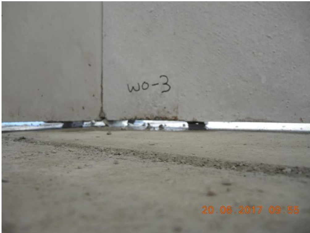
Figure 140. Detail of spacers beneath second-storey precast wall panels.
