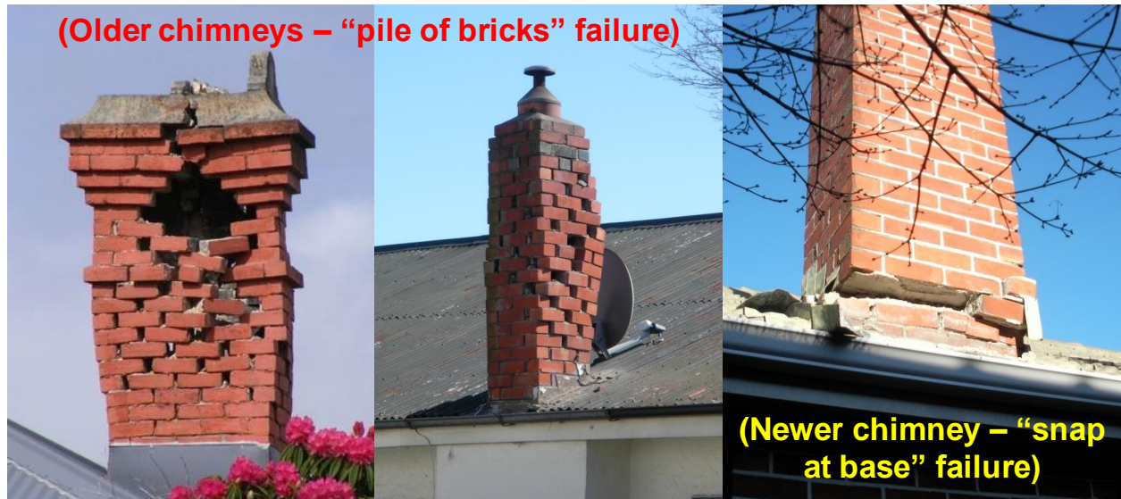
Figure A2.31: Failure Mechanisms for Chimneys
