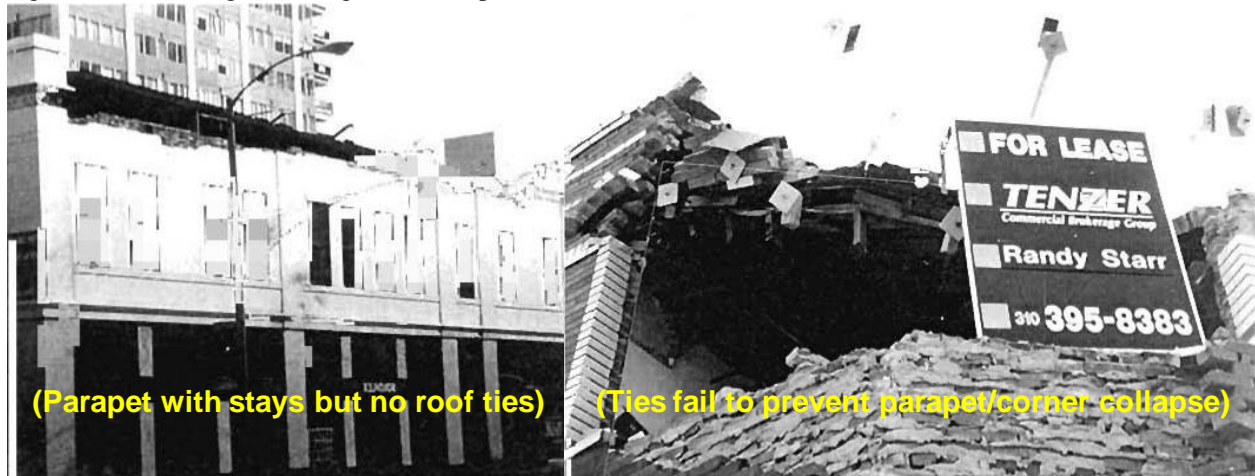
Figure A2.16 Damage to Strengthened Parapets
