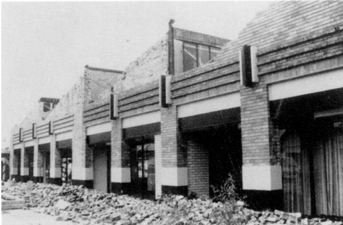
Figure A2.21 Parapet Damage example on a Modern URM Building
