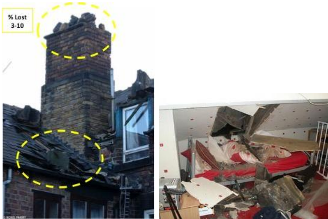
Figure A2.13 (b) Damaged chimney in South Yorkshire and the damage caused by debris inside
