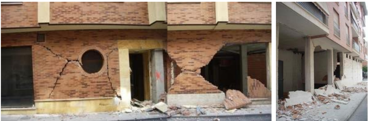
Figure A2.3 Shear Failure and Out of Plane Collapse of Infill Panels
