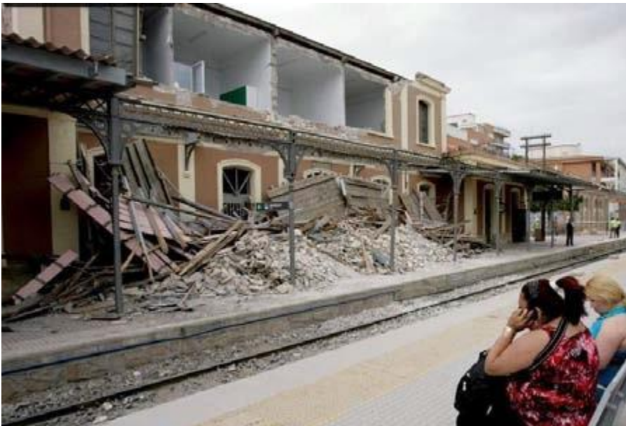
Figure A2.2 Out of Plane Masonry Wall Failure (Lorca Station)
