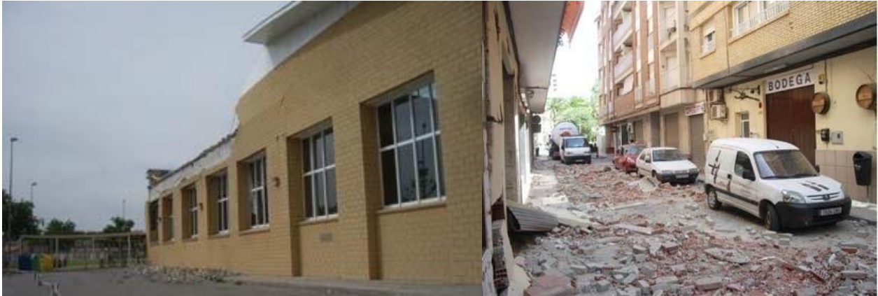
Figure A2.1 Parapet Collapse and Debris in Streets
