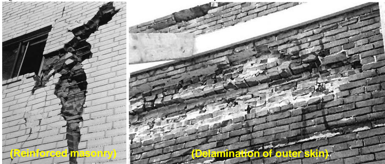
Figure A2.18 Delamination from URM and Reinforced Masonry Walls
