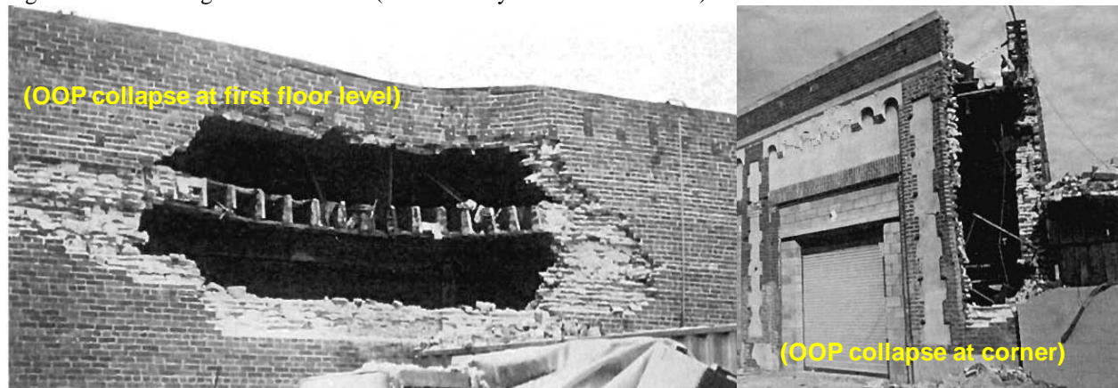
Figure A2.17 Damage to URM Walls (roof ties only – no ties at 1 st floor)
