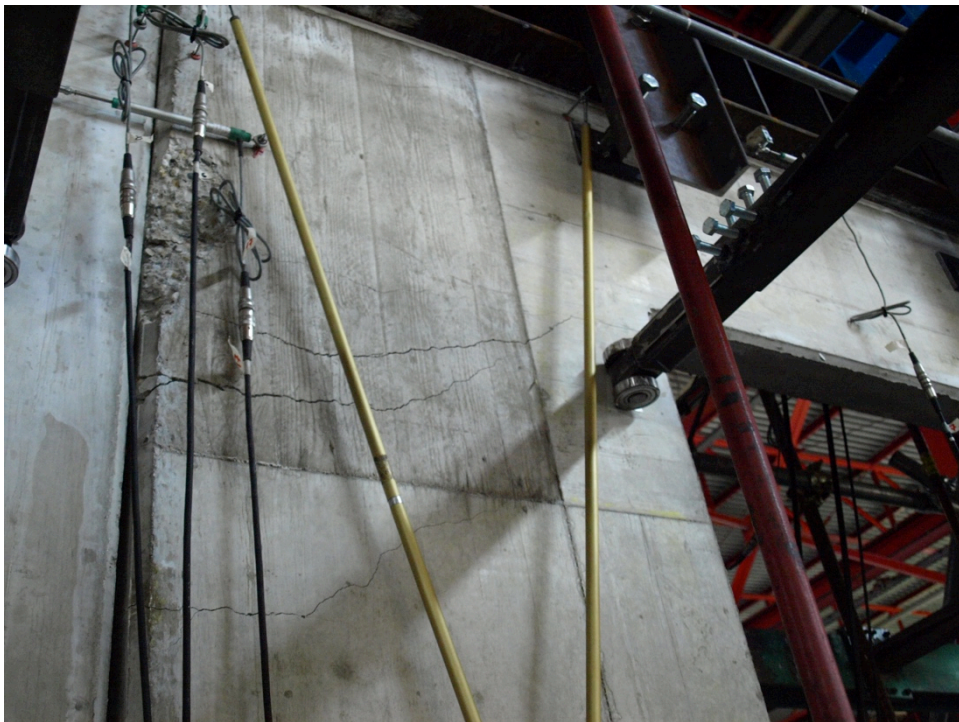
Figure 205: Pounding between the two panels of the assembly – Specimen 07
