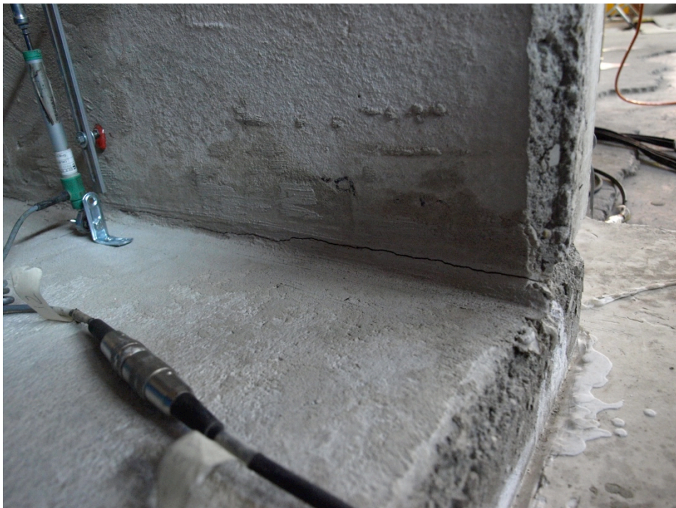
Figure 246: Detail of crack propagation along the width – Specimen 11
