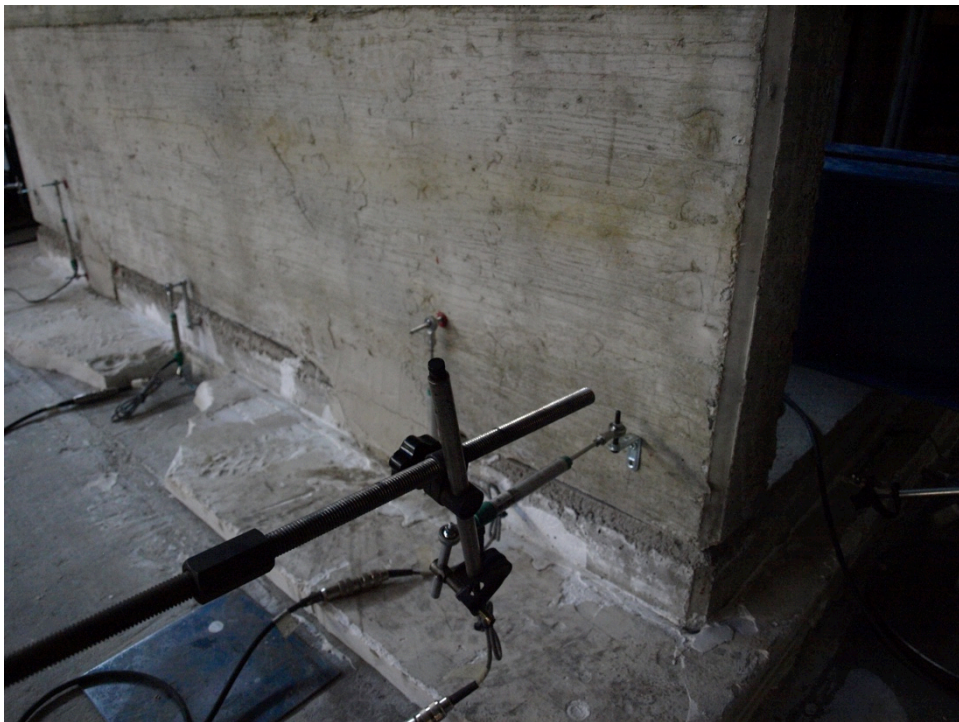
Figure 244: Lateral view of the crack at the base of panel assembly – Specimen 11
