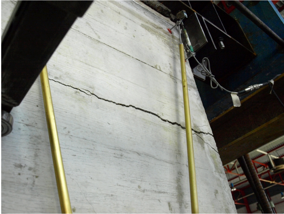
Figure 212: Horizontal cracks at the corner of the door – Specimen 08
