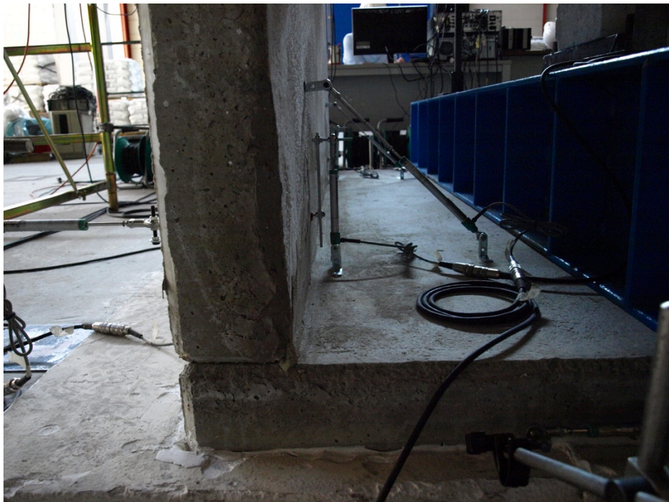
Figure 242: Side view of the damage at the connection – Specimen 11
