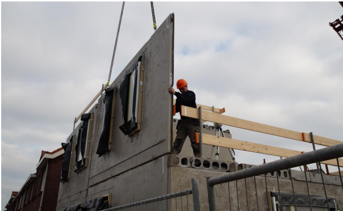
Fig.63: Heembeton construction phases
