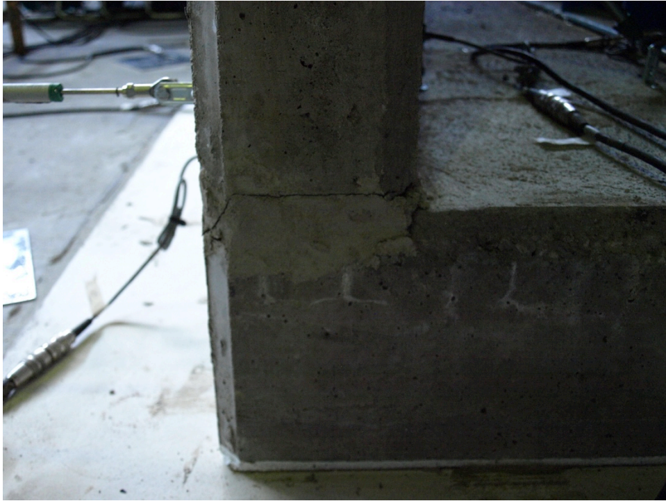
Figure 231: Damage mechanism at the connection level in Specimen 09 – detail of the crack
