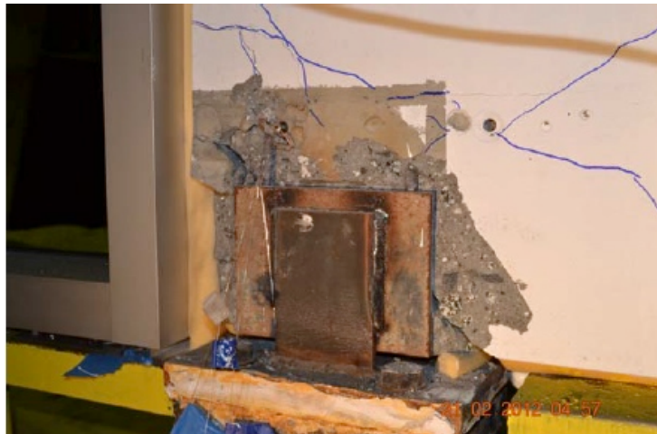
Fig. 38: Bottom connection: damage occurred at the welded steel plates
