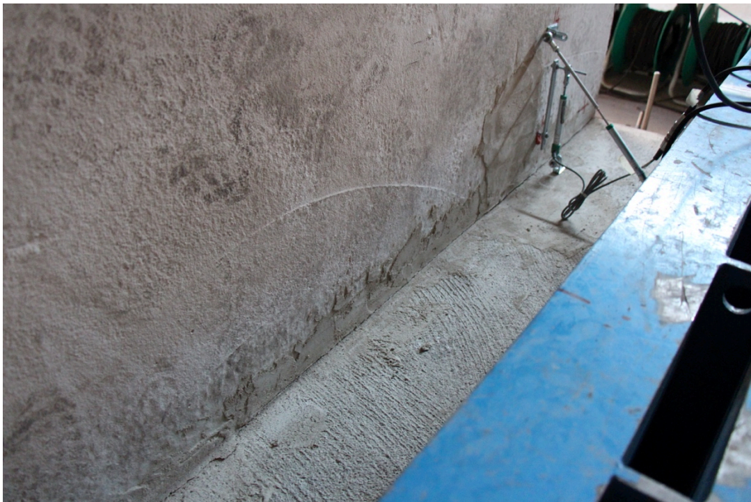
Figure 236: Propagation of the crack along the entire width – Specimen 10
