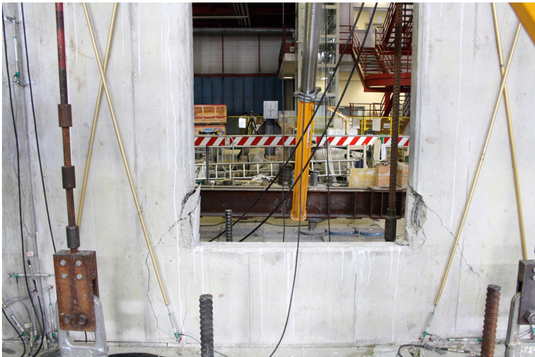
Figure 191: Cracking at the corners of the window at the end of the test – Specimen 06
