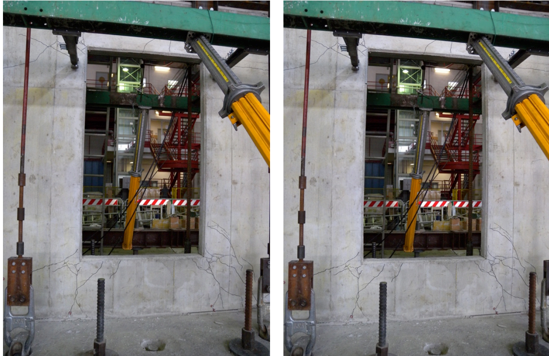
Figure 184: Crack pattern at the corners of the window – Specimen 05
