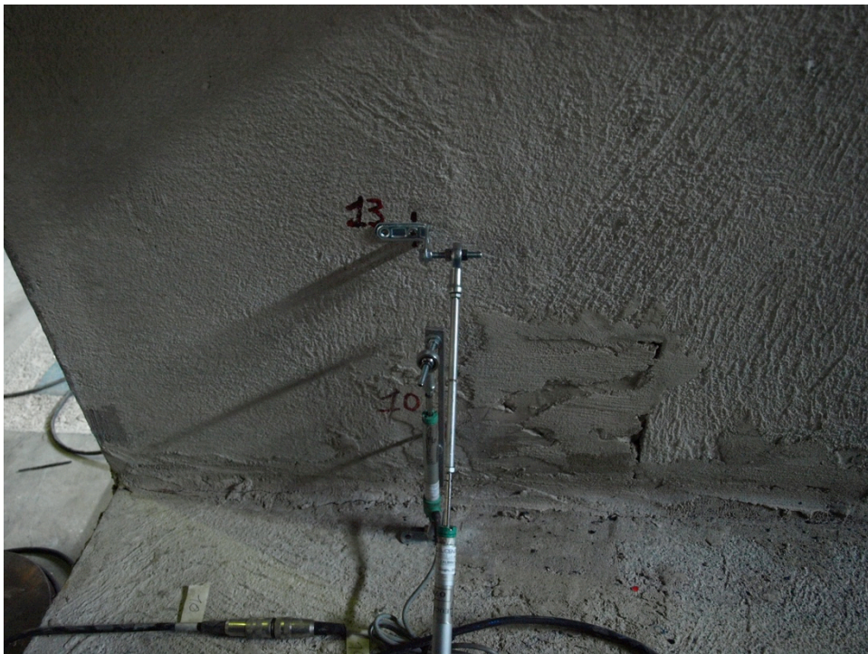
Figure 232: Detail of the mortar at the steel anchor location – Specimen 09
