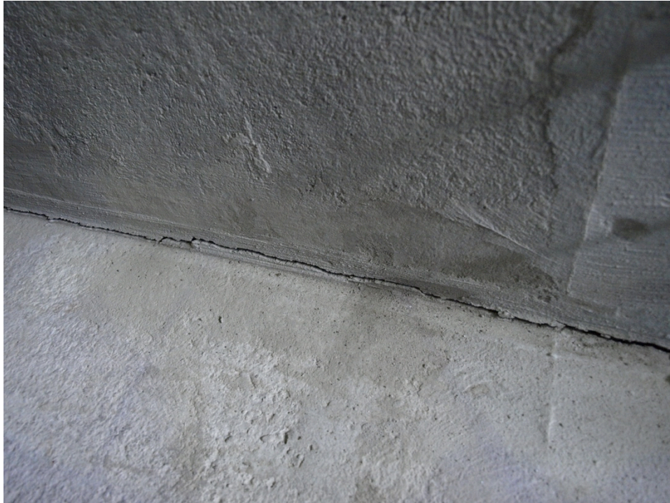
Figure 255: Detail of crack propagation along the width – Specimen 12
