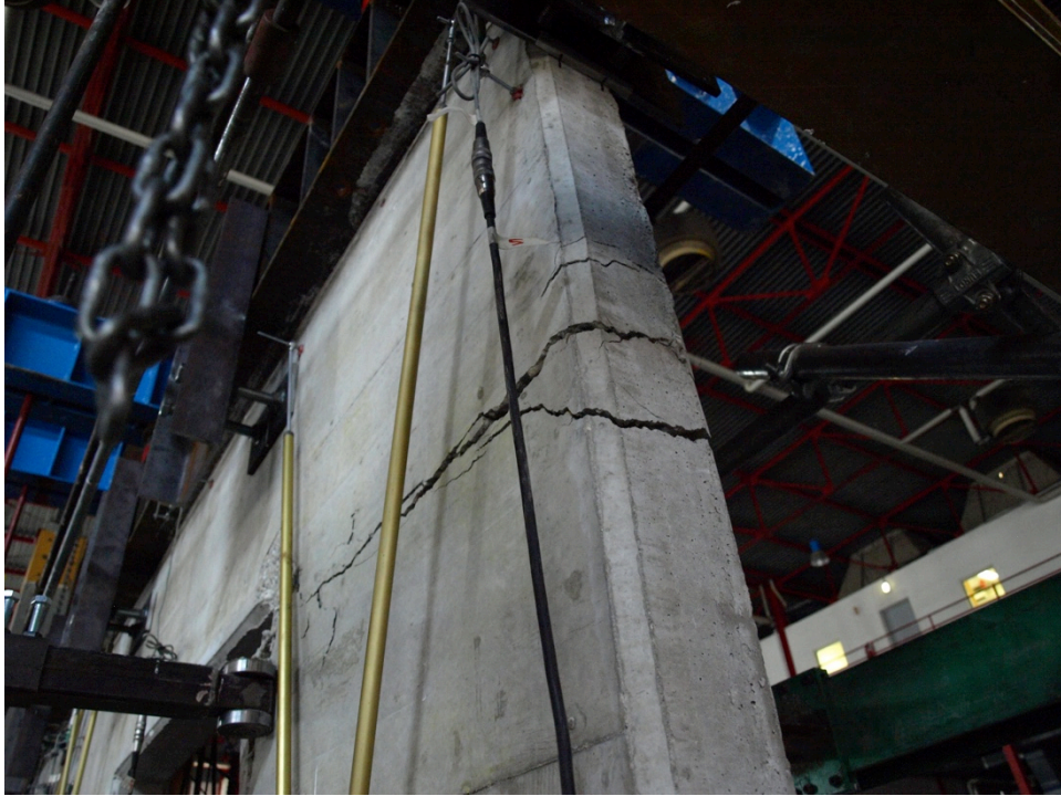
Figure 204: Side view of the horizontal crack at the top of the door – Specimen 07
