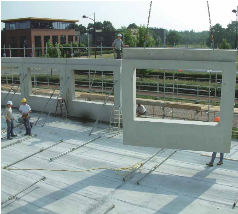
Fig.64: CRH Structural wall panels with openings
