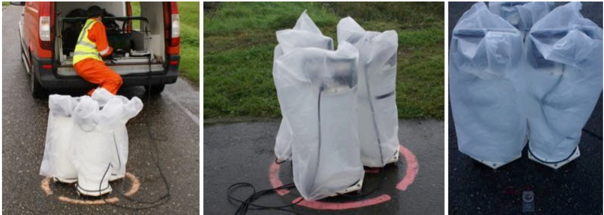
Figure 53: Pictures of plastic covers used for protecting the top electronics against heavy rainfall.
