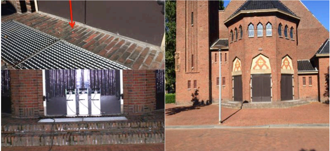
Figure 8: Photos from station 8.
