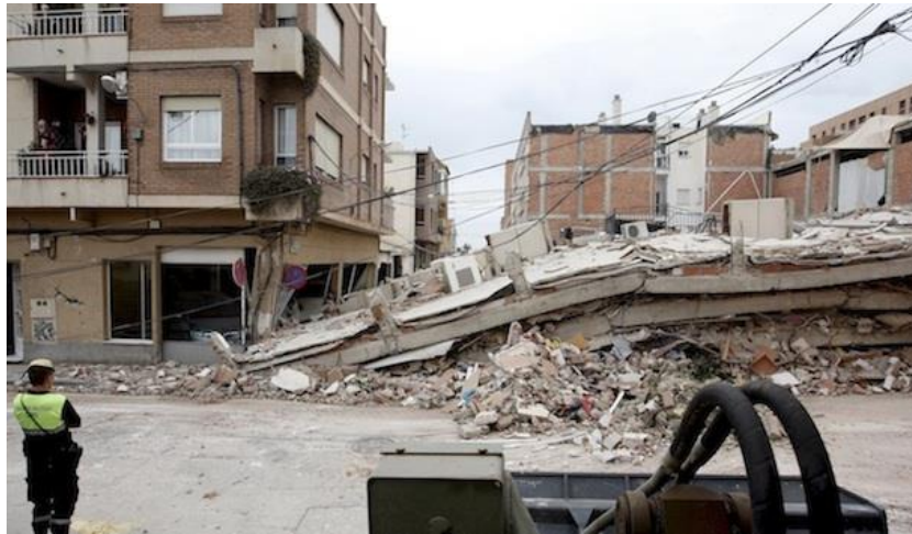
Figure A2.3.34. Building located in La Viña neighbourhood which collapsed during the main shock (Meteoweb, 2016). A street runs in between the two buildings shown.
