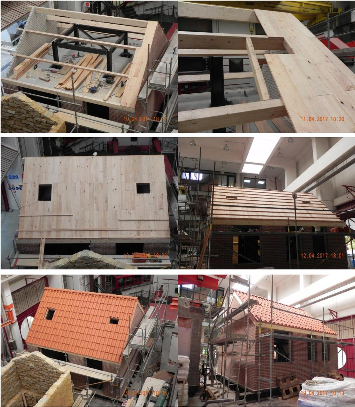
Figure 1.11 Construction of the roof and views of specimen after the laying of the tiles.
