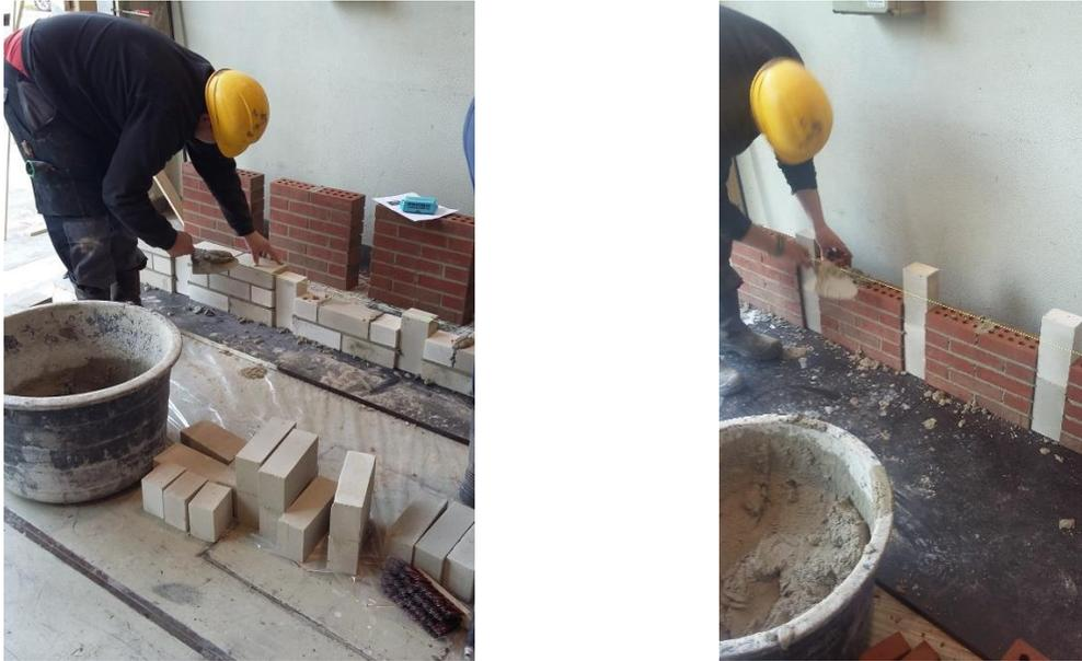
Figure 2.3 Construction of characterisation specimens at the time of mortar sampling.
