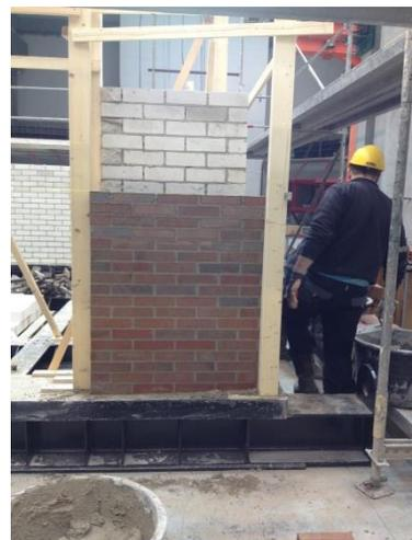
Figure 2.2 Construction of the full scale model at the time of collection of mortar samples.
