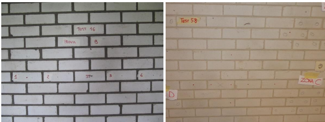
Figure 20. Example of Good Quality masonry for the Calcium Silicate < 1985 typology.
