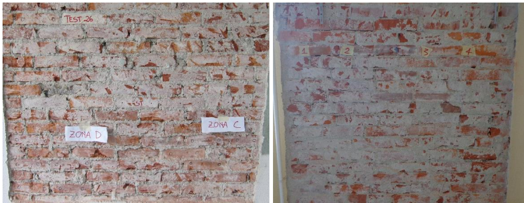
Figure 33. Example of Older Poor Quality masonry for the Clay > 1945 typology.
