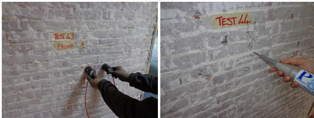
Figure 35. Example of Older Good Quality masonry for the Clay > 1945 typology.
