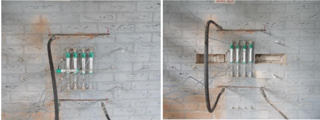
Figure 7. Double Flat Jack Test: “standard configuration” (left) and “Shove Test configuration” (right).
