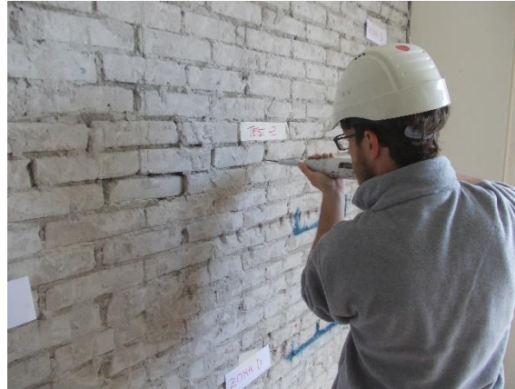
Figure 2. Penetrometric Test on Mortar.
