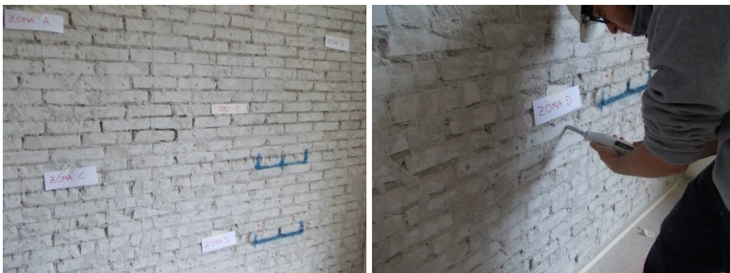
Figure 1. Rebound Hammer Test: identification of the 4 zones (left) and performance of the test (right).
