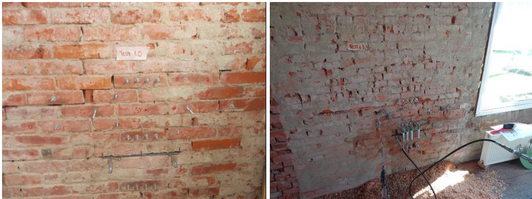
Figure 27. Example of Poor Quality masonry for the Clay < 1945 typology.
