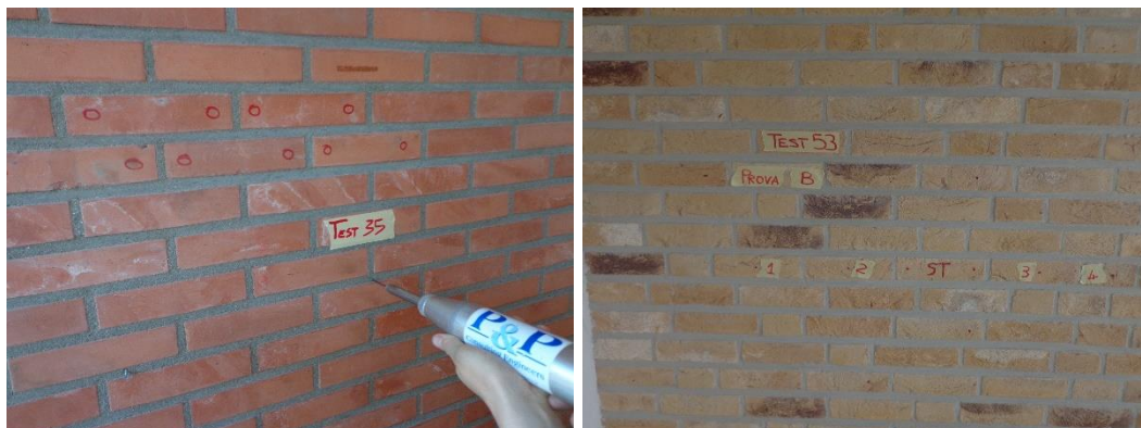
Figure 32. Example of Newer Units masonry for the Clay &gt; 1945 typology.
