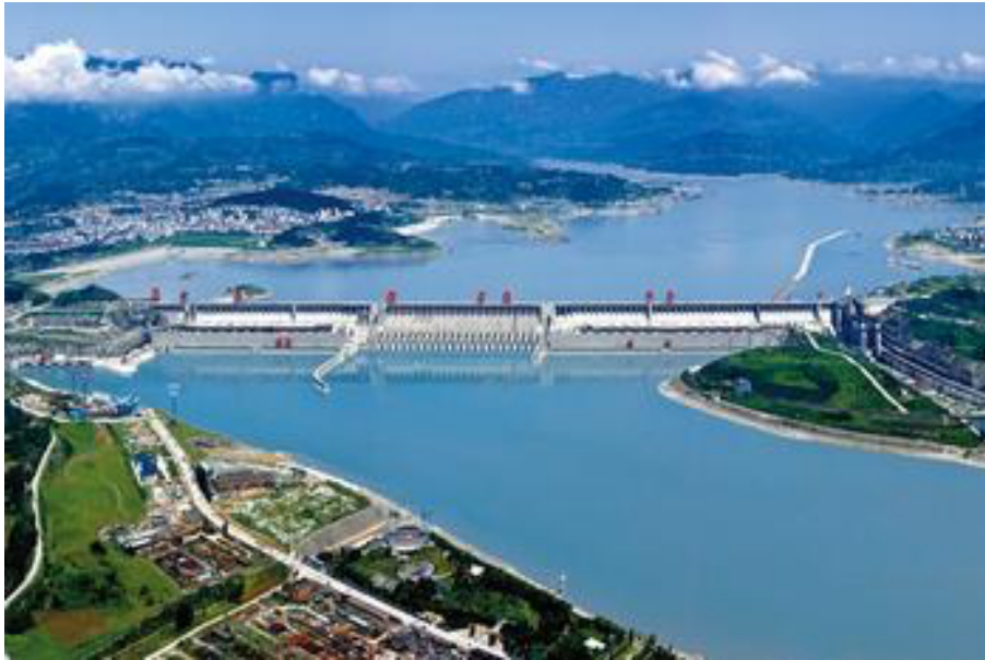
Figure 17: Aerial photograph of the Three Gorges dam, China 15 .
