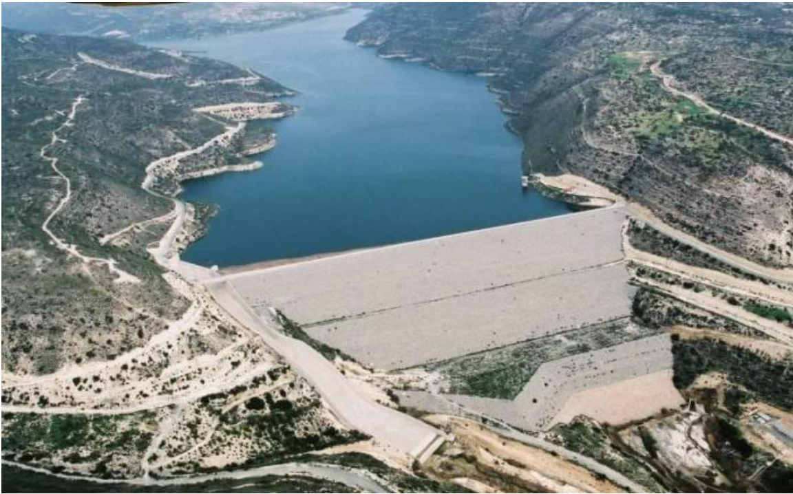
Figure 5: Aerial photograph of Nurek dam, Tadjikistan 14 .
