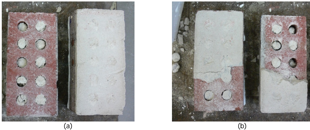
Figure 46 – Crack pattern of clay masonry specimen under shear test: (a) front-left joint; (b) front-right joint.
