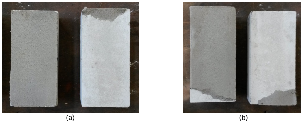
Figure 44 – Crack pattern of calcium silicate masonry specimen under shear test: (a) front-left joint; (b) front-right joint.
