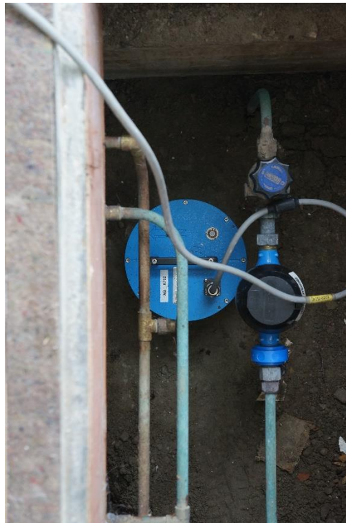
Figure 42. Geophone #10, underground on compacted soil, configuration 1, 2, 3
