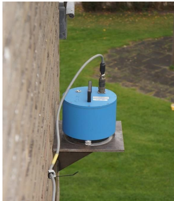
Figure 76. Detail of the positioning of geophone # 9.
