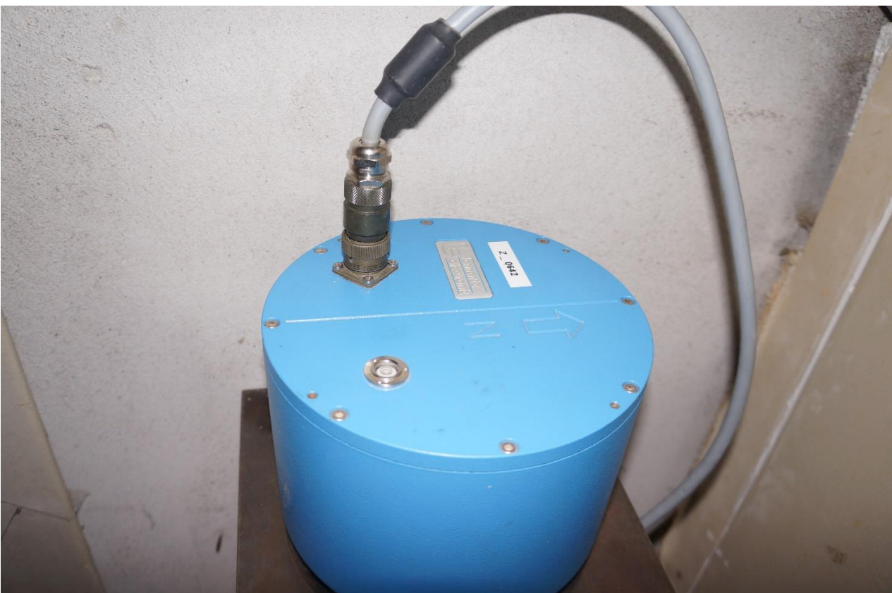
Figure 49. Geophone #7, 2 nd floor, configuration 1,2,3
