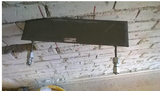
Figure 9. Single Flat Jack Test: the flat jack is inserted in the slot.
