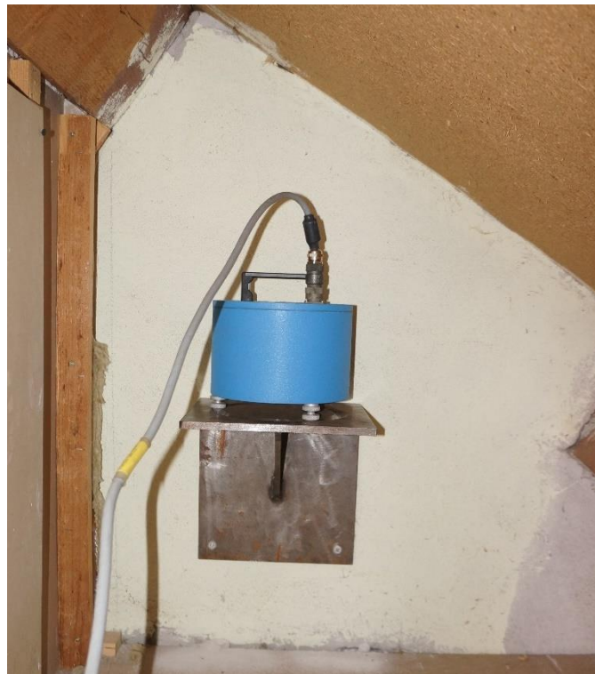
Figure 51. Geophone #9, 2 nd floor, configuration 1
