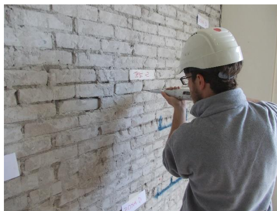
Figure 2. Penetrometric Test on Mortar.
