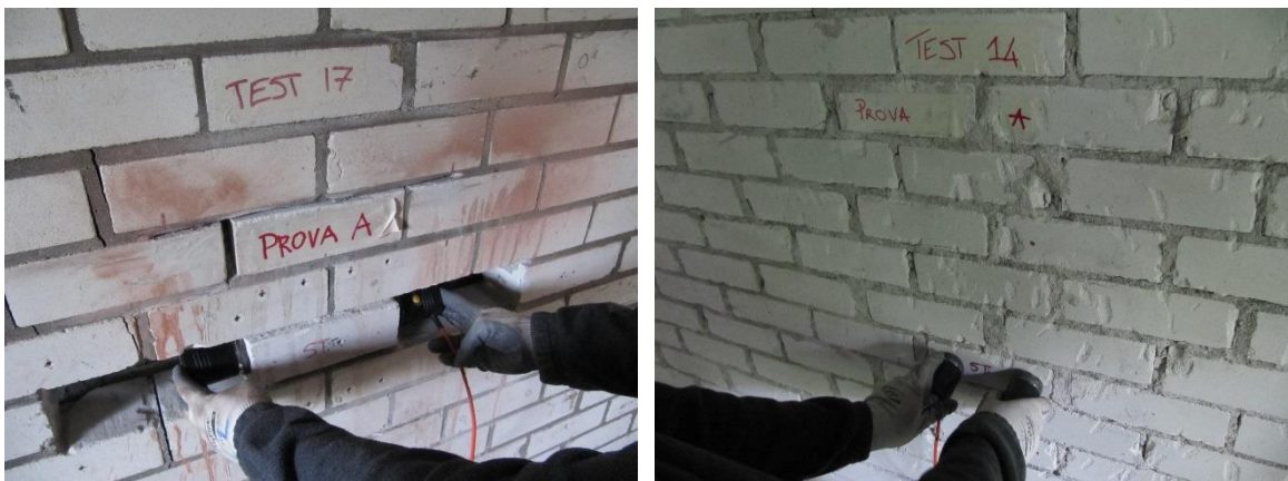
Figure 4. Ultrasonic Test: direct single unit configuration (left) and indirect single unit configuration (right).
