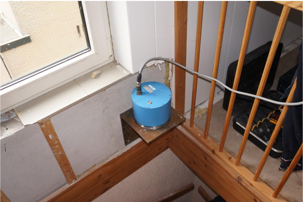
Figure 56. Geophone #8, 2 nd floor, configuration 2, 3
