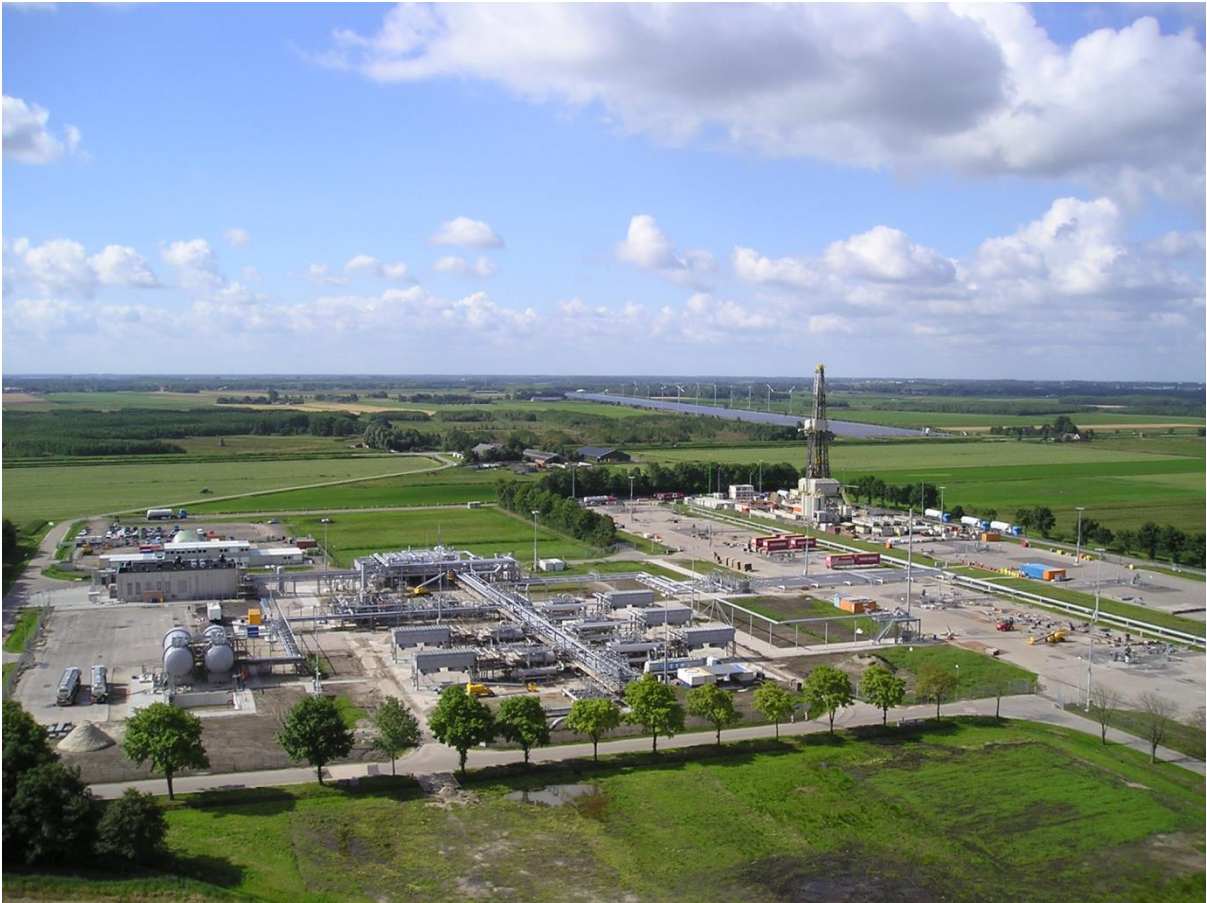
Eemskanaal Cluster with rig drilling Eemskanaal-13
