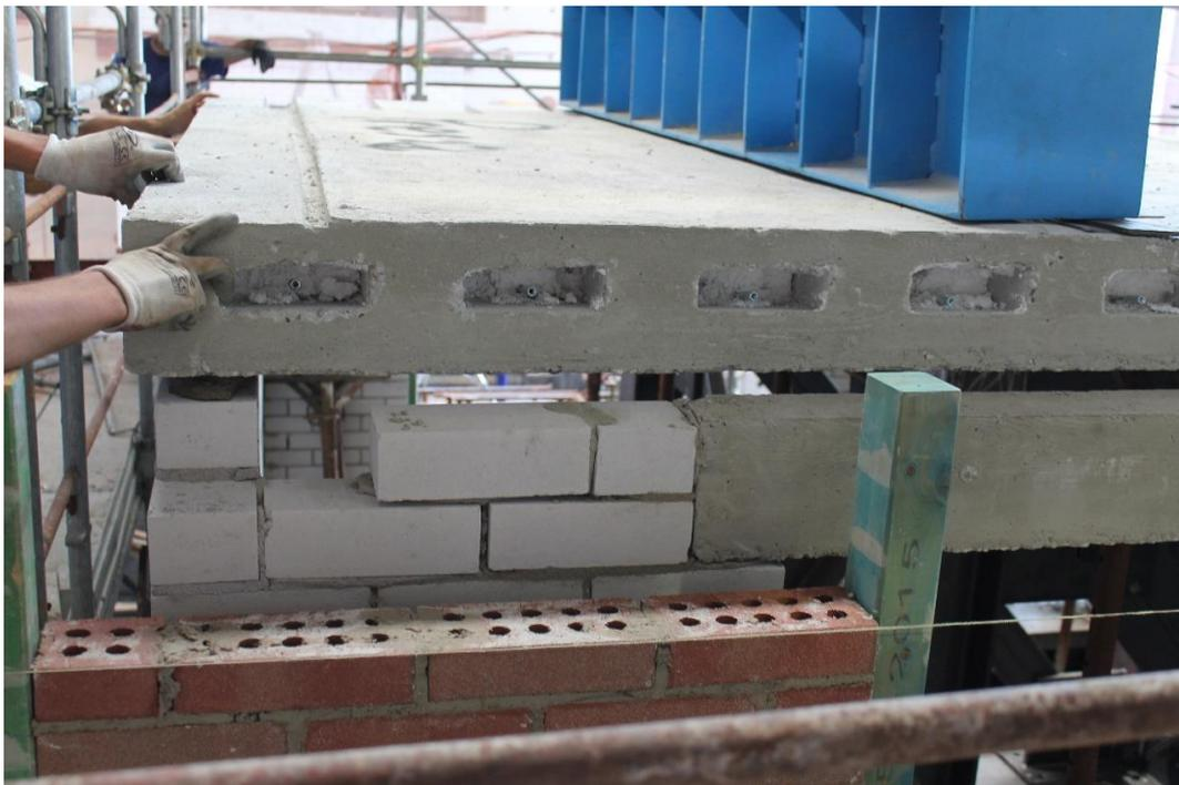
Figure 283. Positioning of the R.C. slab of the first floor - East side
