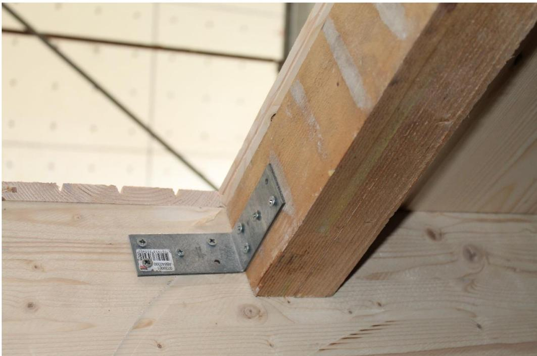
*Figure 295. Detail of the connection between the timber beam of the opening and the girder.*
