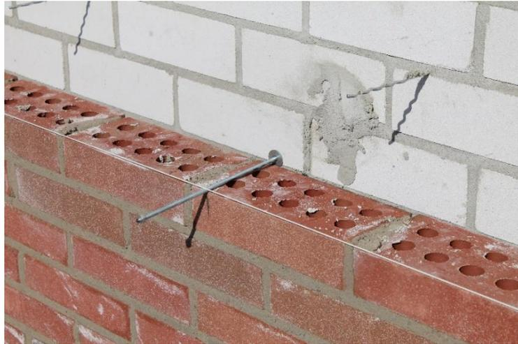
*Figure 167. Detail of tie installed for the specimen transportation.*
