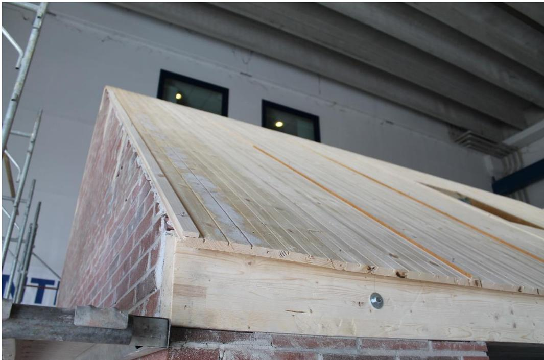
*Figure 297. Detail of the connection between the girder and the clay gable – 2.*
