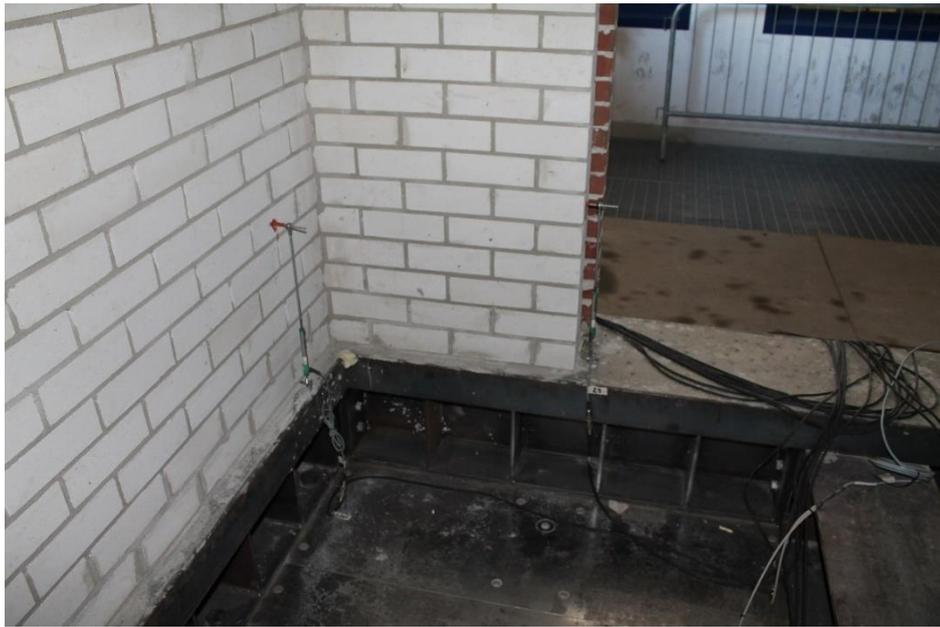
The Following pictures show the wire potentiometers #4 and #7 (passing through the CS walls) .
