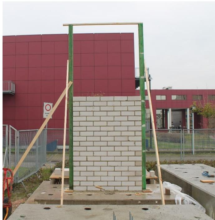
Figure 102. Slender wall during the construction phases.
