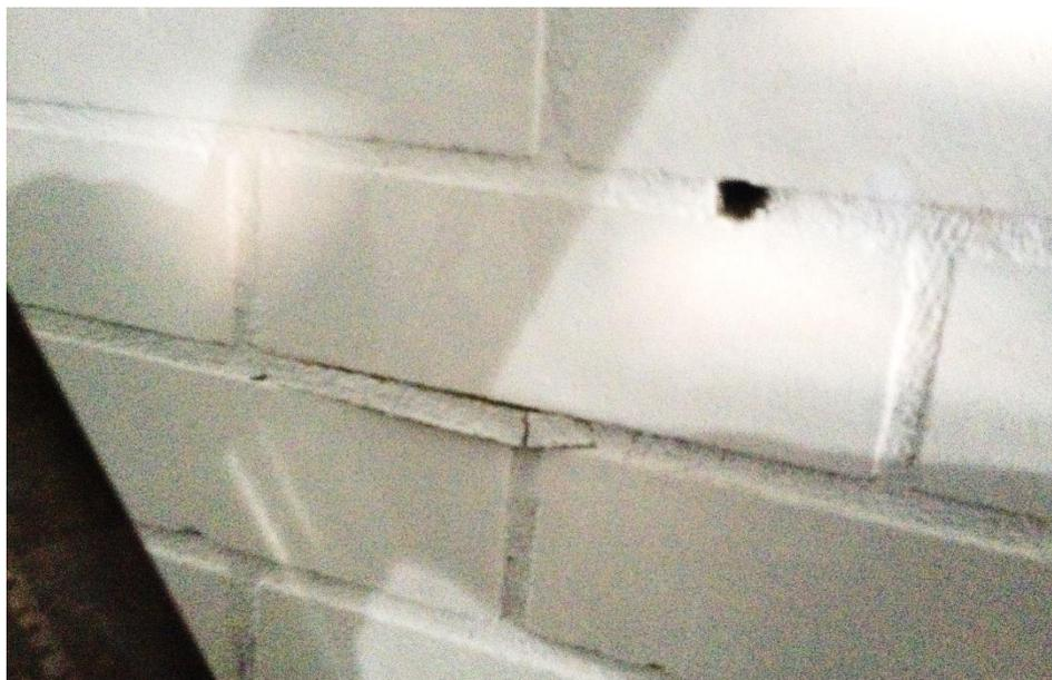
*Figure 250. Damage of the mortar bed joint.*
