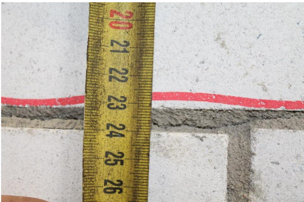
*Figure 198. Decrease in Mortar Bed-joint thickness..*
