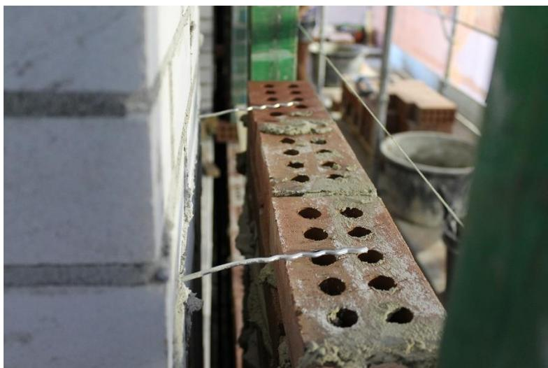
*Figure 279. Laying of the ties.*
