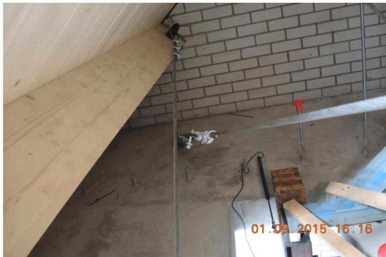
*Figure 299. Detail of two of the rods connecting the second floor to the roof beams.*
