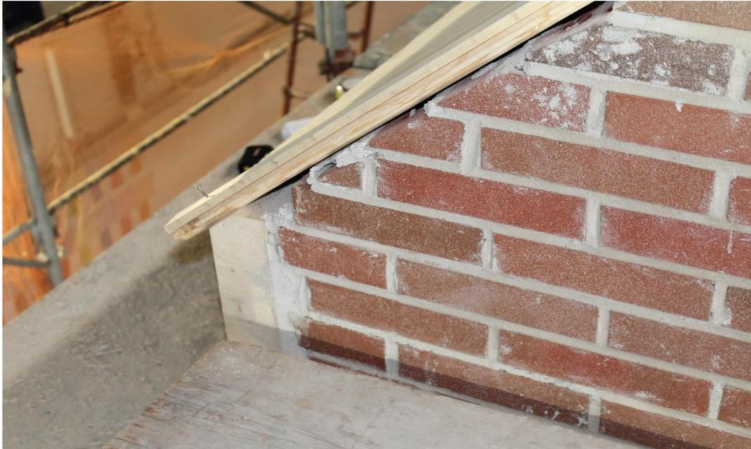
*Figure 296. Detail of the connection between the girder and the clay gable – 1.*
