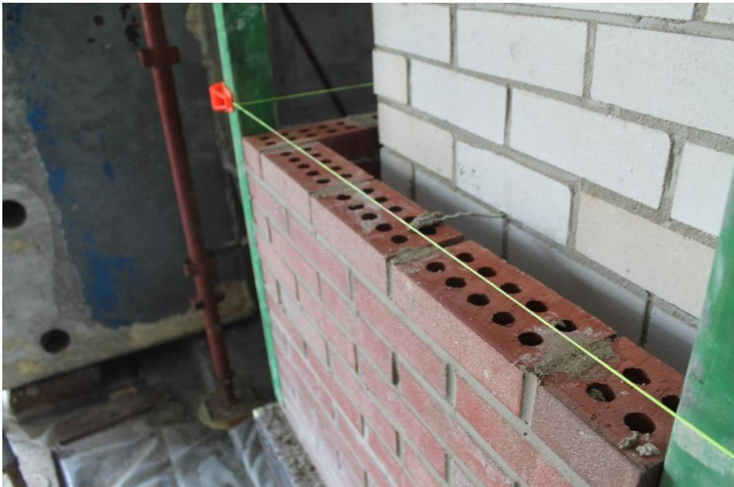
*Figure 268. Cavity wall.*
