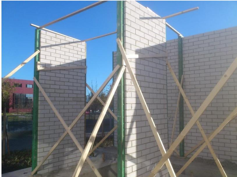
*Figure 104. Specimens for In-Plane tests during the construction phases.*
