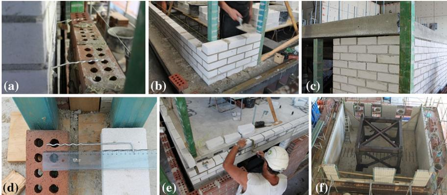
**Fig. 5** Construction details of the specimen: **a** positioning of cavity steel ties; **b** building phase of inner CS leaf; **c** laying of the second floor slab; **d** geometry of steel tie; **e** construction of CS leaves at second floor level; **f** safety steel frame
