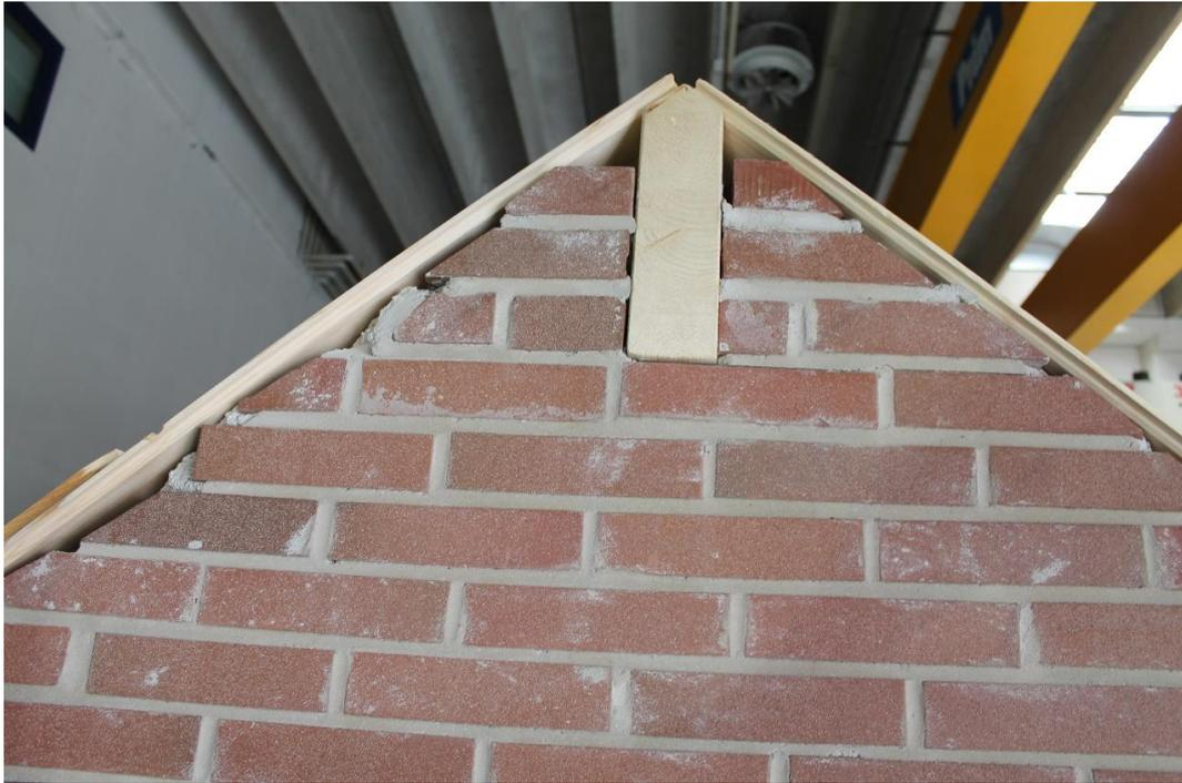
*Figure 298. Detail of the connection between the girder and the clay gable – 3.*
