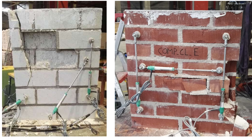
Figure 2:17: Failure of CS (left) and clay (right) walette under compression perpendicular to bed joints..
