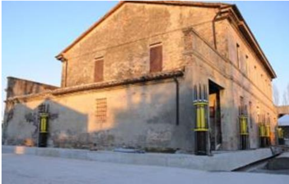
Figure 10.9 Example of an Italian masonry building jacked-up for introduction of isolators
