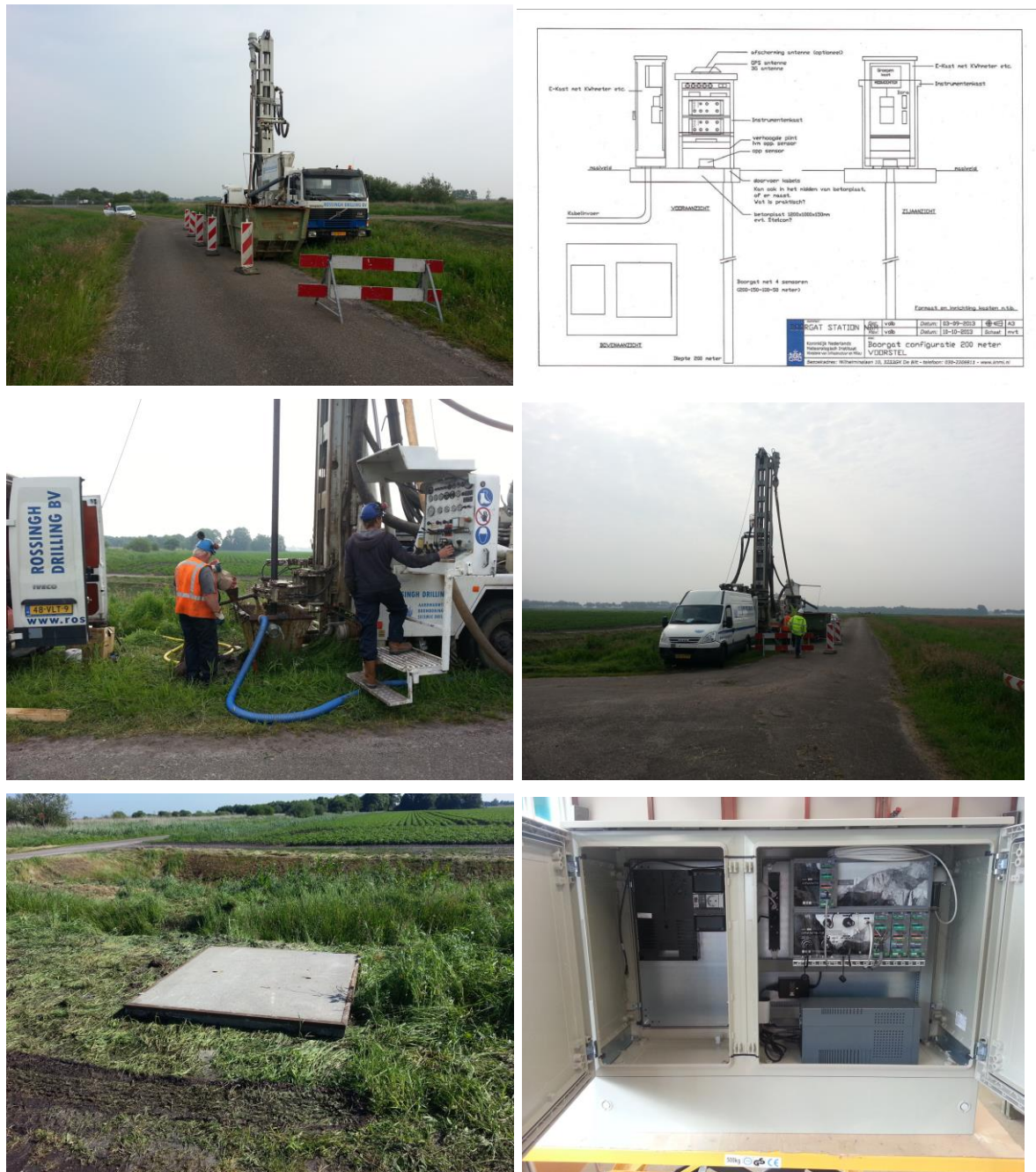
Figure 3.7 Extension of the shallow borehole geophone network.
